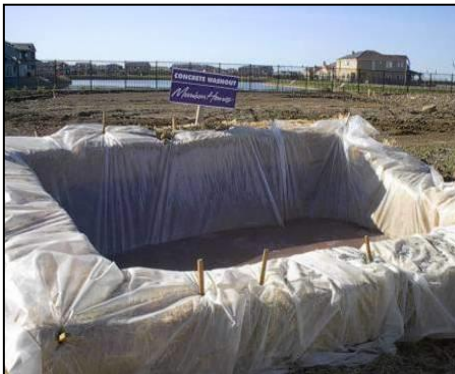
Plate 3-1 Typical concrete wash out areas
