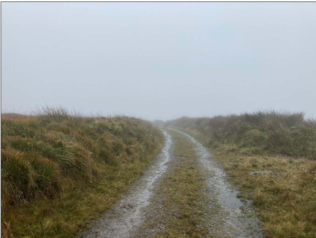
Photo 4: Existing track along section of 110kV underground cabling route
