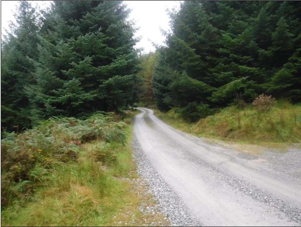
Photo 1: Existing access track on TDR
