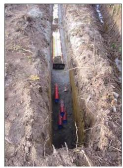
Plate 4-5 Typical Cable Trench View
