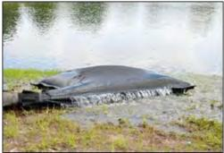
Plate 4-4 Silt bag under inspection
