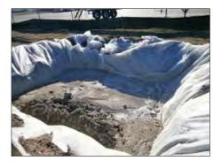
Plate 4-1 Concrete washout area
