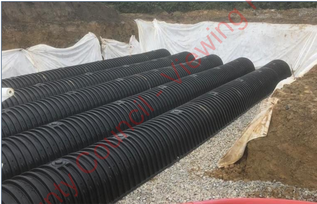
Figure 4-9 Typical Poly Tunnel Installation Arrangement
