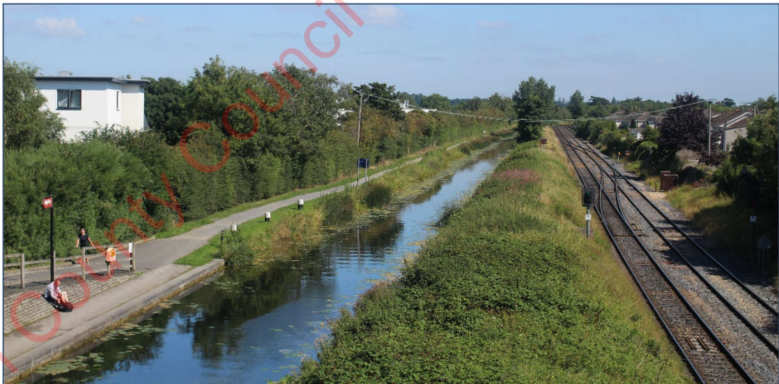
Plate 11-31 View to the east along the Royal Canal corridor from Mullen Bridge in Maynooth Town
