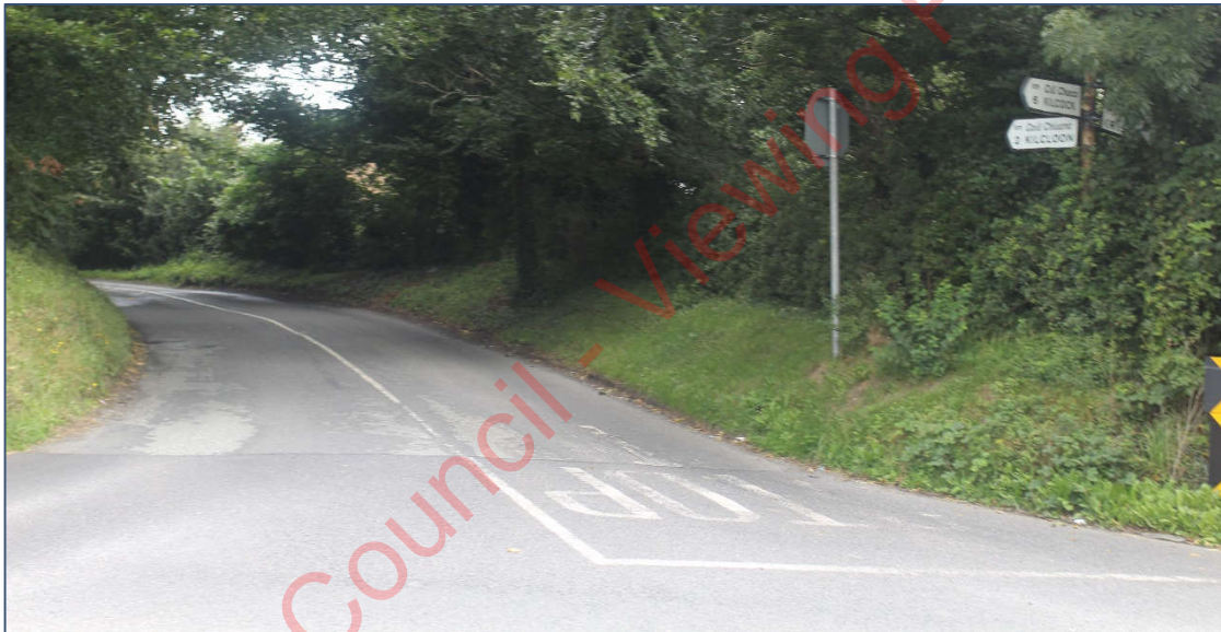
Plate 11-12 Junction between the L6219, L2214-3 and L2214. At the centre of the Proposed Development site.
