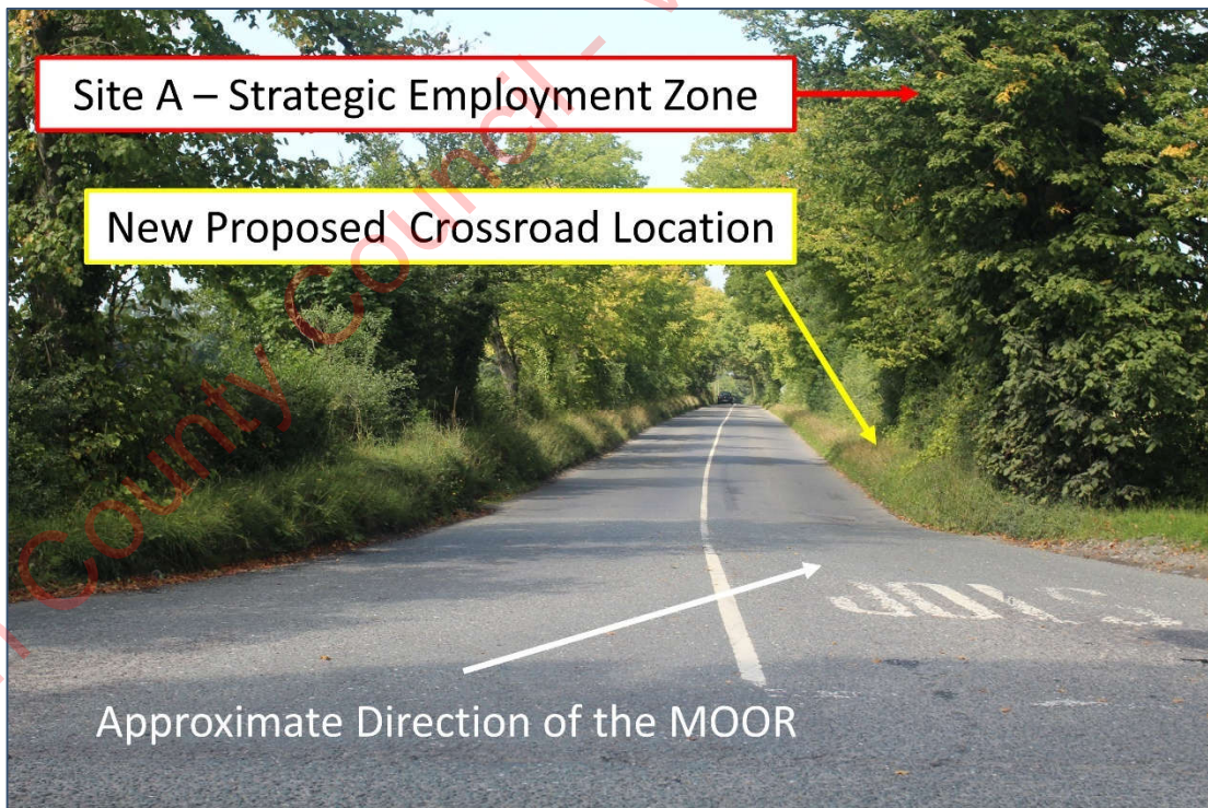
Plate 11-14 View west-north-west along the L2214-3 Local Road from the existing junction with the R157.
