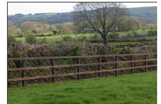
Timber Post and Rail Fence 1.4m high
