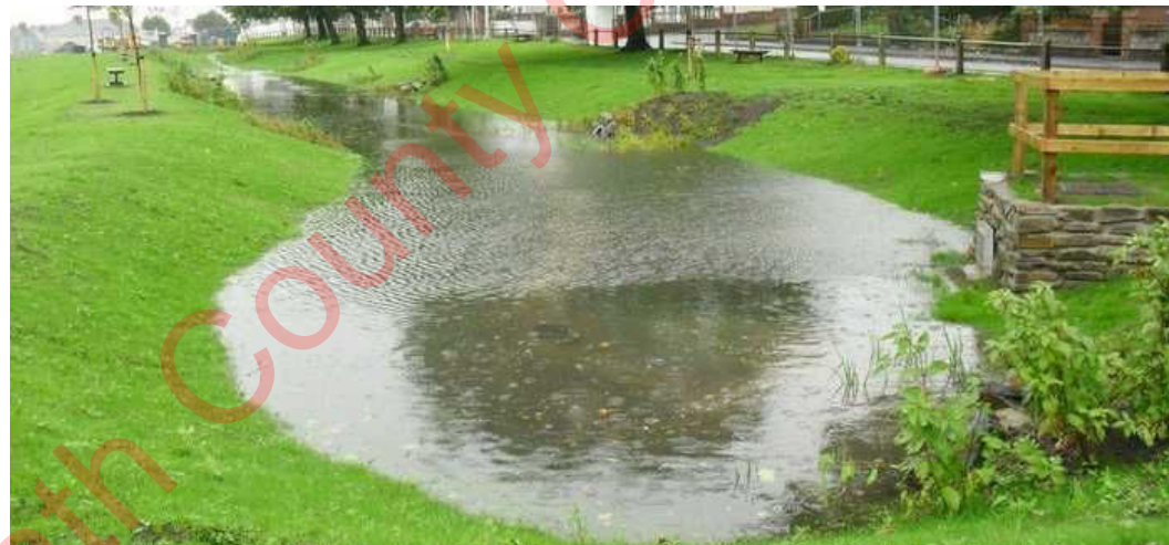
Typical swale in wet weather
