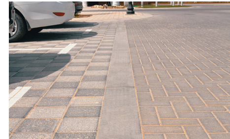
Flush Slipform Concrete Kerb
