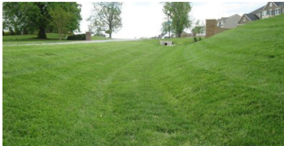
Typical swale in dry weather
