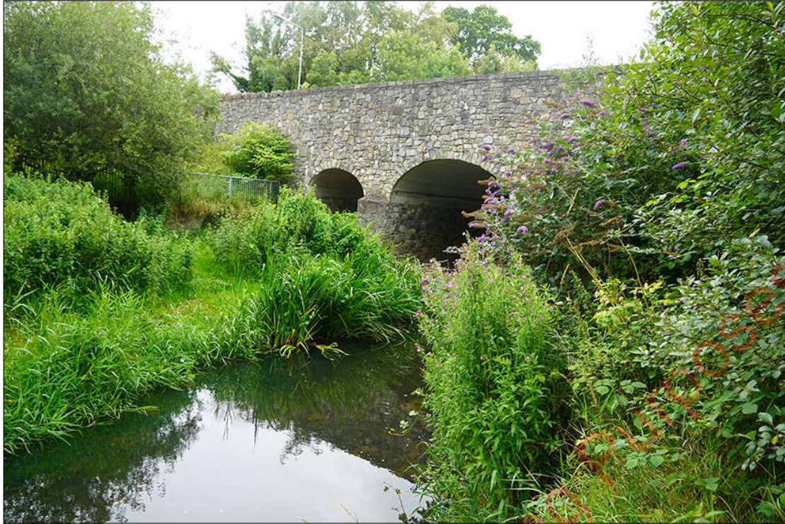
Plate 12-9 Kildare bridge, from SE.
