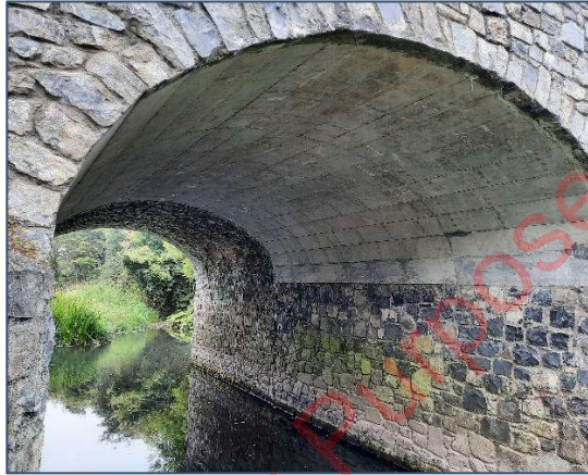
Plate 4-7 Interior bridge view
