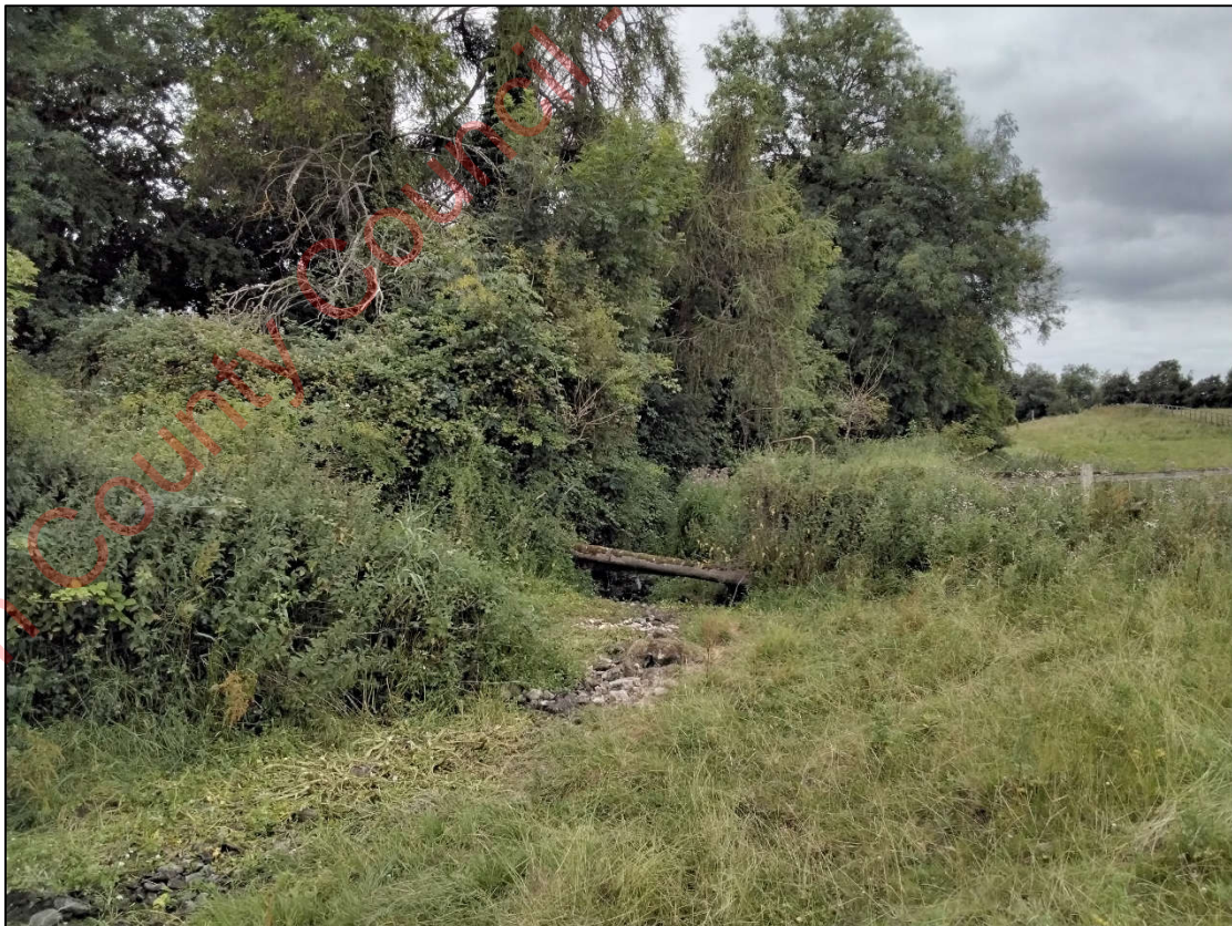
Plate 6-15. Blackhall Little River with no flowing water located to the north of the MOOR route
