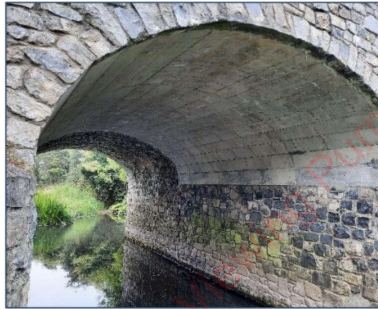
Plate 4-7 Interior bridge view
