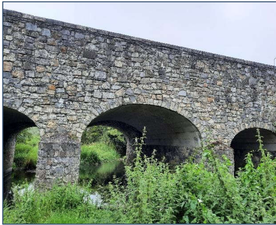
Plate 4-6 Exterior bridge view
