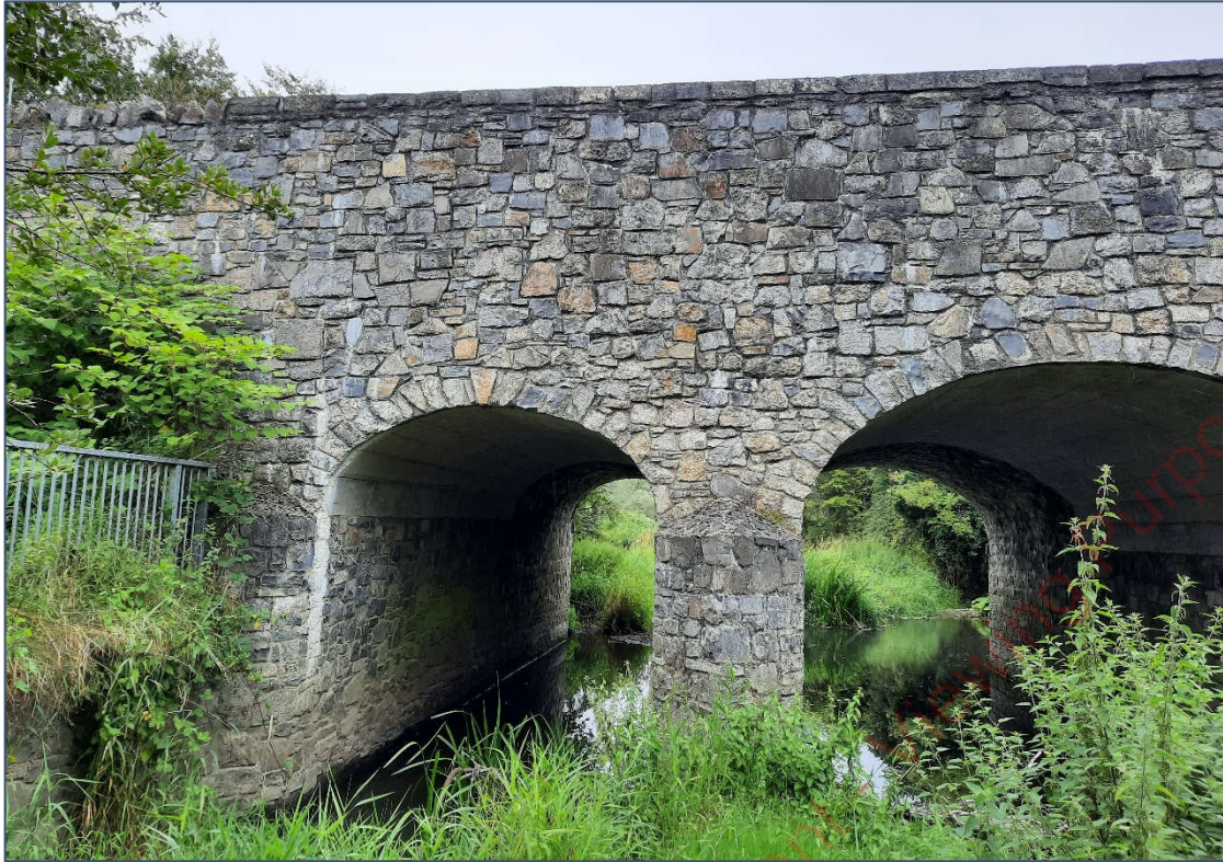
Plate 11-26 Kildare Bridge viewed from the West.
