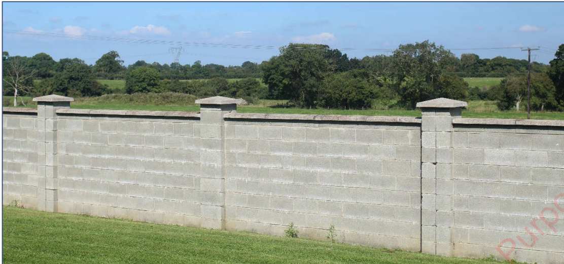
Plate 11-49 View north towards the Site C from within the Moyglare Hall Residential Housing Estate.
