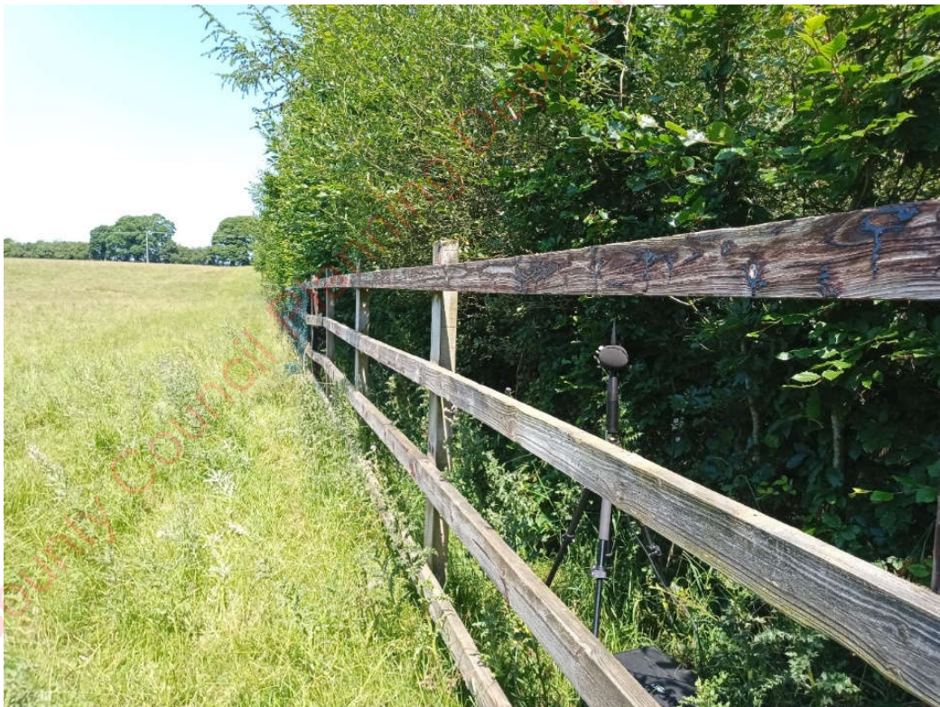
Plate 10-5 N5, looking north.
