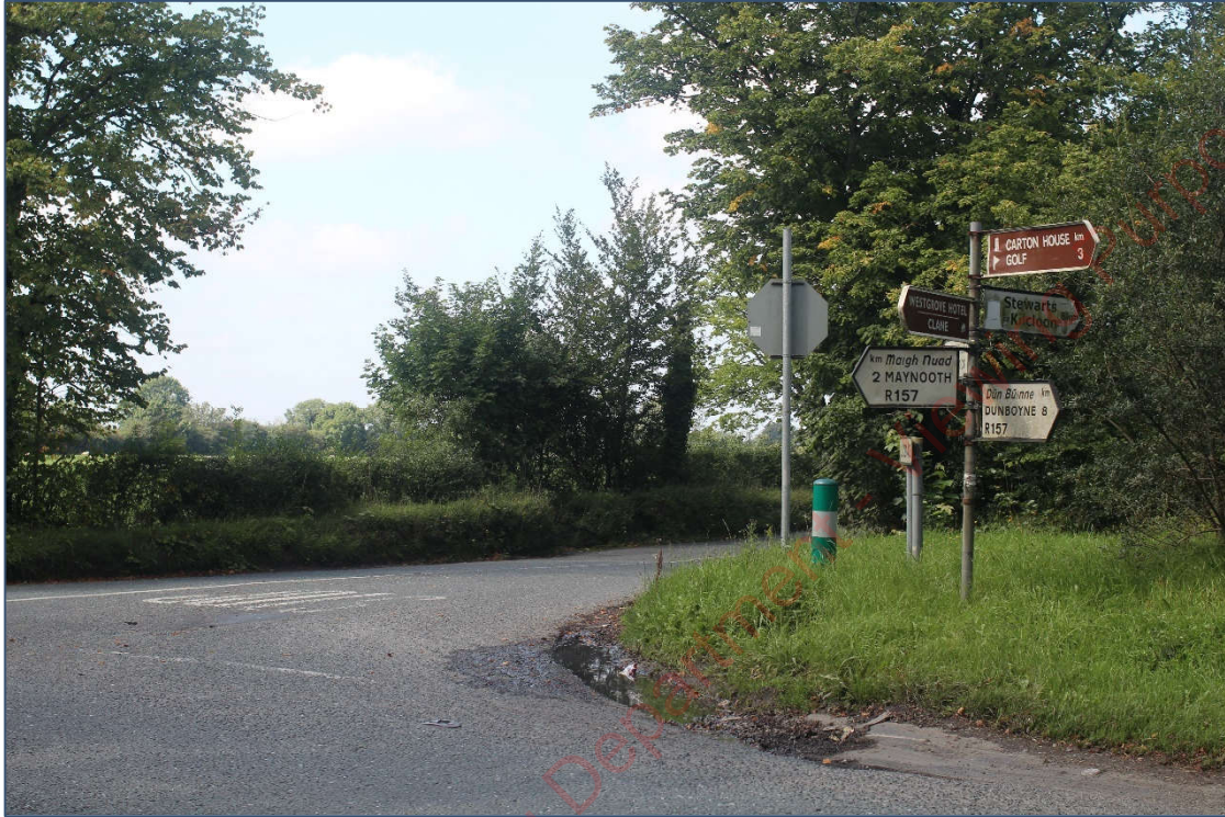
Plate 11-61 Junction between the R157 and the L2214-3 Local Road at Moygaddy
