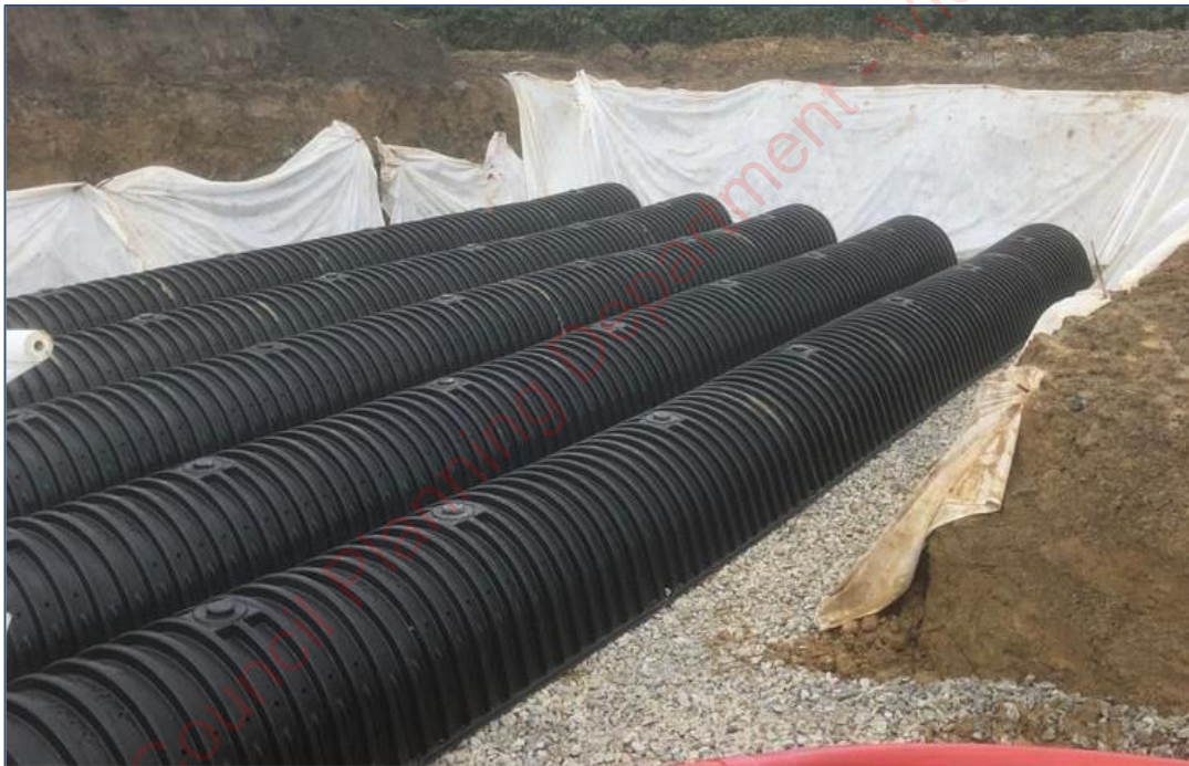
Figure 4-9 Typical Poly Tunnel Installation Arrangement
