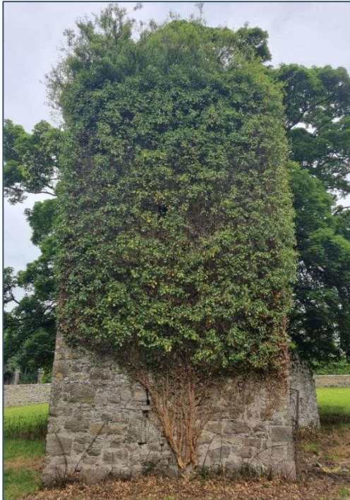
Plate 4-3 South facing wall of the castle tower with dense ivy cover
