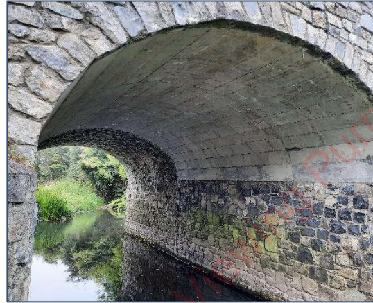
Plate 4-7 Interior bridge view
