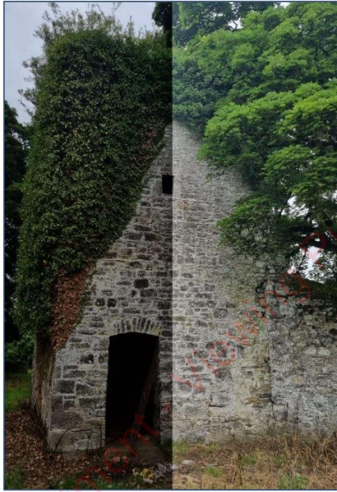
Plate 4-4 East facing wall of the castle tower with potential access through door and window
