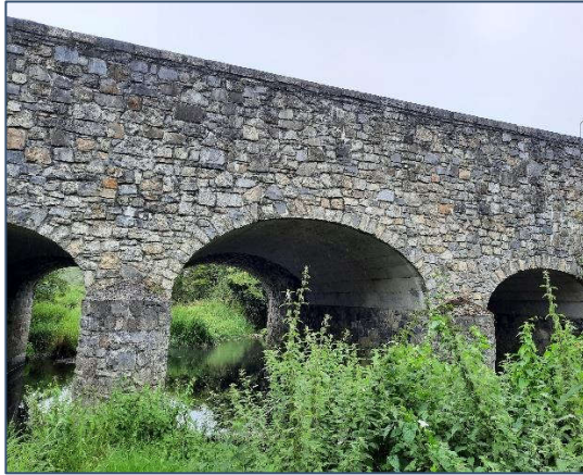
Plate 4-6 Exterior bridge view
