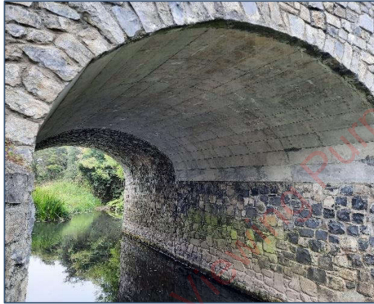
Plate 4-7 Interior bridge view
