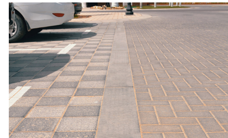
Flush Slipform Concrete Kerb
