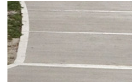
Brushed Concrete with trowel edge finish (streets)
