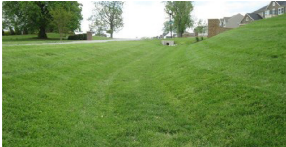
Typical swale in dry weather
