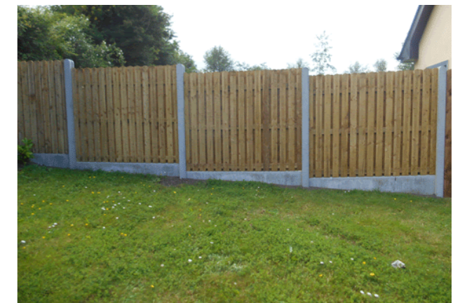
Concrete Post & Wooden Panel Fence █
