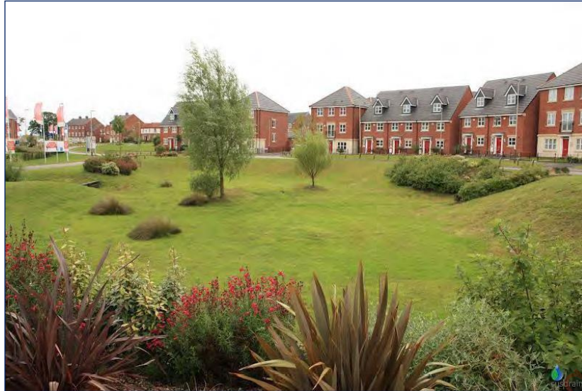
Figure 3.15 - Example Detention Basin
