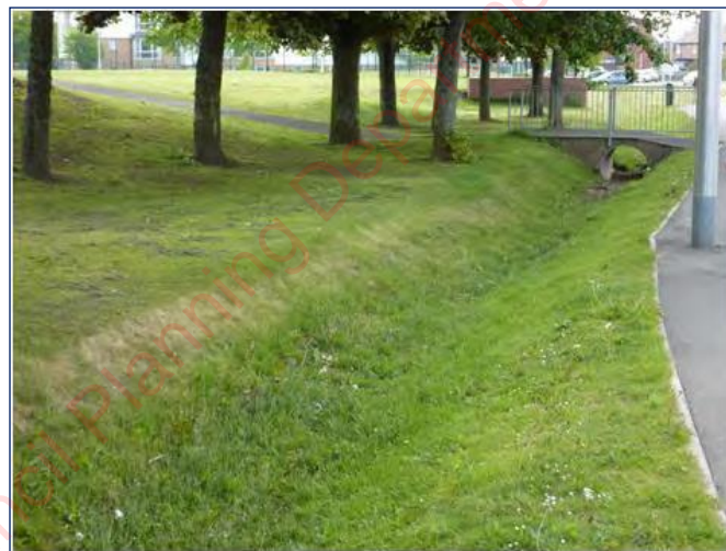
Figure 3.9 – Example Roadside Swale
