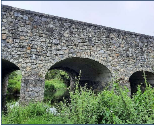
Plate 4-6 Exterior bridge view
