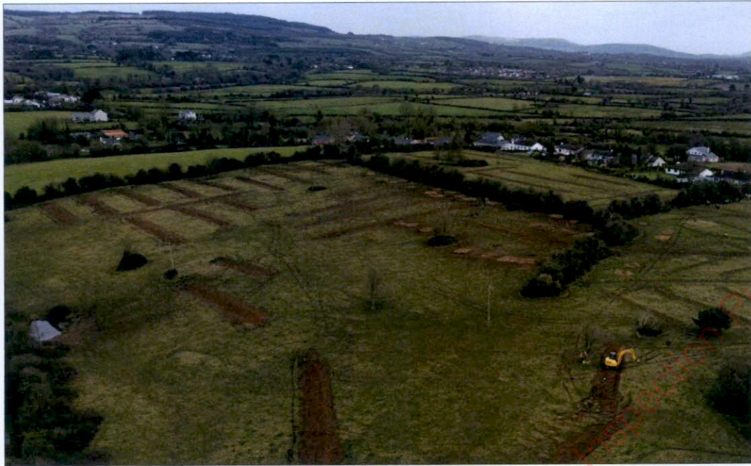
Plate 15.13 Aerial image of closed trenches in the Phase 3 area, facing northeast
