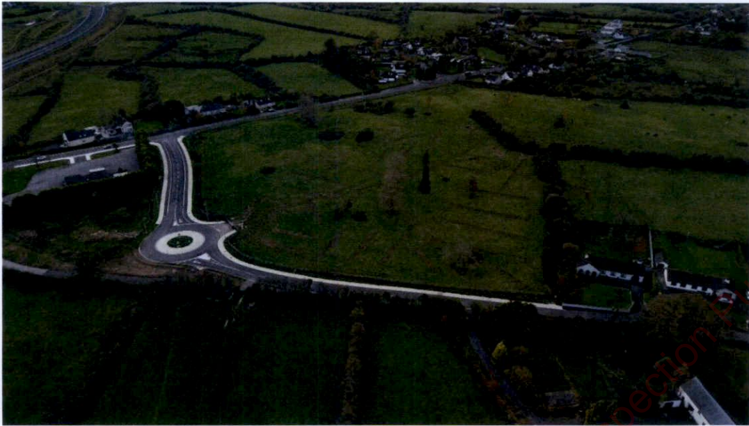
Plate 15.7 Drone view of Clonconane, facing southwest
