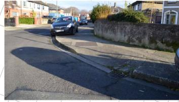
UNCONTROLLED CROSSING POINT WITH NO DISHED KERB AND TACTILE PAVING PROVIDED. A DISHED KERB AND BUFF\* OR GREY TACTILE PAVING SHOULD BE CONSIDERED (FOR AN IN LINE CROSSING). DEPTH OF 1.2 M. GRADIENT 1:12 MAX. LEVEL DIFFERENCE OF DISHED KERB: 6MM.
