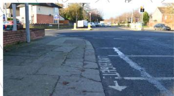
CONTROLLED CROSSING POINT WITH NO TACTILE PAVING AND PROPER KERB
