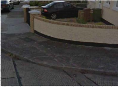
UNCONTROLLED CROSSING WITH A HIGH UPSTAND. LEVEL DIFFERENCE SHOULD BE HIGHER THAN 6MM IN THE DISHED KERB WITH THE CARRIAGEWAY. ABSENCE OF TACTILE PAVING
