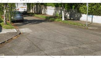
UNCONTROLLED CROSSING POINT WITH NO KERB DISPOSED. A DISHED KERB AND BUFF\* OR GREY TACTILE PAVING SHOULD BE CONSIDERED (FOR AN IN LINE CROSSING). DEPTH OF 1.2 M, GRADIENT 1:12 MAX. LEVEL DIFFERENCE OF DISHED KERB: 6MM.
