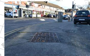
DETERIORATING PAVING AROUND AN IRON GRID COVER IN THE DIRECT LINE OF THE FOOTPATH. PAVEMENT CRACKED SHOULD BE REPAIRED TO BE FIRM AND HARD-
