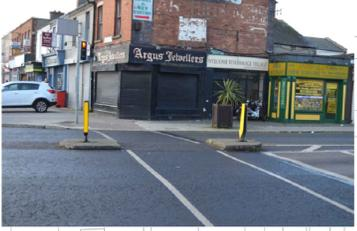
IF THE CENTRAL ISLAND IS INTENDED TO BE AN AREA TO WAIT, THEN TACTILE PAVING SHOULD BE PROVIDED.
