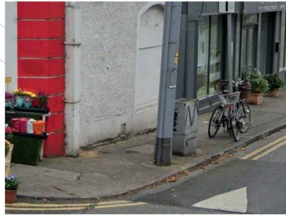
REDUCED WIDTH OF THE FOOTPATH DUE TO THE POSITION OF THE LIGHTING COLUMN AND THE ELECTRICITY BOX. A MINIMUM DISTANCE OF 1200MM IN A LENGTH OF 2000MM SHOULD BE ENSURED.
