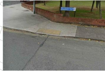
A CONTROLLED CROSSING IS PROPOSED IN THE DESIGN PROJECT IN THE CURRENT UNCONTROLLED CROSSING. ACCESSIBILITY MEASURES FOR THIS TYPE OF CROSSING SHOULD BE CONSIDERED. RED BLISTER TACTILE PAVING WITH A L-SHAPED STEM FOR ORIENTATING PEOPLE WITH VISION IMPAIRMENT.
