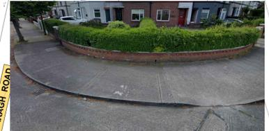
ACCESSIBILITY MEASURES IN UNCONTROLLED CROSSING SHOULD BE PROVIDED. DISHED KERBS AND TACTILE PAVING SURFACE. SOME FOOTPATH IN THIS PART OF THE ROUTE WERE CONSTRUCTED WITH NO BOUNDARY KERB. THIS USE TO BE A HAZARD FOR PEDESTRIANS AND DISABLE PEOPLE WITH A NO CORRECT PROTECTION FROM THE CARRIAGEWAY. KERBS SHOULD BE INTEGRATED.
