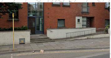
CHANGE IN LEVEL FOR ACCESSING BUILDING. REVIEW TACTILE PAVING IN STAIRS AND RAMPS. DOUBLE HANDRAILS.
