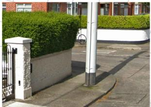
LIGHTING COLUMN IN THE MIDDLE OF THE FOOTPATH. 1500 MM. MINIMUM WIDTH OF THE FOOTPATH WHEN OBSTACLES CAN NOT BE REMOVED. 1200 MM. IN A DISTANCE OF 2000MM LENGTH IS ACCEPTED. LOCATION OF SOME URBAN POLES AND COLUMNS THAT CONSTRAINT THE FOOTPATH SHOULD BE RECONSIDERED.
