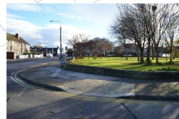
UNCONTROLLED CROSSING POINT WITH NO DISHED KERB AND TACTILE PAVING PROVIDED. A DISHED KERB AND "BUFF" OR GREY TACTILE PAVING SHOULD BE CONSIDERED (FOR AN IN LINE CROSSING). DEPTH OF 1.2 M, GRADIENT 1:12 MAX. LEVEL DIFFERENCE OF DISHED KERB: 6MM
