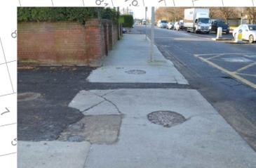
DIFFERENT SURFACE MATERIALS IN THE LINE OF THE FOOTPATH. PAVEMENT SHOULD BE REPAIRED.
