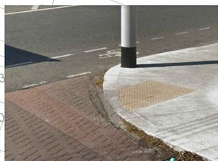
THE ENCOUNTER BETWEEN THE FOOTPATH AND THE ROAD COULD BE IMPROVED. THE VERTICAL DEVIATION AND THE STEEP GRADIENT IN THE EDGE CAN BE A HAZARD FOR PEOPLE WITH MOBILITY IMPAIRMENT.
