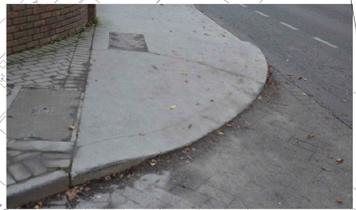
UNCONTROLLED CROSSING POINT WITH NO KERB DISPOSED. A DISHED KERB AND BUFF" OR GREY TACTILE PAVING SHOULD BE CONSIDERED (FOR AN IN LINE CROSSING). DEPTH OF 1.2 M, GRADIENT 1:12 MAX. LEVEL DIFFERENCE OF DISHED KERB: 6MM. THE CRACKED PAVING IN THE CARRIAGEWAY OF THE SIDE ROAD SHOULD BE REPAIRED. IT SHOULD BE LOCATED NOT IN THE CURVE OF THE FOOTPATH.
