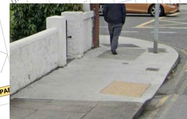
A L-SHAPEP STEM EXTENDED TO THE BUILDING LINE SHOULD BE RECOMMENDED IN A NOT IN LINE UNCONTROLLED CROSSING.
