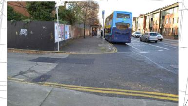
UNCONTROLLED CROSSING POINT WITH NO KERB DISPOSED. A DISHED KERB AND BUFF\* OR GREY TACTILE PAVING SHOULD BE CONSIDERED (FOR AN IN LINE CROSSING). DEPTH OF 1.2 M. GRADIENT 1:12 MAX. LEVEL DIFFERENCE OF DISHED KERB: 6MM. THE CRACKED PAVING IN THE CARRIAGEWAY OF THE SIDE ROAD SHOULD BE REPAIRED
