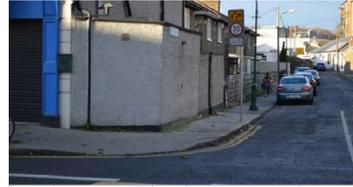
UNCONTROLLED CROSSING WITH NO TACTILE PAVING AND DISHED KERB. ACCESSIBILITY MEASURES FOR THIS TYPE OF CROSSING SHOULD BE PROVIDED. A DISHED KERB AND BUFF\* OR GREY TACTILE PAVING SHOULD BE CONSIDERED (FOR AN IN LINE CROSSING). DEPTH OF 1.2 M. GRADIENT 1:12 MAX.
