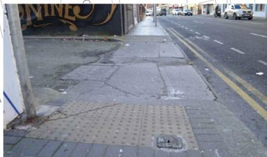
UNCONTROLLED CROSSING POINT AT A SIDE ROAD. CRACKED PAVING IN THE CARRIAGEWAY FOR CROSSING. THE PAVEMENT SHOULD BE REPAIRED AT THIS POINT WITH MINIMAL VERTICAL DEVIATIONS.
