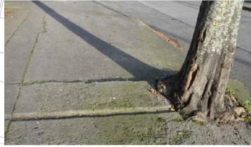
UNEVEN PAVING IN CONCRETE FOOTPATH BY THE ROOTS OF THE TREES. VERTICAL DEVIATIONS OF MORE OF 5MM. SHOULD BE AVOIDED. CONCRETE PAVING SURFACE AROUND THE TREE SHOULD BE REPAIRED.
