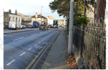
REDUCED WIDTH IN THE FOOTPATH ADJACENT TO HAROLD CROSS PARK. A MINIMUM WIDTH OF THE FOOTPATH OF 1500MM SHOULD BE ENSURED AND 1200MM IN SOME POINTS IN A LENGTH OF 2000MM.
