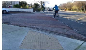
UNCONTROLLED CROSSING POINT AT SIDE ROAD. HIGH UPSTAND IN THE INTERSECTION WITH THE CARRIAGEWAY. LEVEL DIFFERENCE BETWEEN SURFACES SHOULD BE LESS THAN 6MM.
