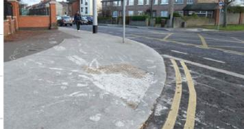
DETERIORATING PAVING AT UNCONTROLLED CROSSING POINT. TACTILE PAVING SHOULD BE REPAIRED AT THIS CROSSING IN-LINE. 1200MM DEEP (3 SLABS)
