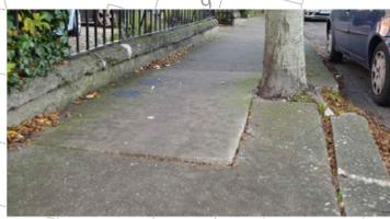
CONCRETE LIFTED IN THE FOOTPATH BY THE ROOT OF THE TREES. PAVEMENT SHOULD BE REPAIRED FOR AVOIDING VERTICAL DEVIATIONS.
