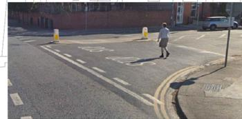
UNCONTROLLED CROSSING WITH NO TACTILE PAVING AND DISHED KERB. ACCESSIBILITY MEASURES FOR THIS TYPE OF CROSSING SHOULD BE PROVIDED. A DISHED KERB AND BUFF\* OR GREY TACTILE PAVING SHOULD BE CONSIDERED (FOR AN IN LINE CROSSING). DEPTH OF 1.2 M. GRADIENT 1:12 MAX. LEVEL DIFFERENCE OF DISHED KERB: 6MM IF THE CENTRAL ISLAND IS INTENDED AS AN AREA TO WAIT THEN TACTILE PAVING TO BE ALSO PROVIDED INSIDE. OPTIMUM TIME OF CROSSING SHOULD BE CHECKED.
