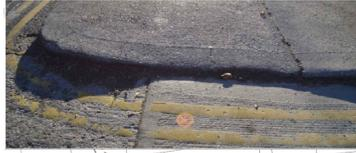
UNCONTROLLED CROSSING WITH A HIGH UPSTAND. LEVEL DIFFERENCE SHOULD BE HIGHER THAN 6MM IN THE DISHED KERB WITH THE CARRIAGEWAY. ABSENCE OF TACTILE PAVING
