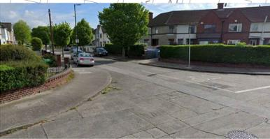
ABSENCE OF KERB AND TACTILE PAVING IN AN UNCONTROLLED CROSSING POINT. A DISHED KERB AND BUFF\* OR GREY TACTILE PAVING SHOULD BE CONSIDERED (FOR AN IN LINE CROSSING). DEPTH OF 1.2 M, GRADIENT 1:12 MAX. LEVEL DIFFERENCE OF DISHED KERB: 6MM.
