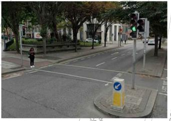
IF THE CENTRAL ISLAND IS INTENDED AS AN AREA TO WAIT THEN RED BLISTER TACTILE PAVING SHOULD BE PROVIDED AT THIS POINT. OPTIMUM TIME FOR CROSSING SHOULD BE CHECKED.
