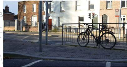
CONTROLLED CROSSING WITH A HIGH UPSTAND. THE LEVEL DIFFERENCE IN THE DISHED KERB SHOULD NOT BE HIGHER THAN 6MM. FOR AVOIDING HAZARD FOR WHEELCHAIR USERS AND PEOPLE WITH MOBILITY IMPAIRMENTS.
