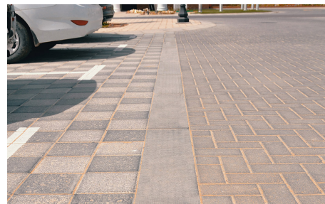
Flush Slipform Concrete Kerb
