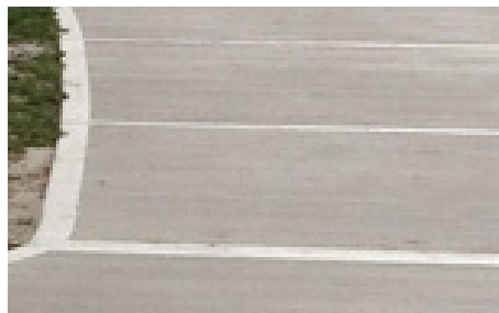
Brushed Concrete with trowel edge finish (streets)
