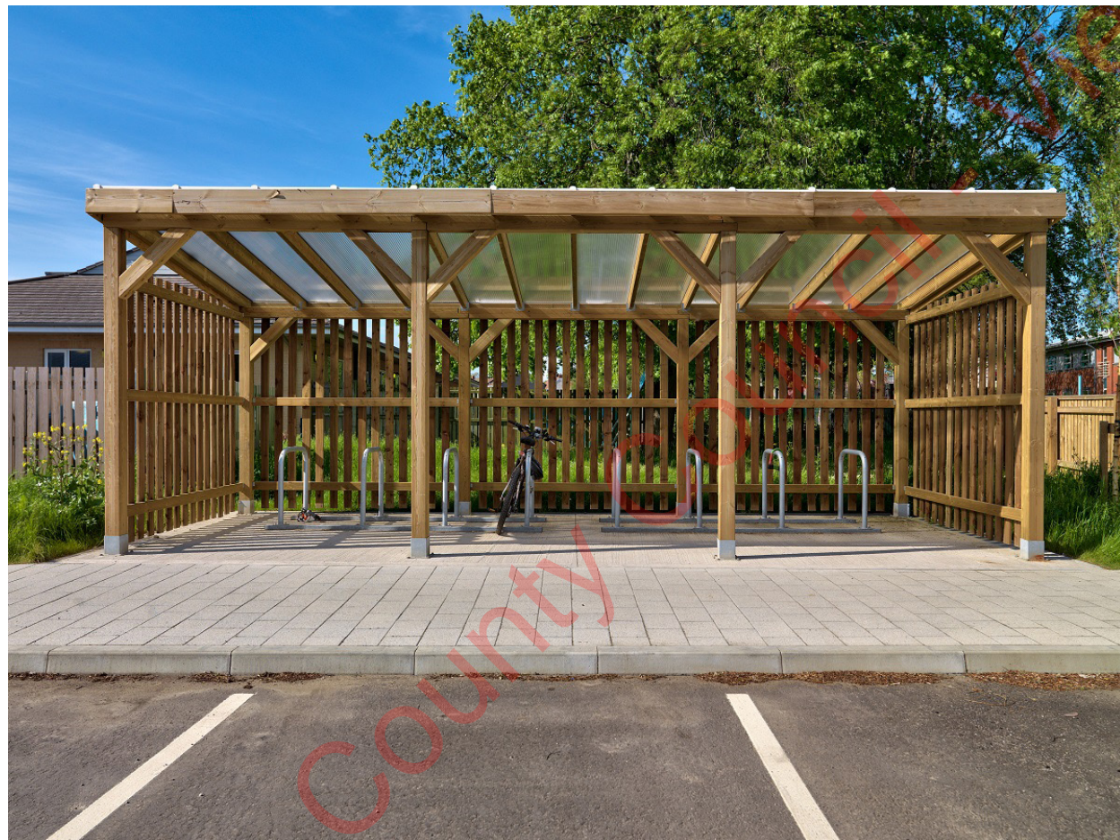
Covered Cycle Storage Area
