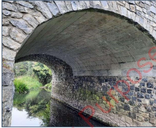
Plate 4-7 Interior bridge view
