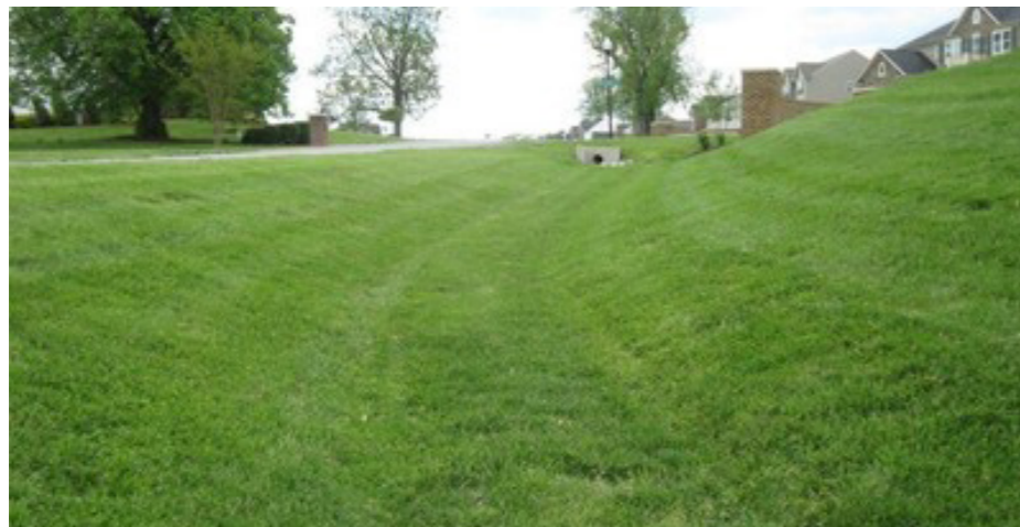
Typical swale in dry weather
