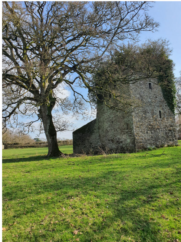
1. Moygaddy Castle - Tower house in ruins
