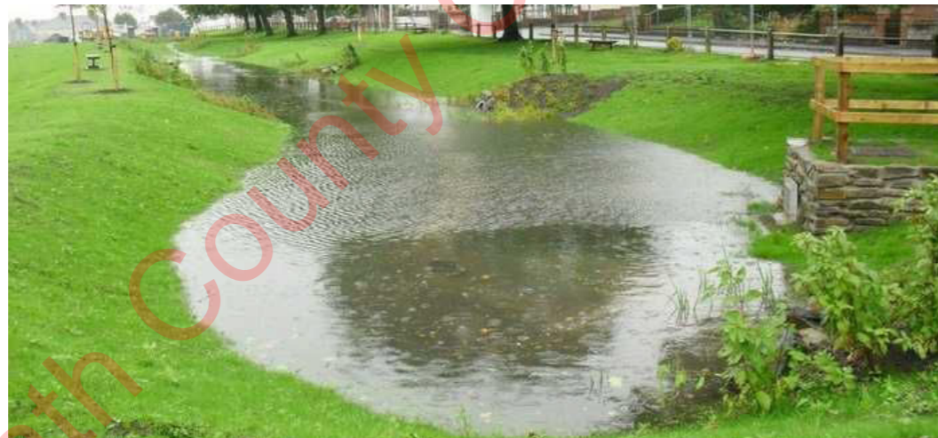
Typical swale in wet weather
