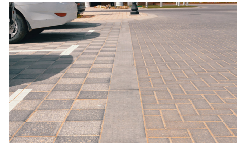
Flush Slipform Concrete Kerb
