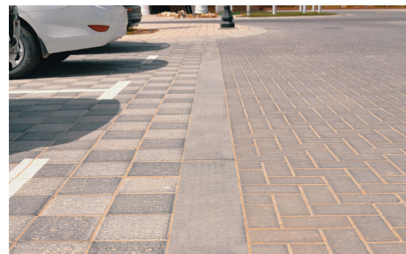
Flush Slipform Concrete Kerb
