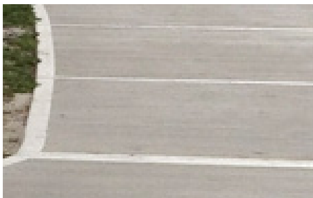
Brushed Concrete with trowel edge finish (streets)
