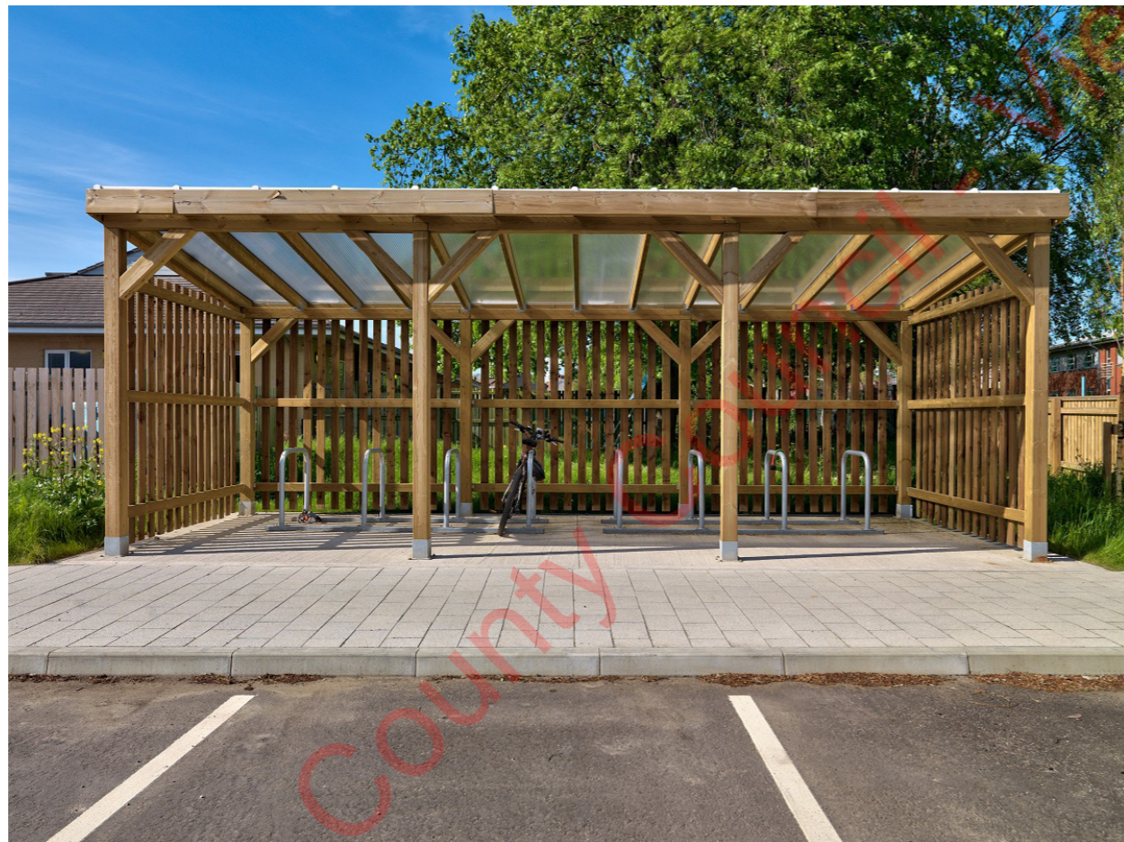
Covered Cycle Storage Area
