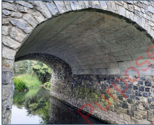
Plate 4-7 Interior bridge view
