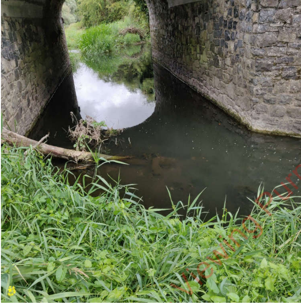
Plate 8-3 Water Levels at SW3 Sample Location (Kildare Bridge) on 5 th of August 2021
