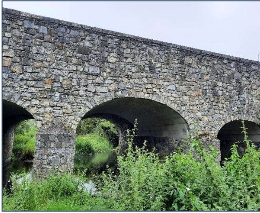
Plate 4-6 Exterior bridge view
