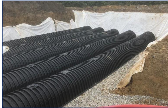
Figure 3.8 – Typical Poly-Tunnel Installation Arrangement
