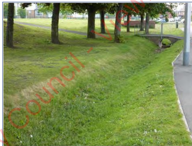
Figure 3.9 – Example Roadside Swale
