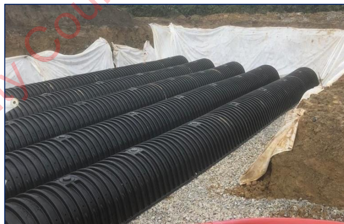
Figure 3.8 – Typical Poly-Tunnel Installation Arrangement
