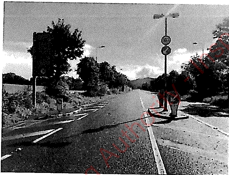
Location 42 - Lissivigeen Splitter Island Exit
