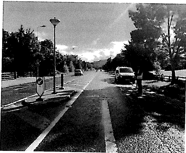
Location 41 - N22 Splitter Island In Lissivigeen
