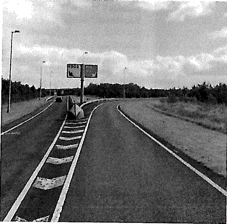
Location 9 - N18/M20 Junction Direction Turn Right Onto M20 Visual inspection indicates that loaded blade component will navigate with no issue
