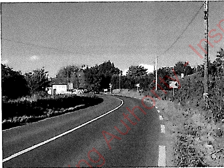
Location 4 - Left Bend On N69 At Junction With L6062
