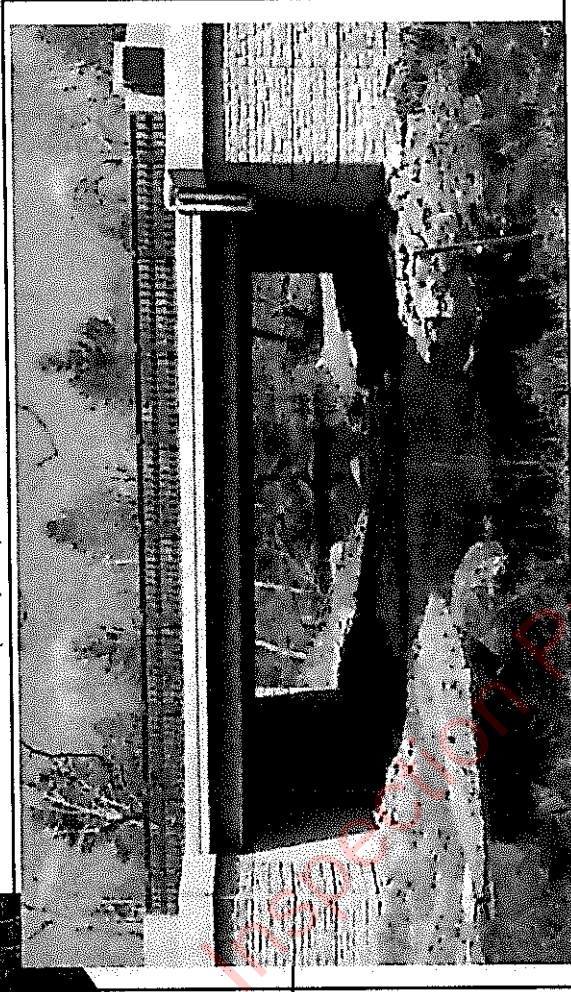
Example of a clear-span bridge which retains the existing river channel, abutments are set back from the river bank (AT&F, 2022)
