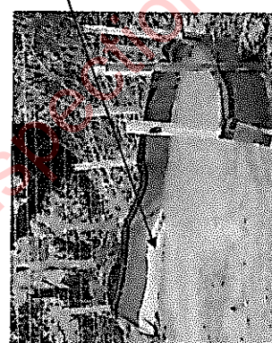
Example of Silt fencing in use (EnviroPro, 2022) Available at: <https://www.enviropro.co.uk/entry/153977/siltbuster/terrastop-silt-fences-for-erosion-and-runoff-control/>
