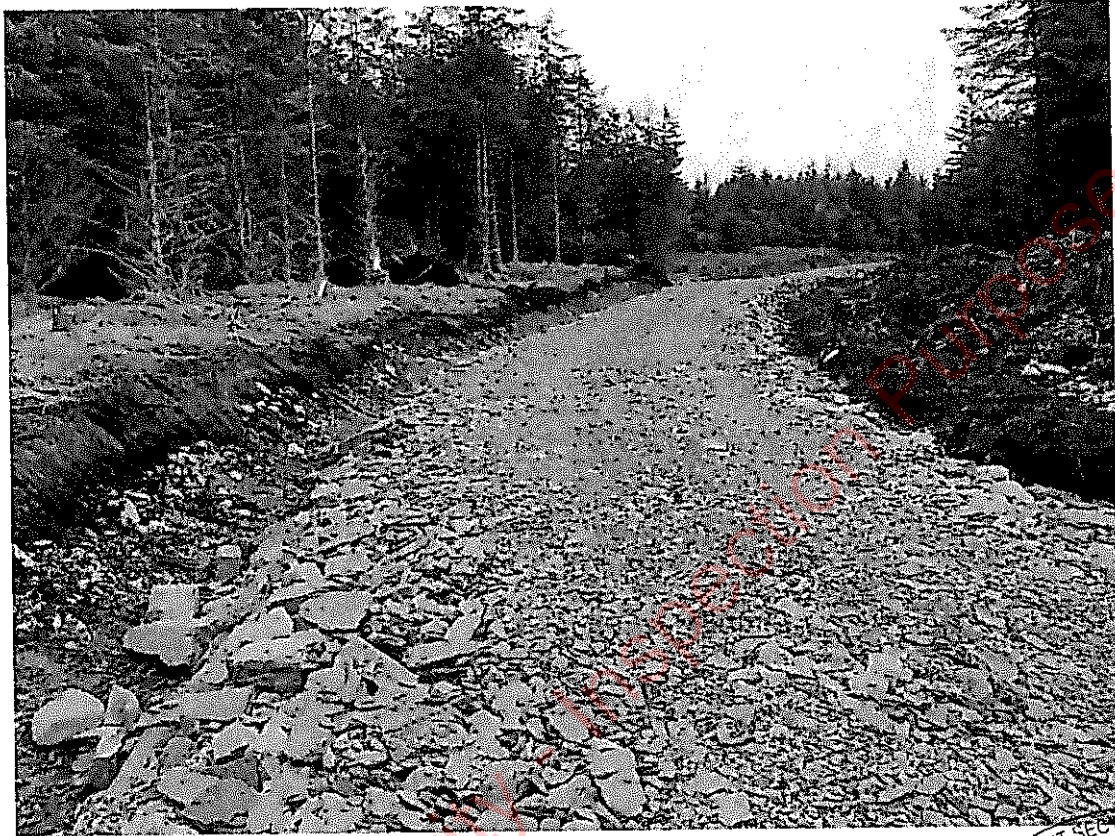
Peat and till exposed at new access track and drainage associated with ongoing forestry activities observed during site surveys.
