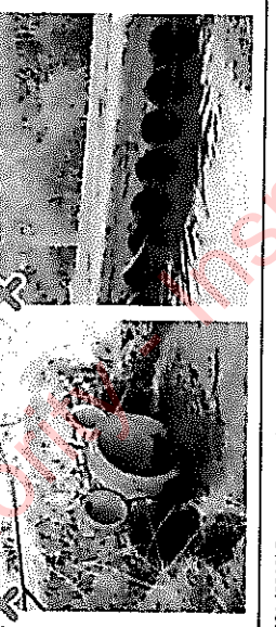
Figure 42: Poor practice: do not use smaller multiple pipes: they can create a barrier to fish passage.
