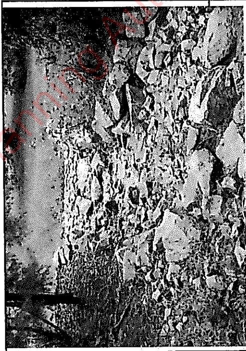
Example of buffered outfall with coarse aggregate (Catchments and Creeks Pty Ltd., 2020)
