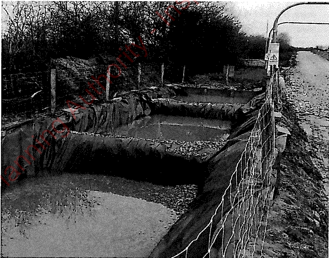
Plate 5.4b: Completed settlement pond system showing levels of settlement
