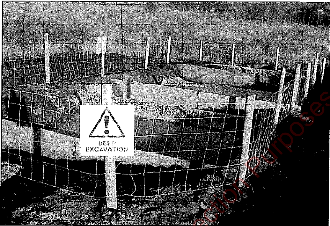
Plate 5.4a: Completed settlement pond system
