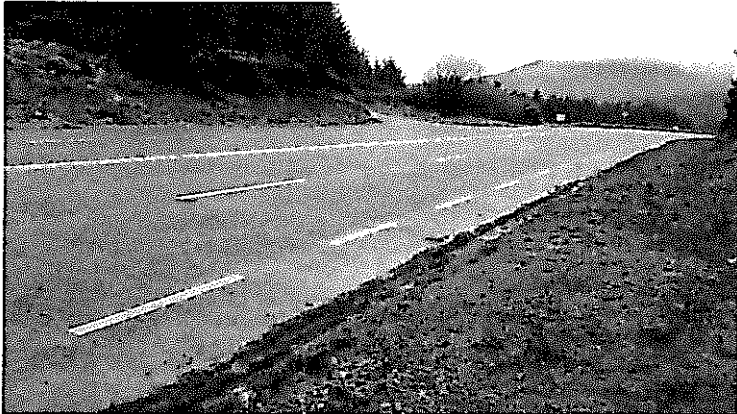
Photo 15.1 – N22 at Derryreag
