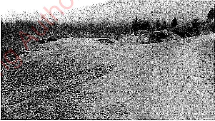
Photo 15.3 – Existing Forest Road at Chainage 1000 m
