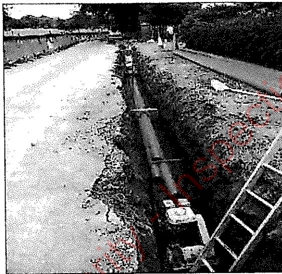
Figure 2 - Typical 38kV Underground Duct Installation
