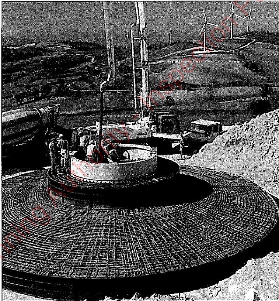
Plate 3.2: Wind Turbine Foundation 6
