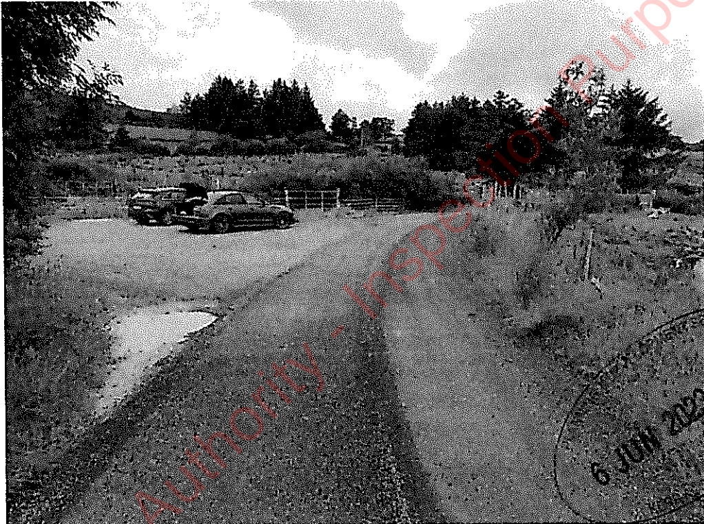
General view of the bridge surface, looking north
