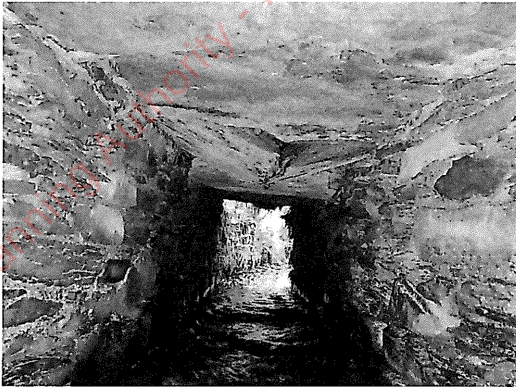
Soffit of bridge deck/box stone culvert. Flag stone is damaged and has collapsed as seen viewed from U/S (north span).
