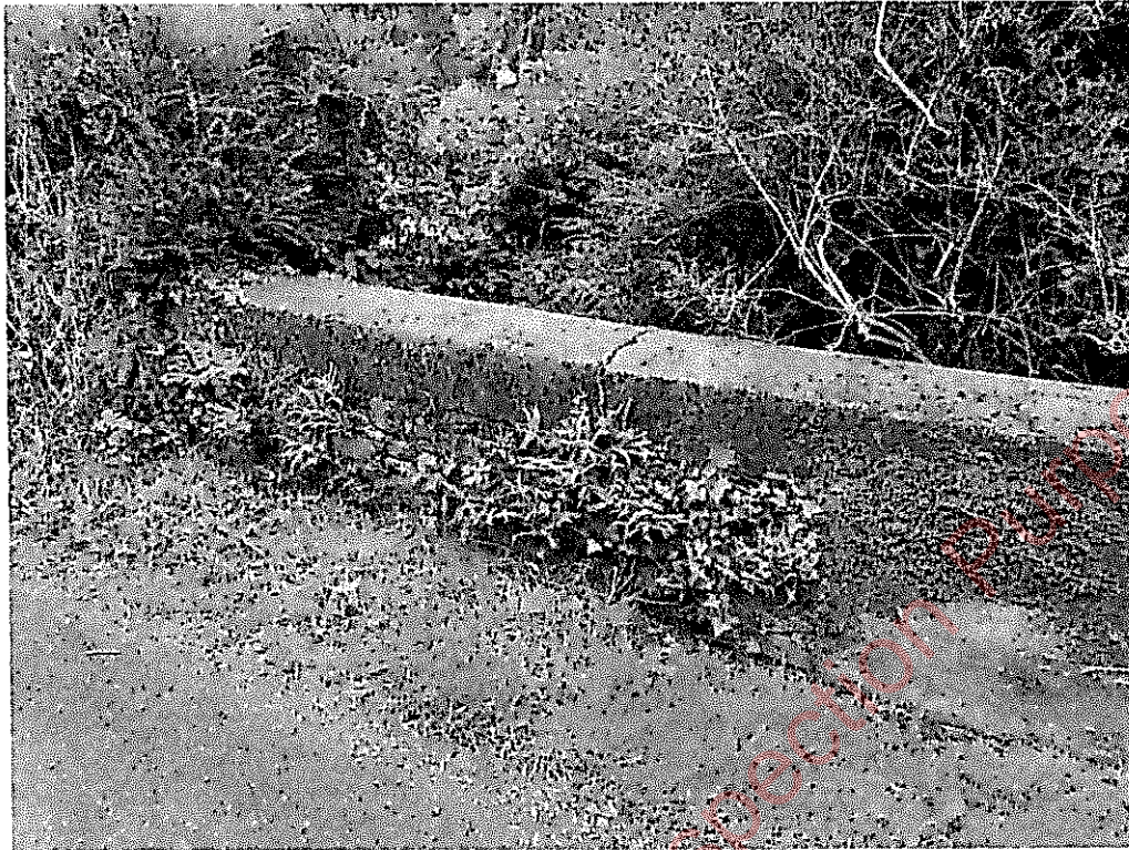
North parapet, west end
