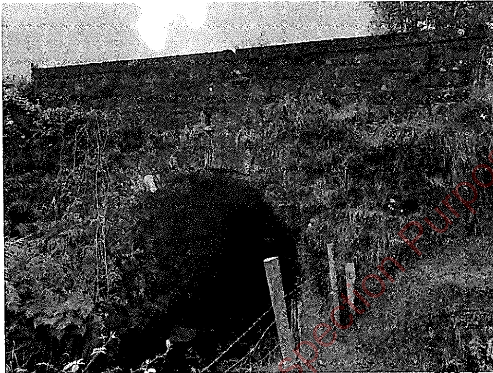
General view of the east elevation
