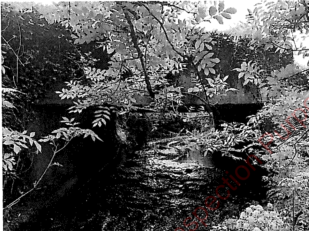
General view of the bridge elevation
