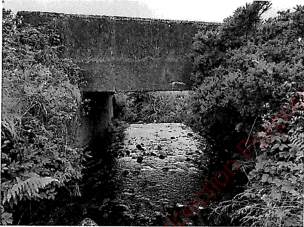
General view of east elevation, looking downstream
