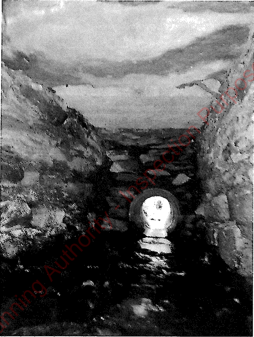
View of south span from the west
