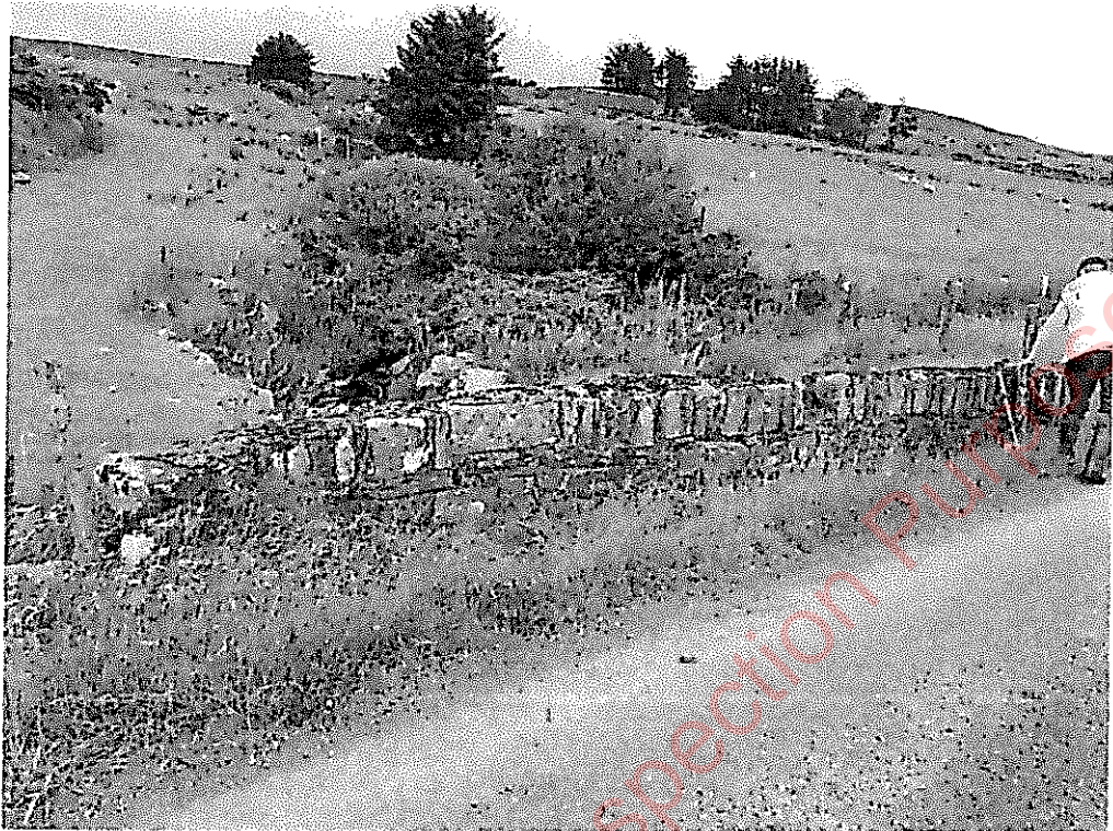
General view of the north parapet
