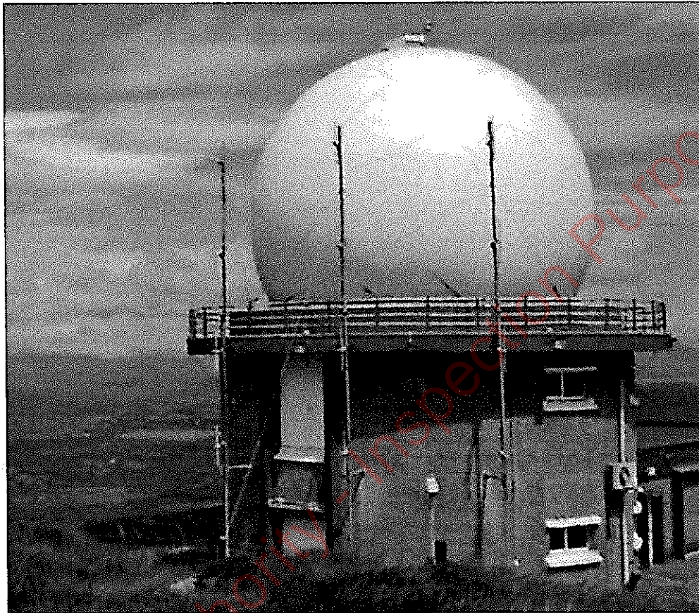
Figure 9. Mt Gabriel Radar Station.
