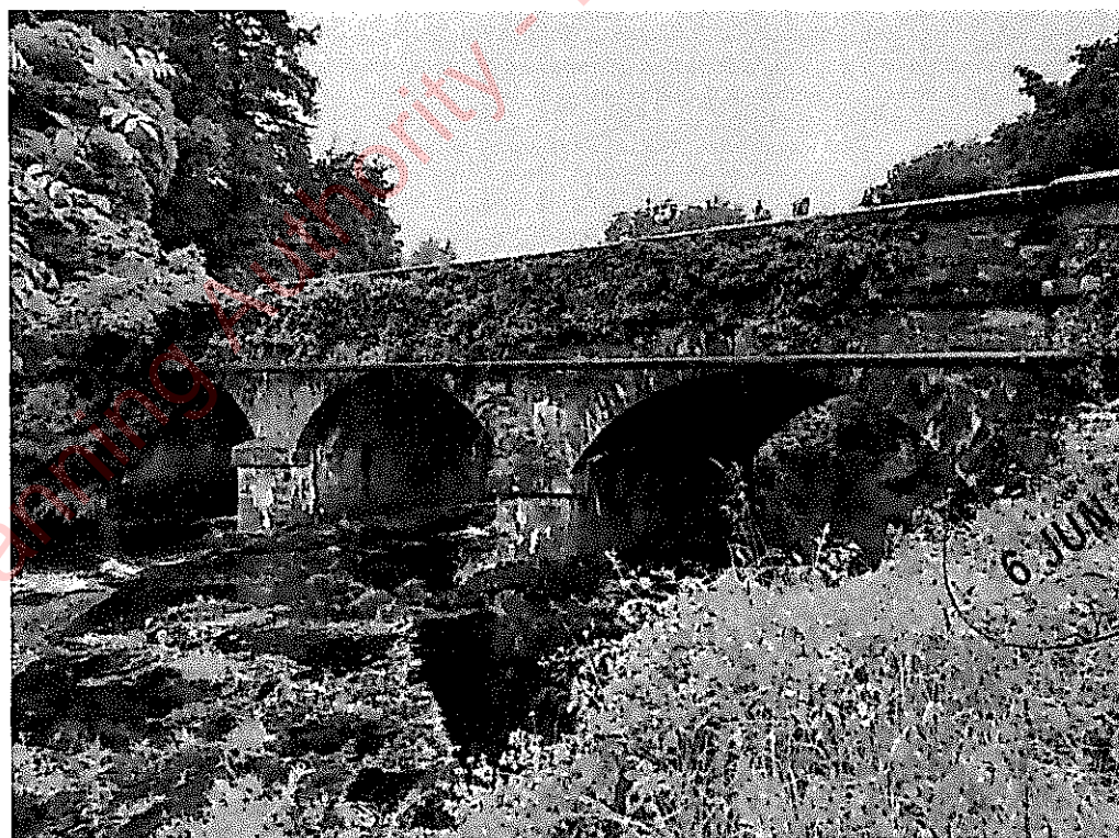
General view of the south elevation
