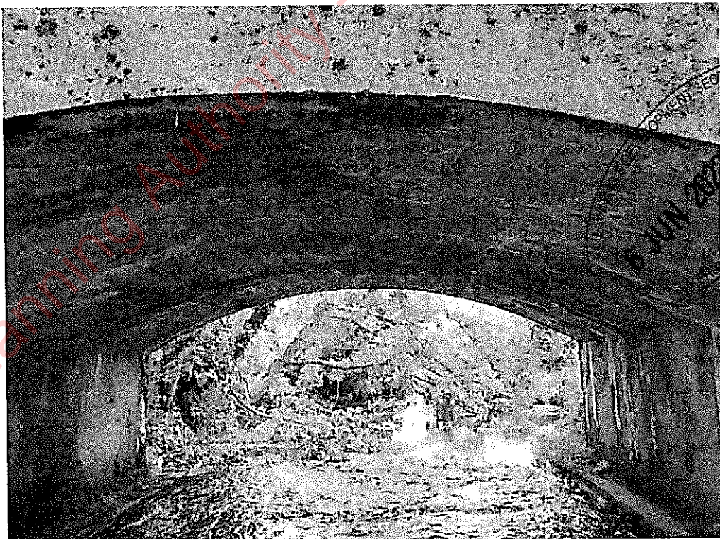
General view of the arch barrel
