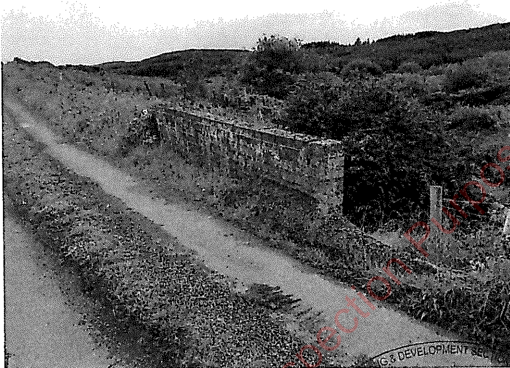
General view of bridge surface and west parapet
