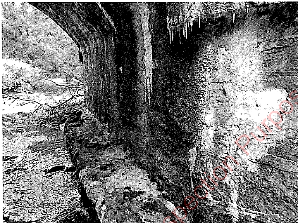
Typical pier condition
