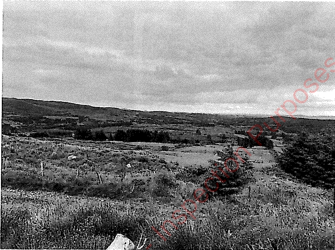
Image : 88 Ballyvouskill substation to the north of this image
