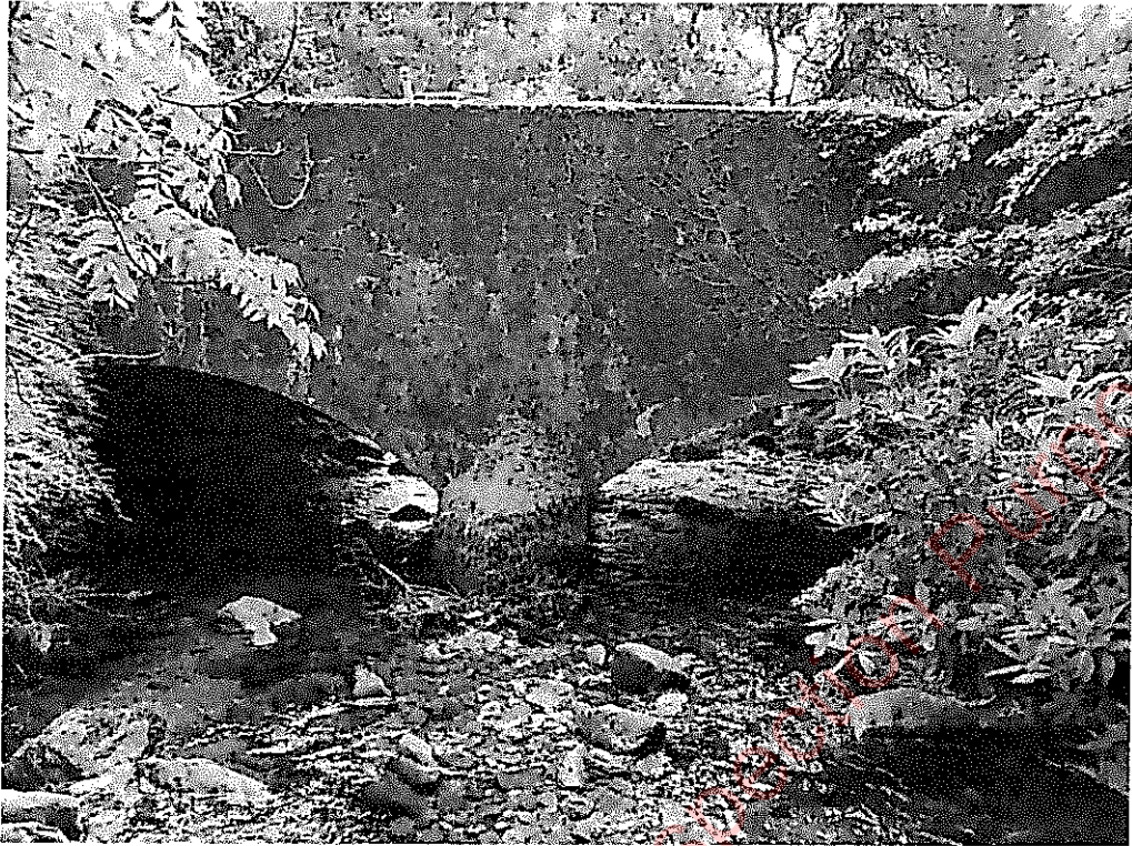
General view of the west elevation
