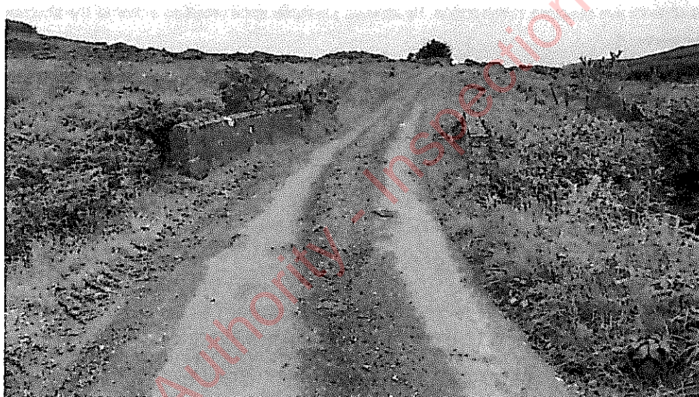
General view of the bridge surface looking south
