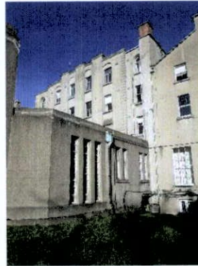
Fig. 37 The later southern central extension in context with the Archive.
