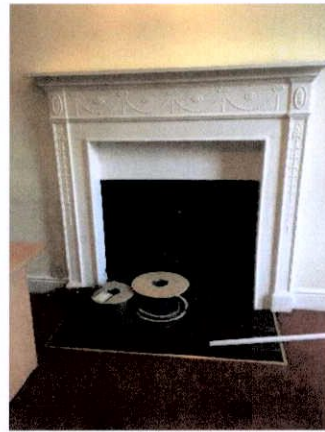
Fig. 32 Early chimney piece with later tiled inset and hearth, in same room.
