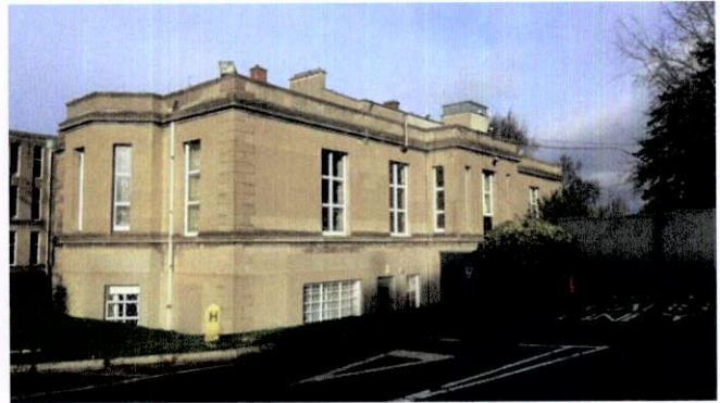
Fig. 44 View of east elevation
