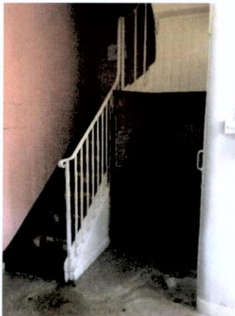
Fig. 70 Secondary steel stair of interest
