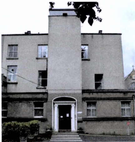
Fig. 21 Present day configuration of east (front) elevation of Milltown Park, with the vertically extended entrance lobby; vertical extension to south (denoted by higher level windows) and repositioning of first floor windows
