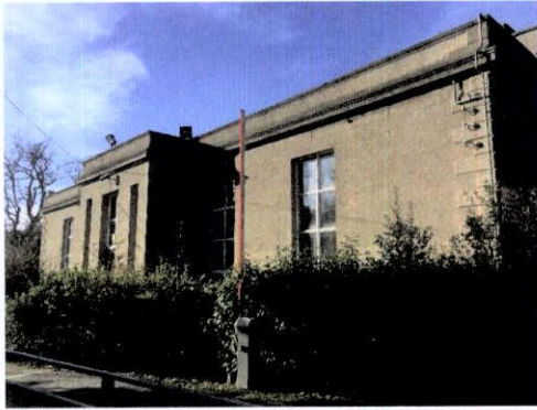
Fig. 43 View of east elevation
