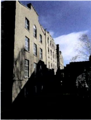
Fig. 41 View from west
