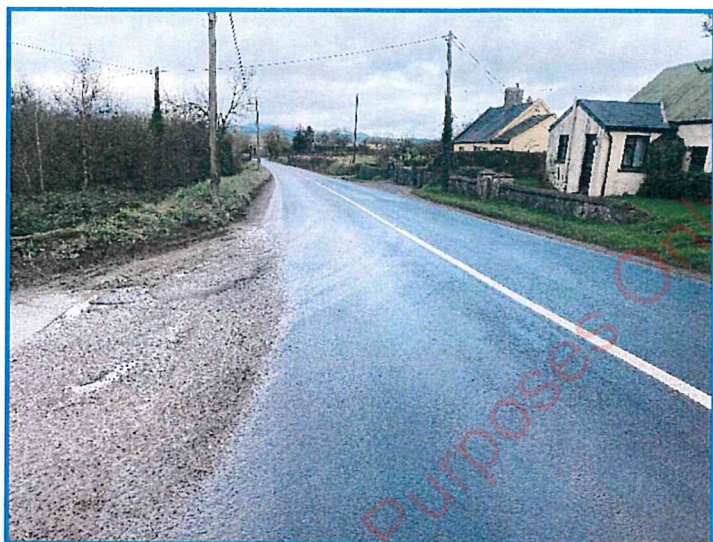
Photograph 14. 2: Northbound view Existing site access.
