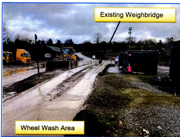
Photograph 14. 4 View of existing weight bridge within quarry site.
