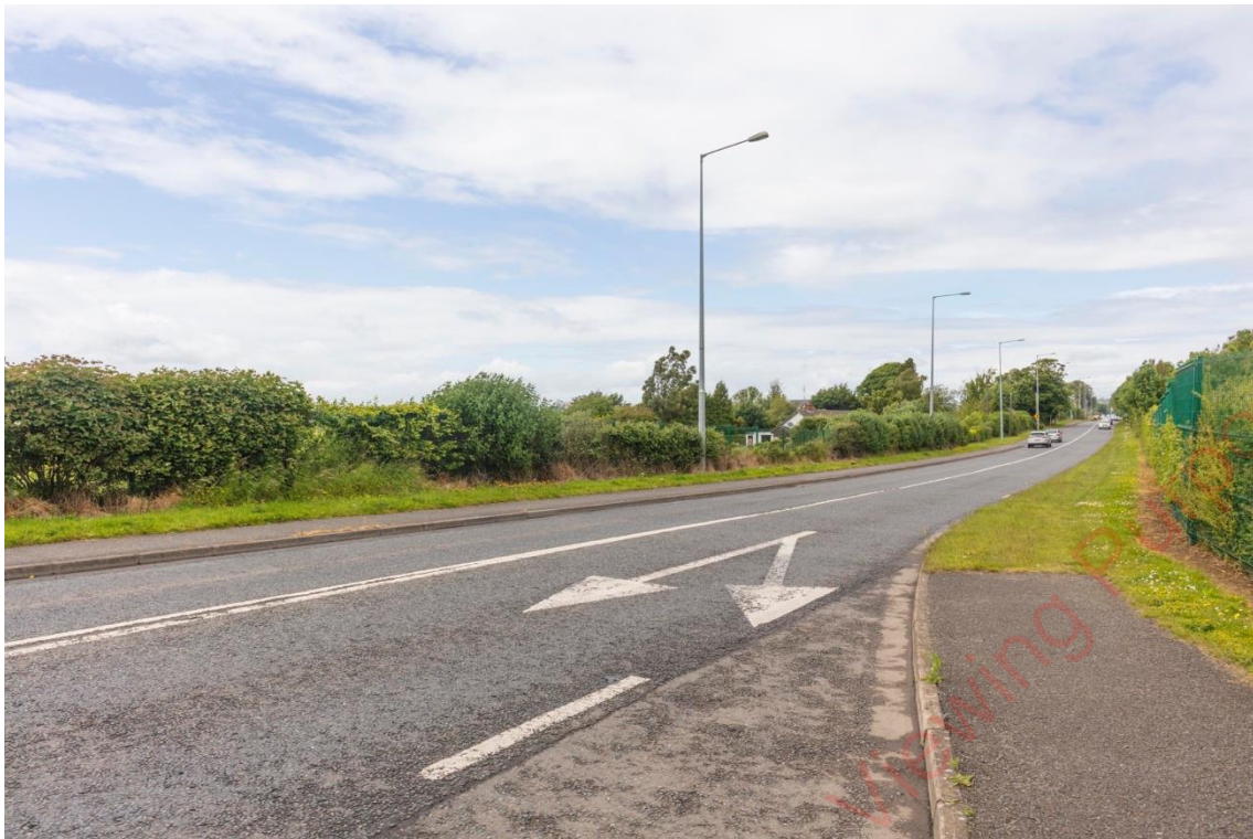
Figure 10-48: Viewpoint H, R168 (Trinity St.), Existing View
