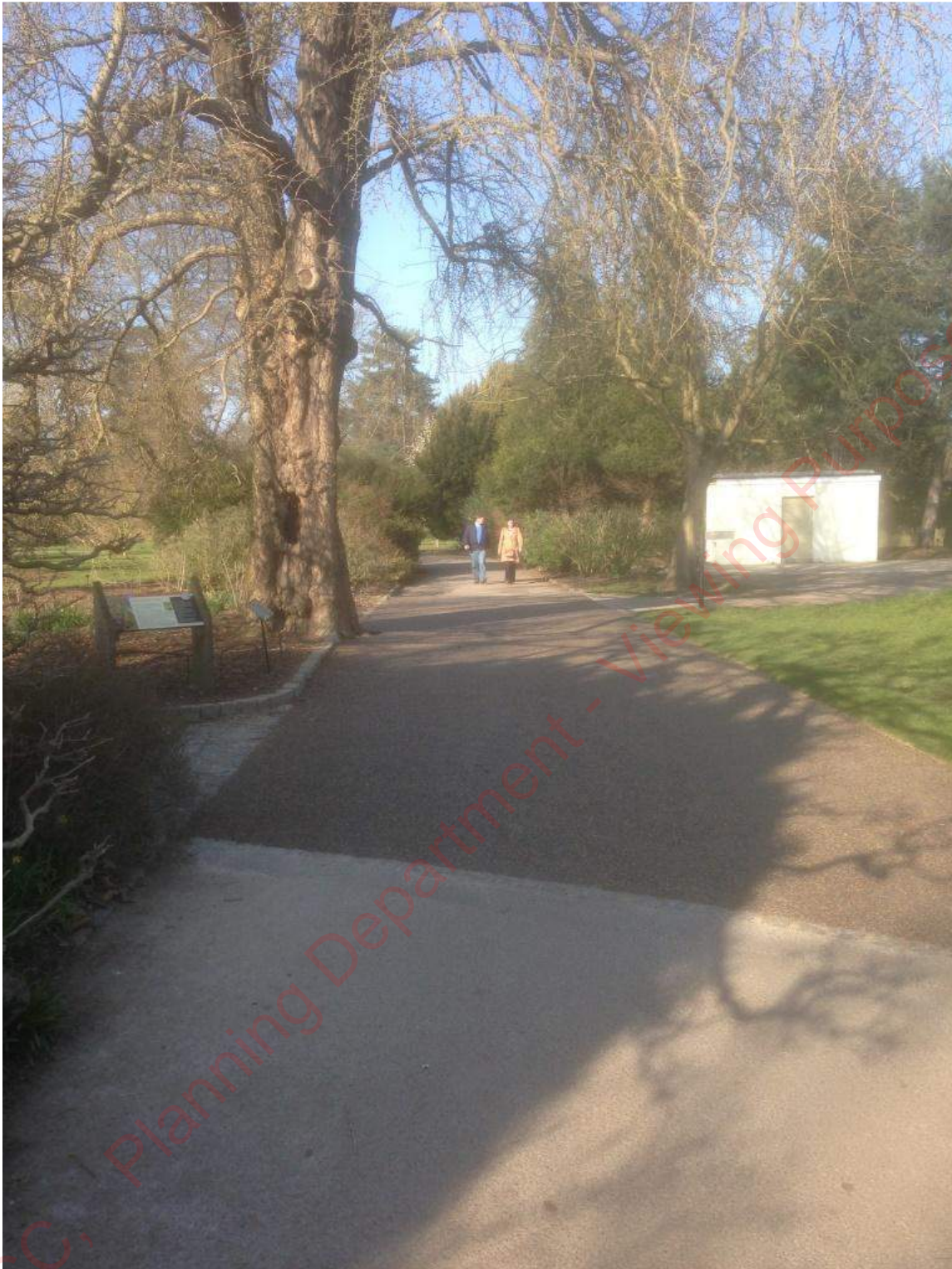
Photo 11 -Resin Bonded Gravel used across a root-plate of the TROBI Champion Ginkgo at Kew Gardens (London)
