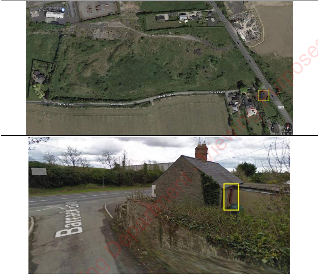
Barrack Lane – Existing Property 01
