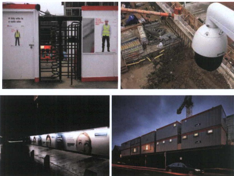
Figure 8 – Typical Site Security Measures
