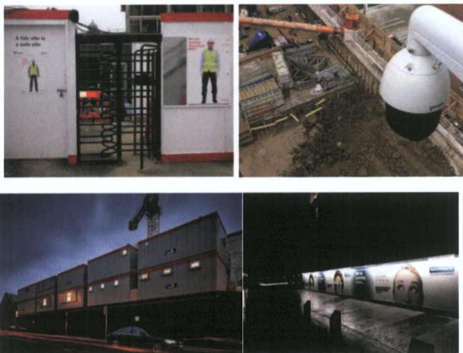
Figure 32. Typical Site Security Measures
