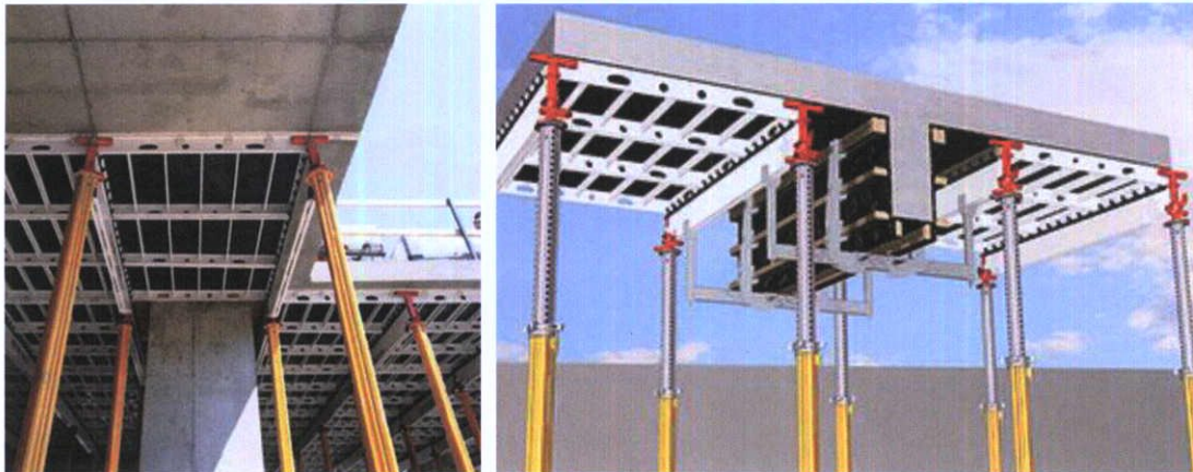
Figure 20 - Typical RC Formwork (Skydeck)
