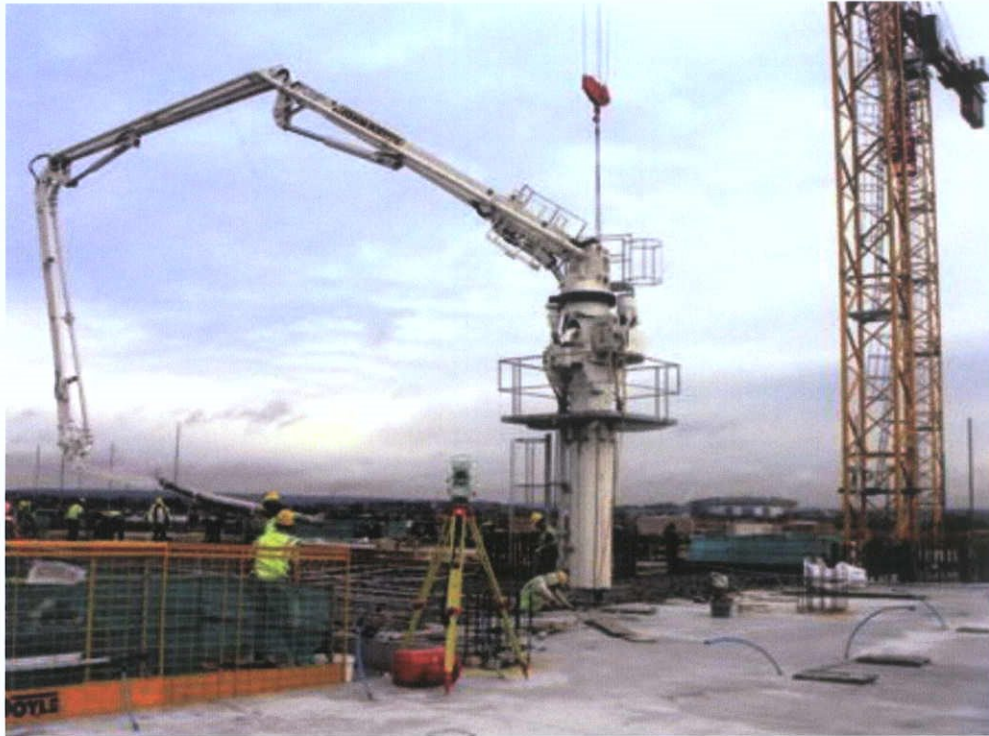
Figure 21 - Typical Concrete Placement
