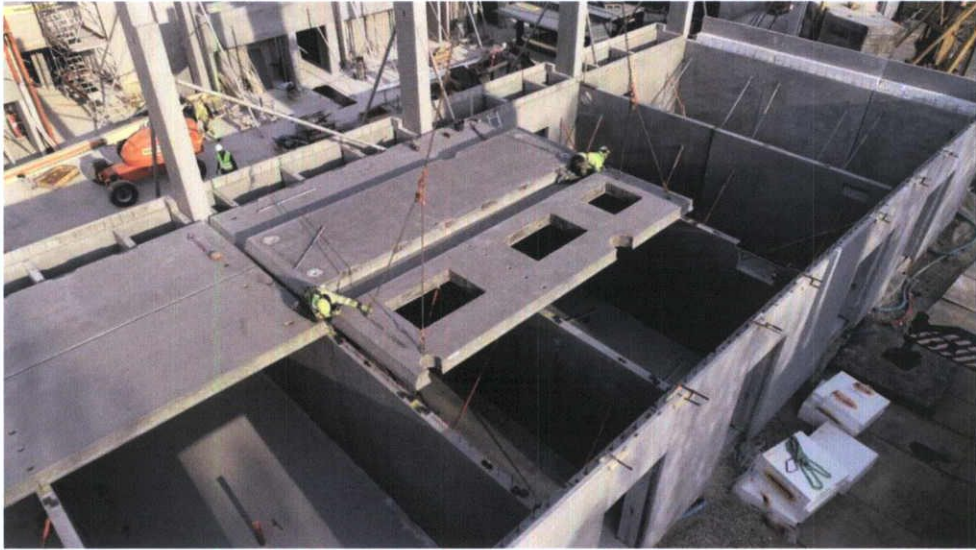
Figure 24. Typical Precast Concrete Construction
