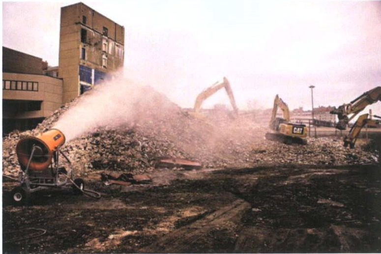
Figure 45 – Typical Dust Mitigation Measures
