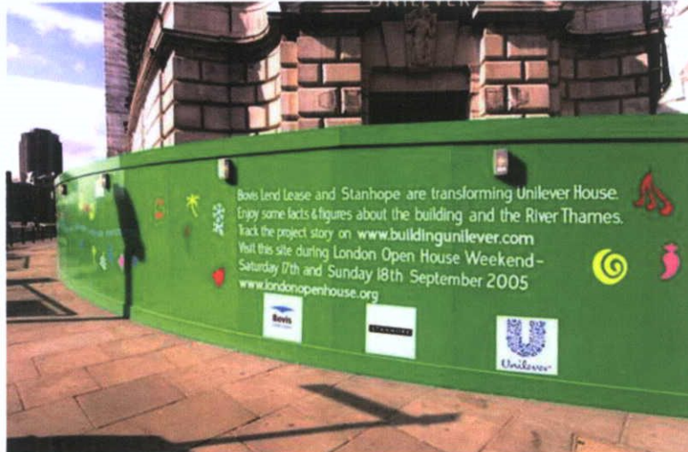
Figure 3 | Typical Perimeter Hoarding
