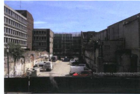
High level view of vacant site. Note niches and indentations in boundary walls. Front wall onto O'Connell Street and rear wall onto Moore Lane have been removed.
