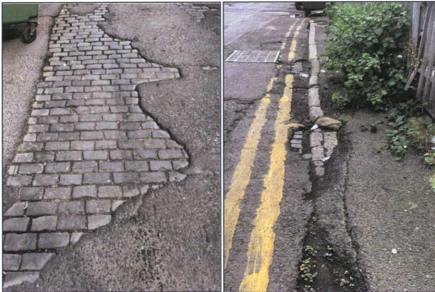
Plate 5 Relic street kerbs and paving
