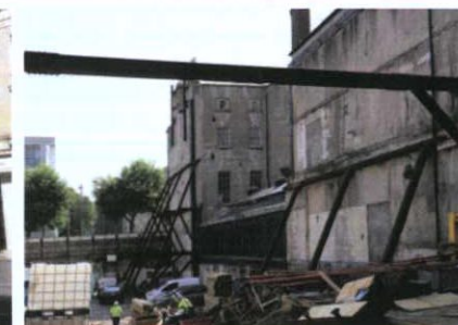
Interior of vacant site
