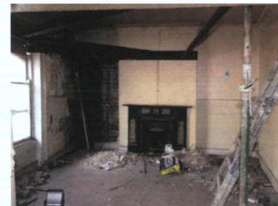
Upper floor, note structural propping
