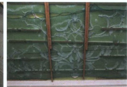
Sample of decorative plasterwork
