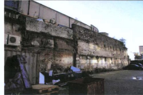
Indentations to southern boundary wall at No.51 suggesting a large-scale industrial type structure
