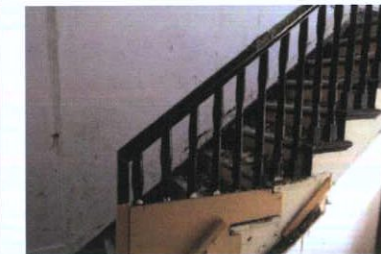
Detail of stair
