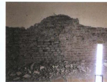
Creep hole at first floor level
