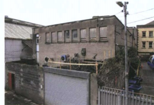
Rear elevation onto Moore Lane
