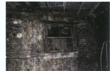
Sash window within modified structure
