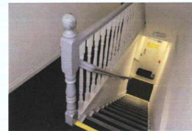
Good early 20th century staircase
