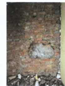
Creep hole at entrance level
