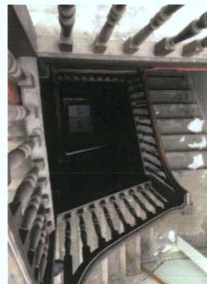
Staircase from 3rd floor level
