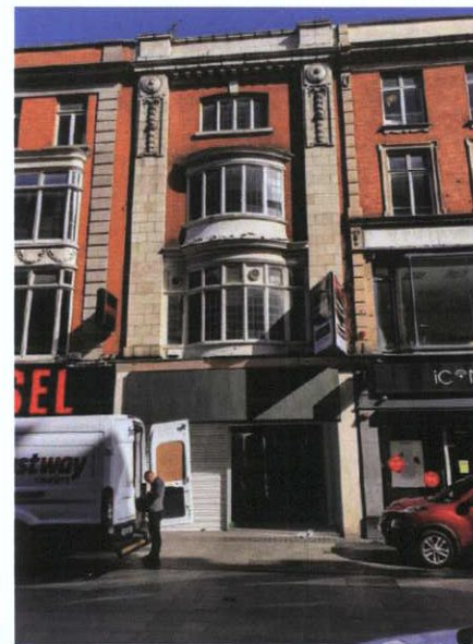
Front façade 37 Henry Street, oriel window, detail of stucco work, stair
