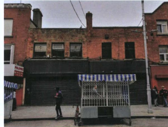
Front façade 18 Moore Street, right-hand-side
