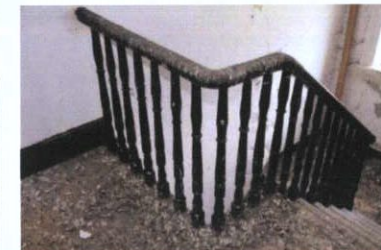
Turned balusters and timber handrail
