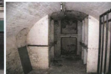
Vaults at basement level within rear buildings
