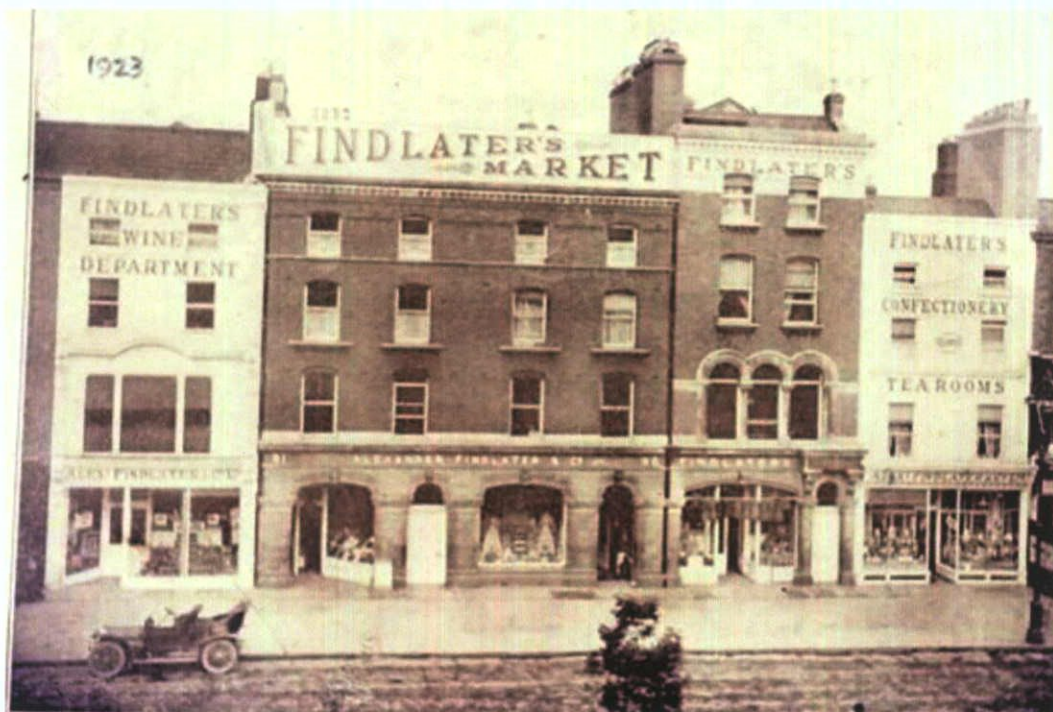
Figure 4.6 East side of the north end of O'Connell Street before 1923. Several plots combined for a single enterprise – Findlater's. Lettering imposed on building fronts. (Courtesy of Dublin City Library and Archive)
