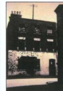
P 25 View of same building depicted in P23, depicting the entirety of the front façade.
