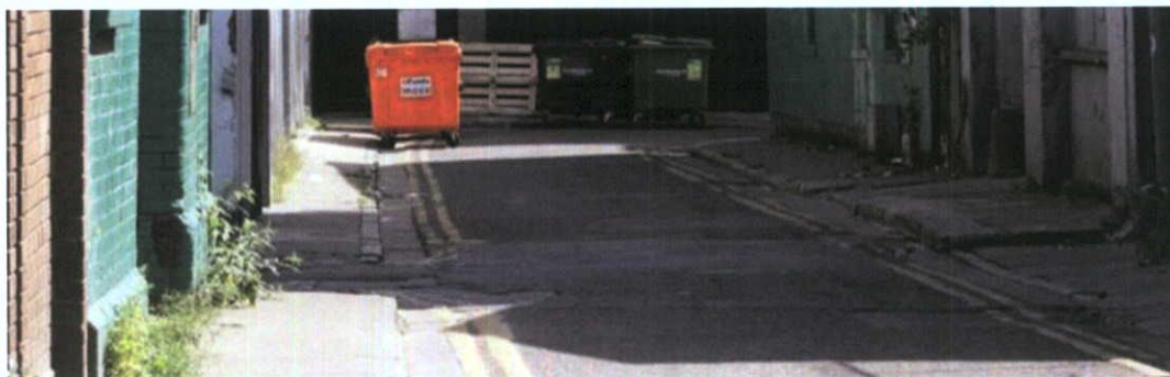
Figure 9.17 Henry Place some surviving sections of pavement. A section on the right has larger width granite kerbstones. 2020
