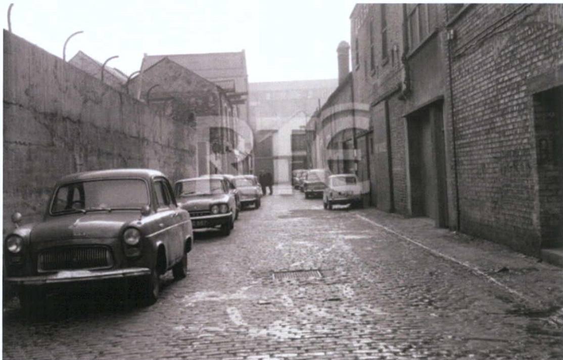
Figure 9.14 Looking south down Moore lane paved with setts and grade to drain to gutters either side. (RTE Archive)
