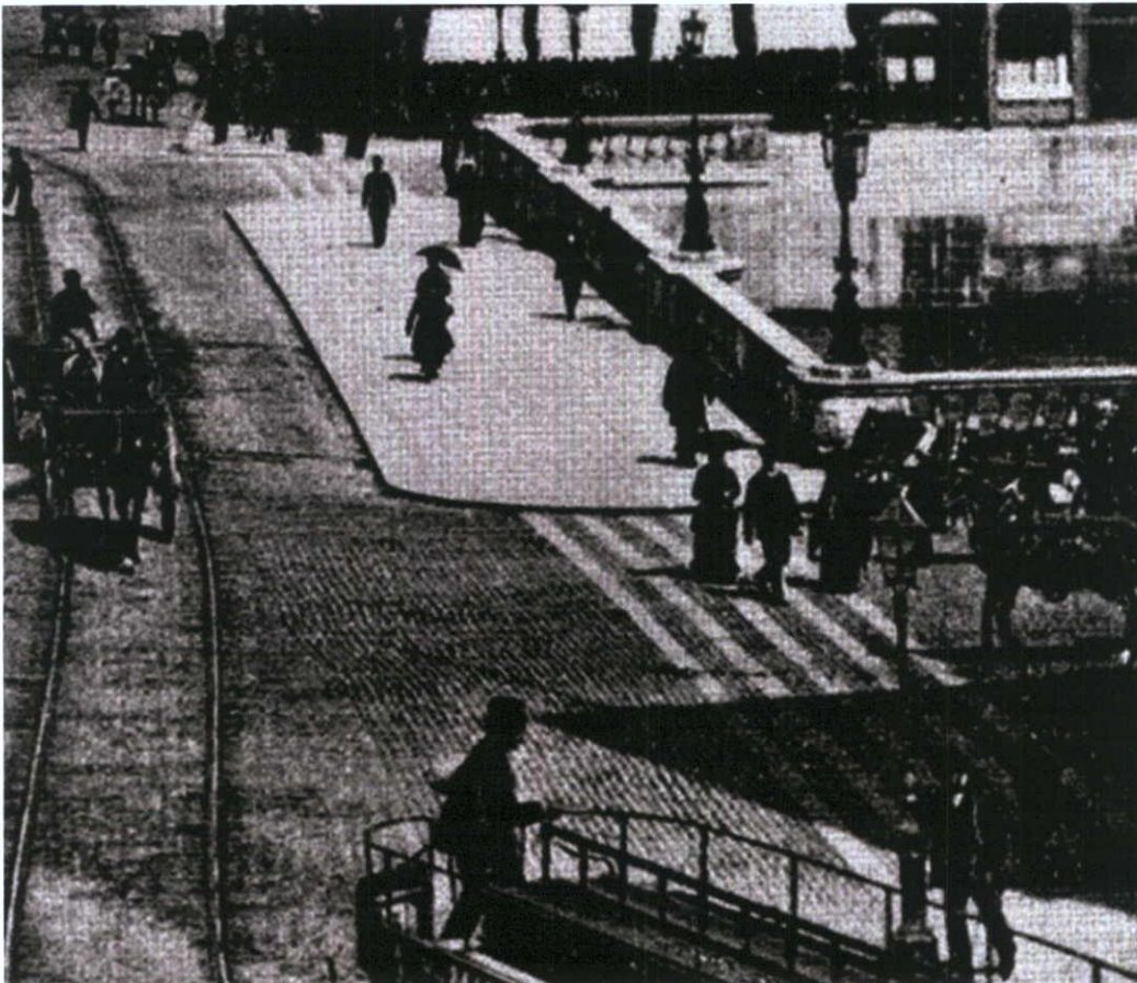
Figure 9.21 Carlisle Bridge late nineteenth century. Apparently, different coloured setts were used to define the junction and indicate the crossing for pedestrians. The ladies appear to use the light coloured area to cross, indicating that it may have been smoother and easier to walk on. 1892 (Military Archive)
