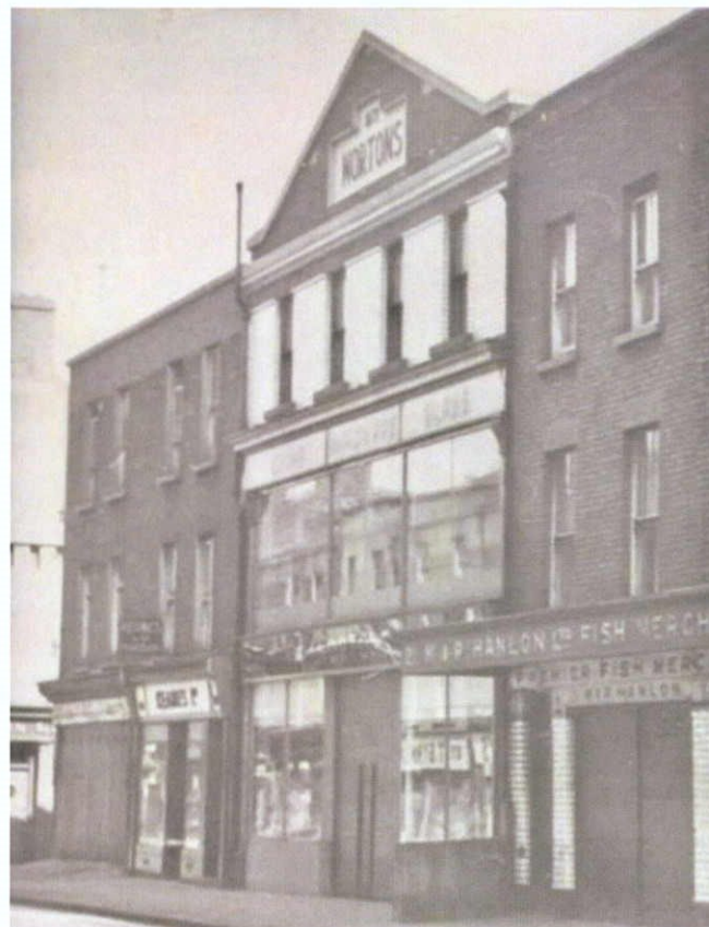
Figure 8.12 A single building had occupied the plots of 22 and 23 Moore Street with a completely glazed first floor display. (Military Archives)
