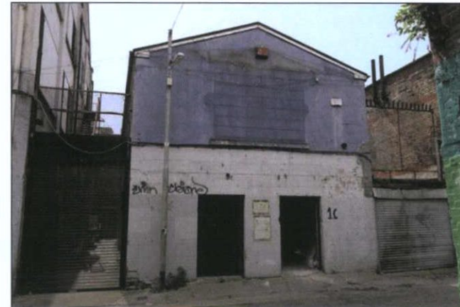
P 23 Northern façade of 10 Henry Place, facing Moore Lane. (2020)
