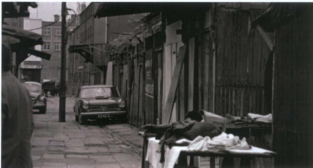
Figure 9.19 Looking east towards Moore Street, the original mews lane to Parnell Street, later part of the Moore Street market zone and most recently called Riddle's Row. 1972 (Courtesy of Dublin City Library and Archive)
