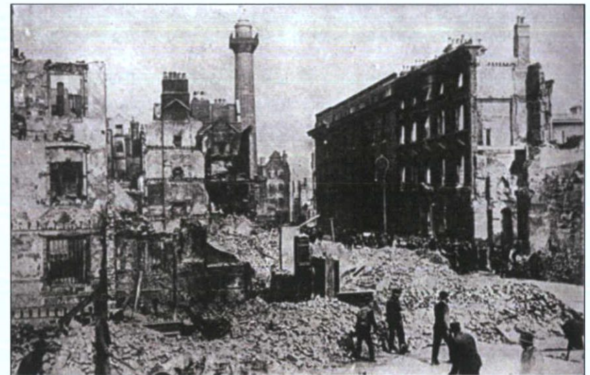
P 6 View of junction of Henry Street and Moore Street, Source: Warhistoryonline.com
