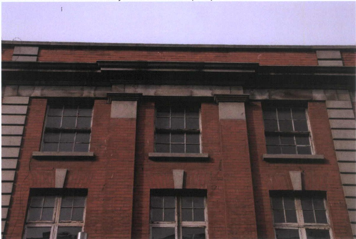
Fig.4.3.2: The superstructure is built with machine-cut red brick with granite used for architectural detailing. The granite shows brown staining, but the building surface is generally free from soiling and has been cleaned in the past.
