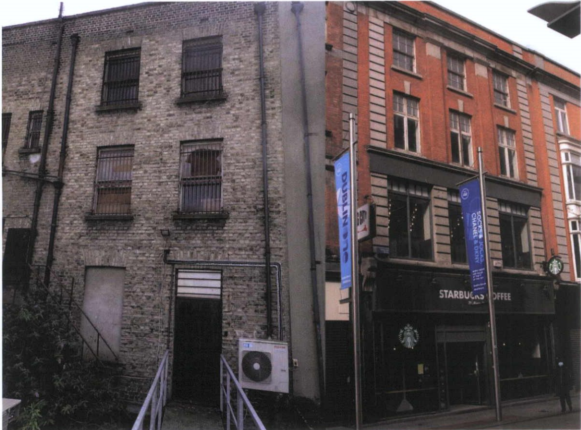
Fig.4.3.1: General views of the rear elevation (note rebuilt parapet) and façade of 39 Henry Street. The rear elevation brickwork matches that of No.38 and is contemporary with same.
