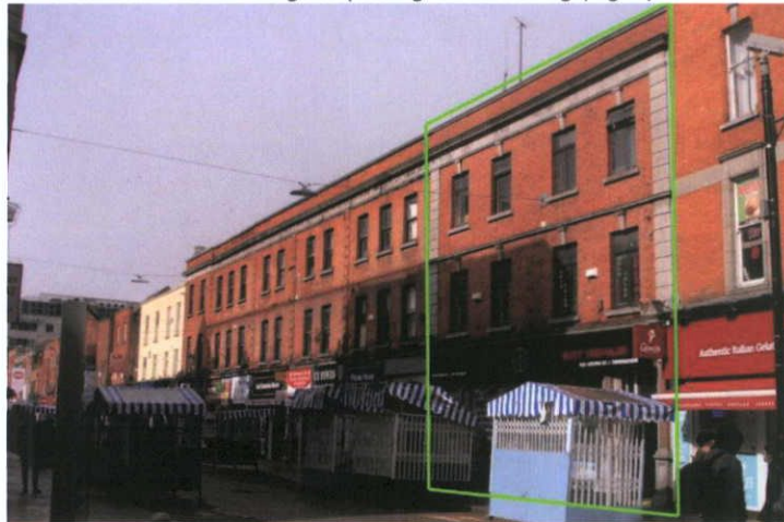
Fig.4.6.2: 1-2 Moore Street. The brickwork is remarkably free from soiling, indicating that it has been cleaned in the relatively recent past.
