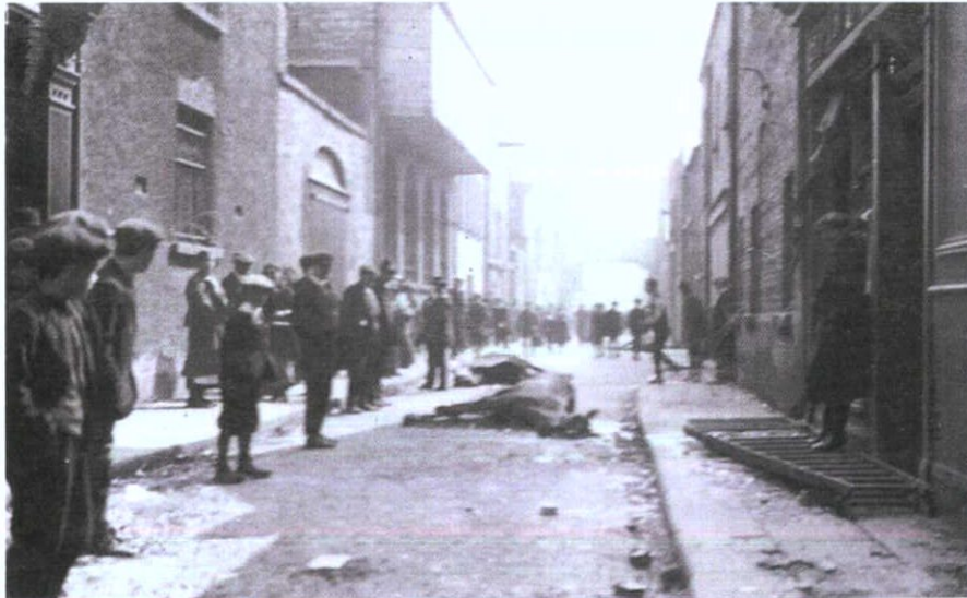
P 45 Moore Lane in the aftermath of the 1916 Rising, View looking south from the Parnell Street towards Henry Place.
