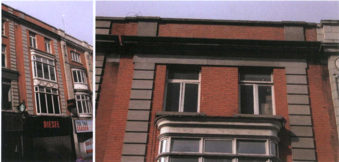
Fig.4.2.1: The façade of 38 Henry Street is of well-fired red brick with limestone detailing, with the parapet rebuilt in a different brick and heavier Portland Cement-based mortar.
