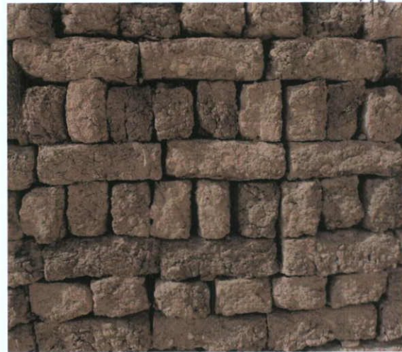
Fig.3.4: 'The Brick Children' from 'The Graphic', Saturday 27 May 1871, with a pug mill in the background; and a detail showing hand-made bricks which had been laid out to dry and then stacked.
