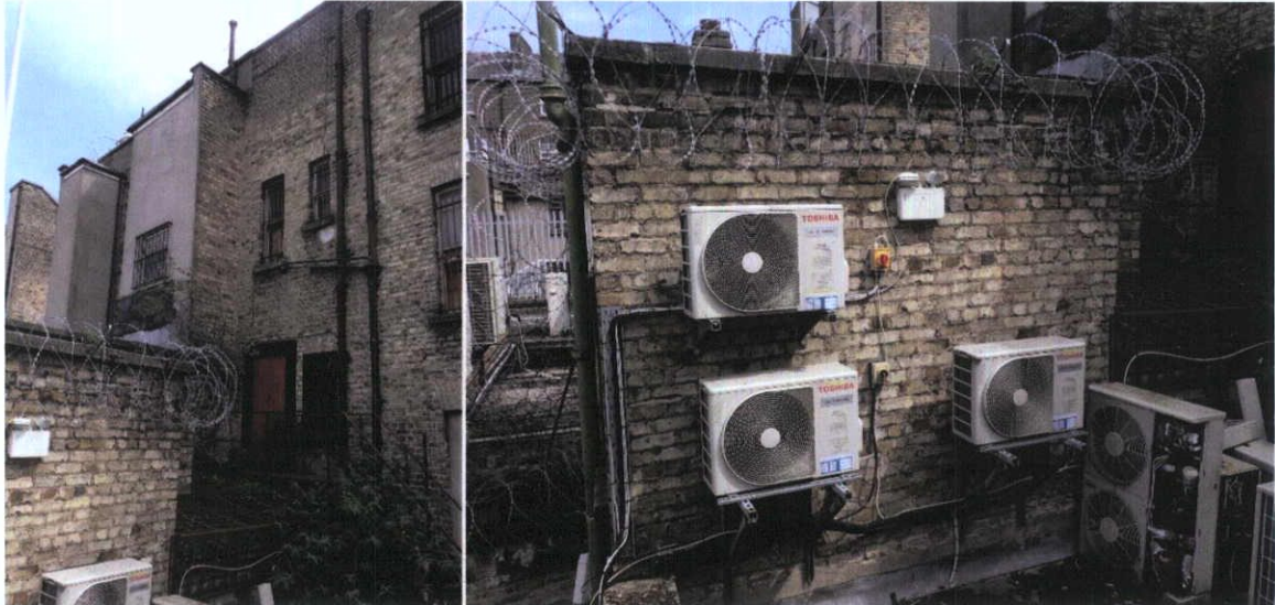
Fig.4.2.4: Yellow stock brick masonry fabric used for the rear and for the return of the building. The same brick is used in the neighbouring rear elevations of Nos.37 and 39 Henry Street, and all three buildings appear to have been erected at the same time.
