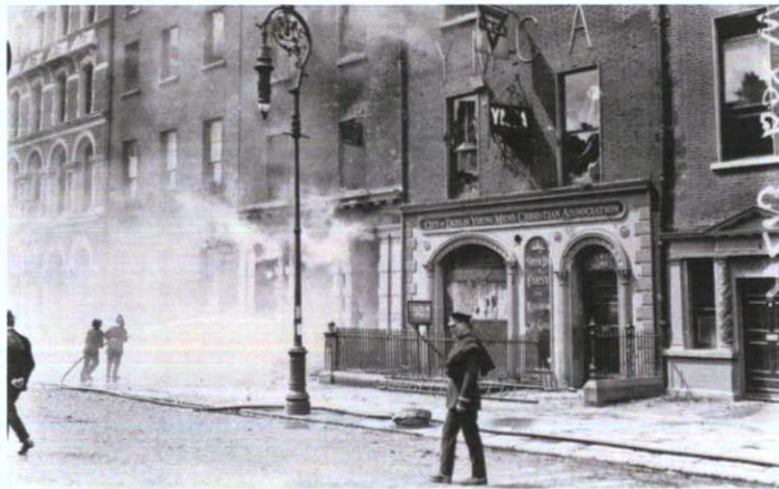
P 51 43 and 44 Sackville Street following the fire.
