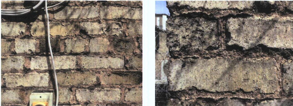
Fig.4.2.5: Slightly pinkish coloured bedding mortar due to the presence of abundant brick aggregate.
