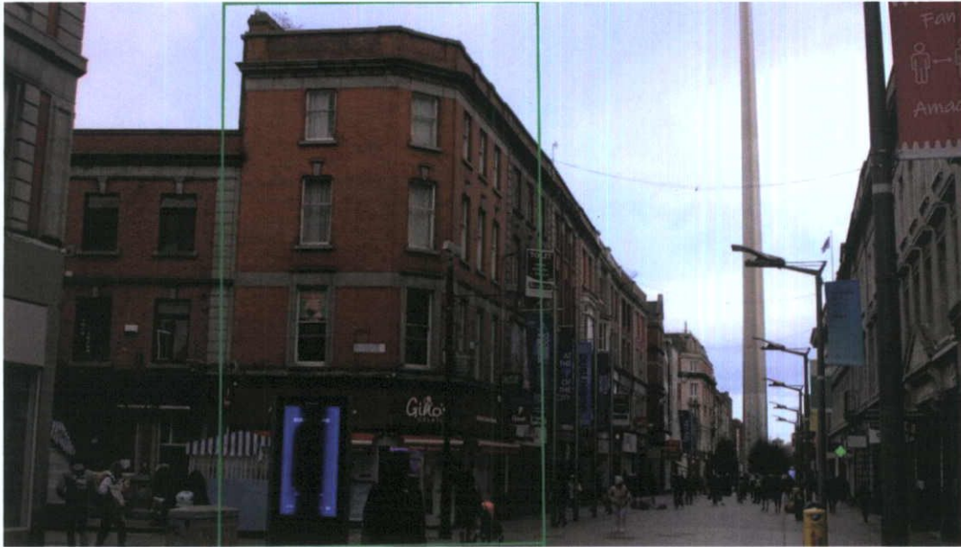
Fig.4.5.1: The brickwork on the soiled façade of No.40 Henry Street consists of well-fired machine-cut red clay brick with weatherstruck Portland Cement-based pointing mortars. Leinster granite was used for architectural detailing. The work probably dates to c.1917-1920.
