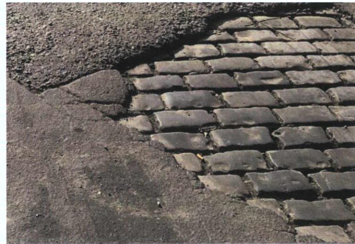
P 40 Detail of smoothly worn diorite setts on Moore Lane.
