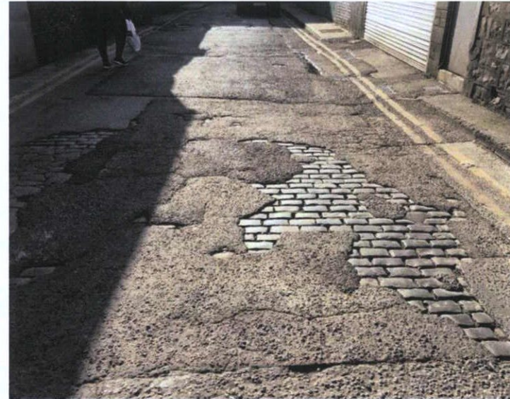
P 39 Original setts on Moore Lane visible under modern road surface.
