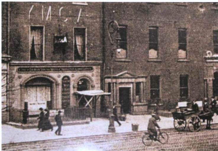
P 50 43 and 42 Sackville Street prior to 1922.
