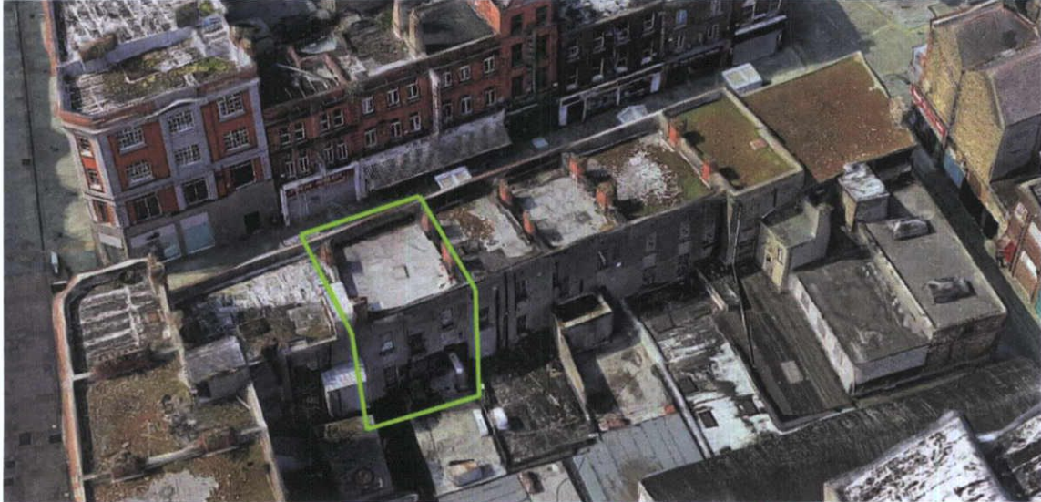
Fig.4.7.5: GoogleMaps view showing the flat roof and rendered rear elevation of the building.
