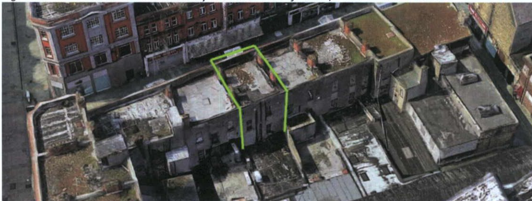
Fig.4.8.3: GoogleMaps view of the roof and rear elevation of No.4 Moore Street.
