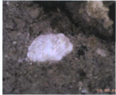
Fig.4.16.10: Cementitious bedding mortar seen externally at the north end of the east elevation.
