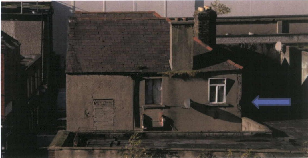
Fig.5.1.5: The rear of No.10 Moore Street is rendered. The north side (arrowed) was opened up.
