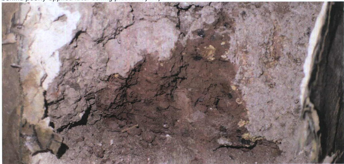
Fig.4.12.7: Hand-made clamp-fired brick with angular limestone aggregate similar to that seen at No.42 O'Connell Street and other Georgian buildings in the area. This type of brick may have been fired at the Moore Street brickfield.
