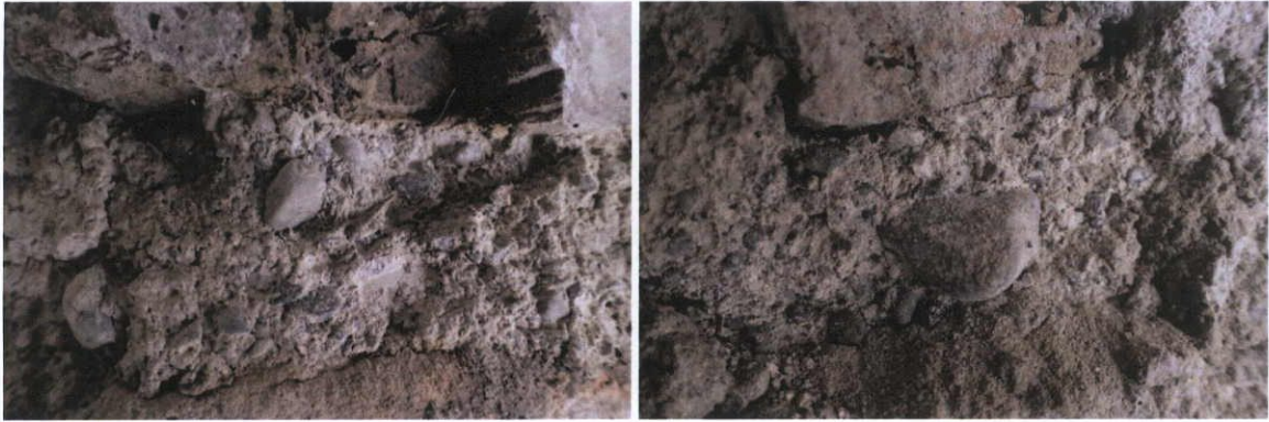
Fig.5.3.6: The original bedding mortar is lime based, without obvious pozzolanic additions, and containing rounded limestone pebble to gravel-sized aggregate.
