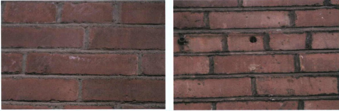
Fig.4.14.5: The brick at first floor level is remarkably free from airborne particulate soiling (which is commonly found on building surfaces which have not been previously cleaned in Dublin City). Some soiling is found on the weatherstruck joints – suggesting that the brickwork was either cleaned (or possibly built) not too long before the Air Pollution Act 1987.
