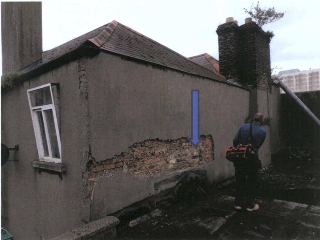
Fig.5.1.6: Exposed brickwork beneath Portland Cement render, north elevation, 10 Moore Street. The masonry has been disturbed and appears to be a 'creephole' (arrowed). See Fig.5.1.9 also.
