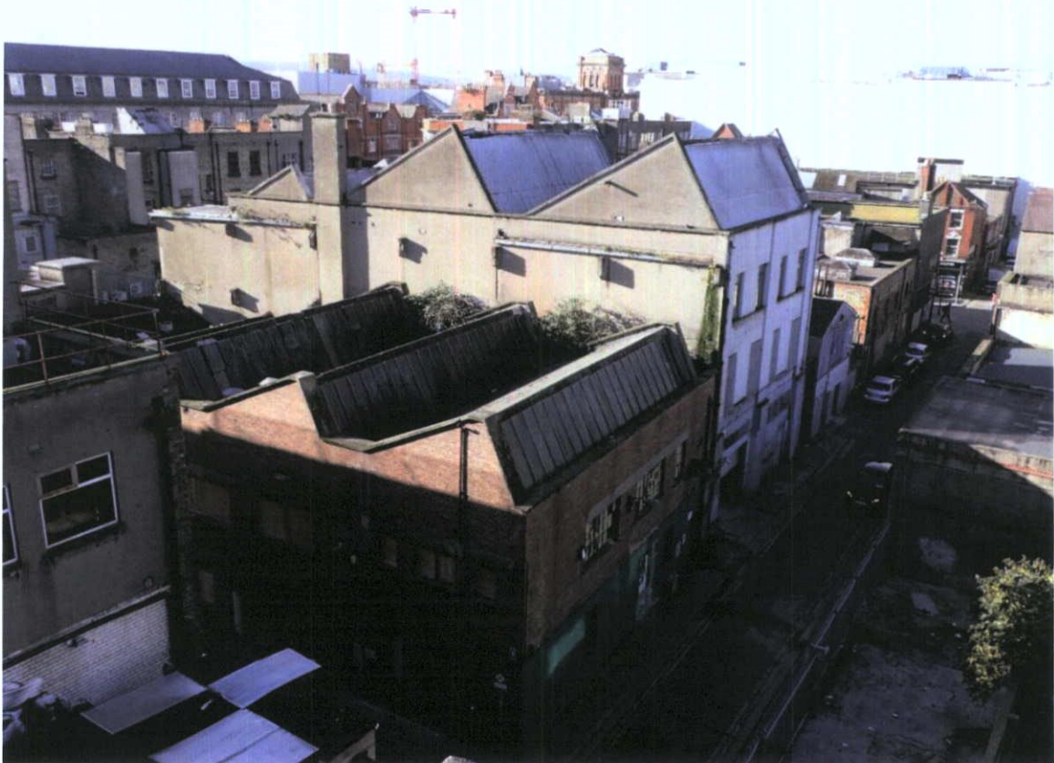
Fig.4.14.1: General view of the building showing a rendered and painted ground floor level, with a brick first floor rising to a sawtooth roof.
