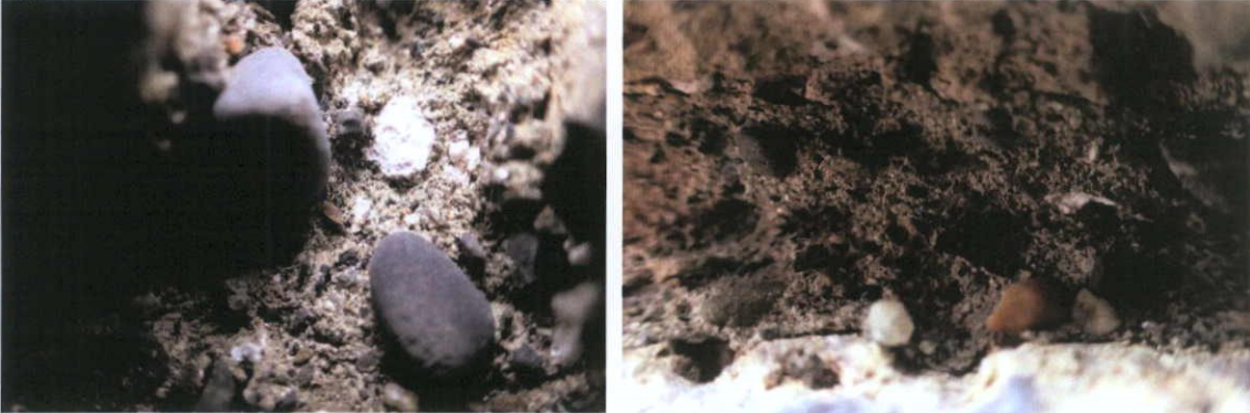
Fig. 4.17.7: Rounded limestone aggregate and sub-angular quartz with coarse burnt fuel fragments.
