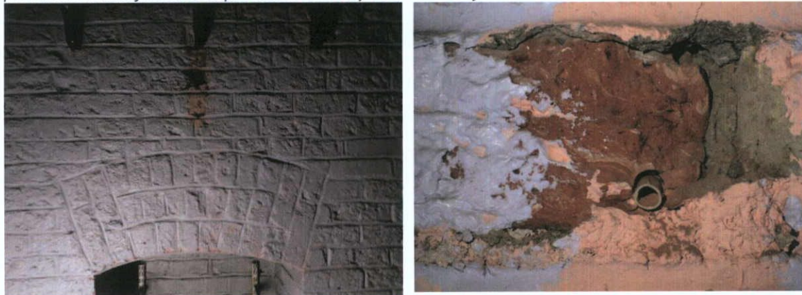
Fig. 4.17.12: The brick fireplace in the east wall at first floor level.
