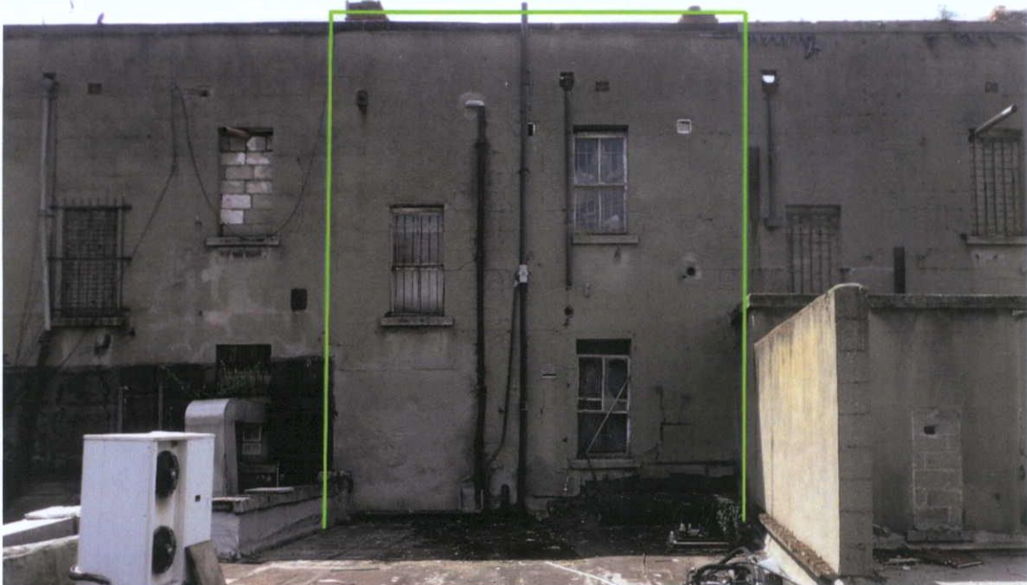
Fig.4.8.4: Note the rendered rear of No.4 mirrors the treatment of No.3 and 5.
