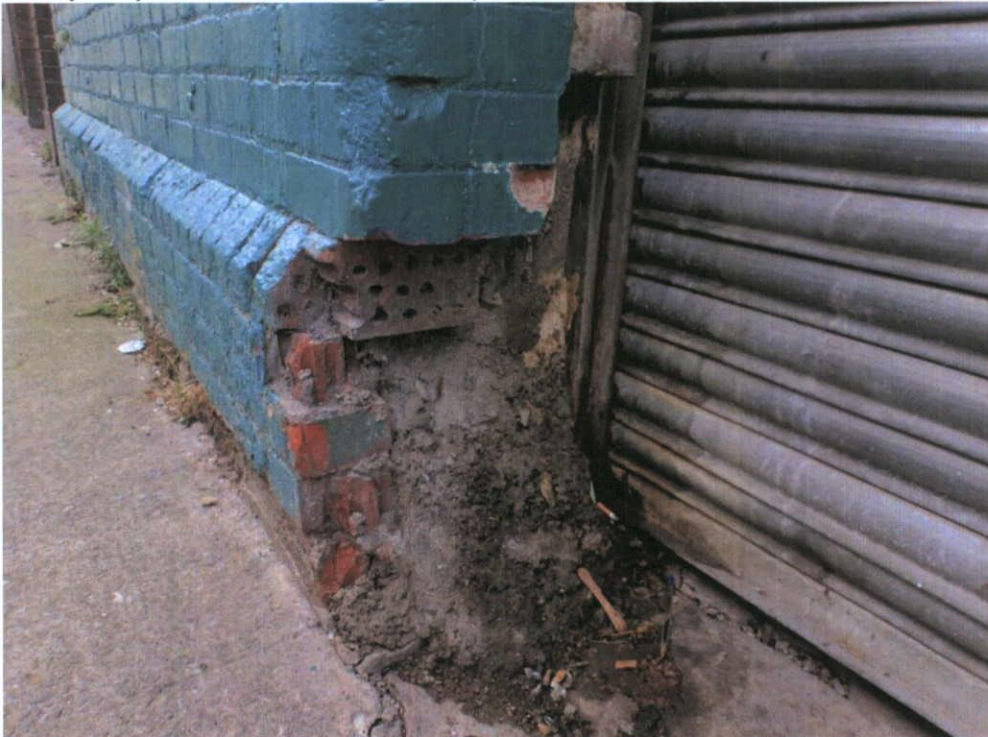
Fig.5.6.9: The south wall is of extruded brick and terracotta with yellow stock brick as internal wall linings, and is probably late nineteenth century construction work.
