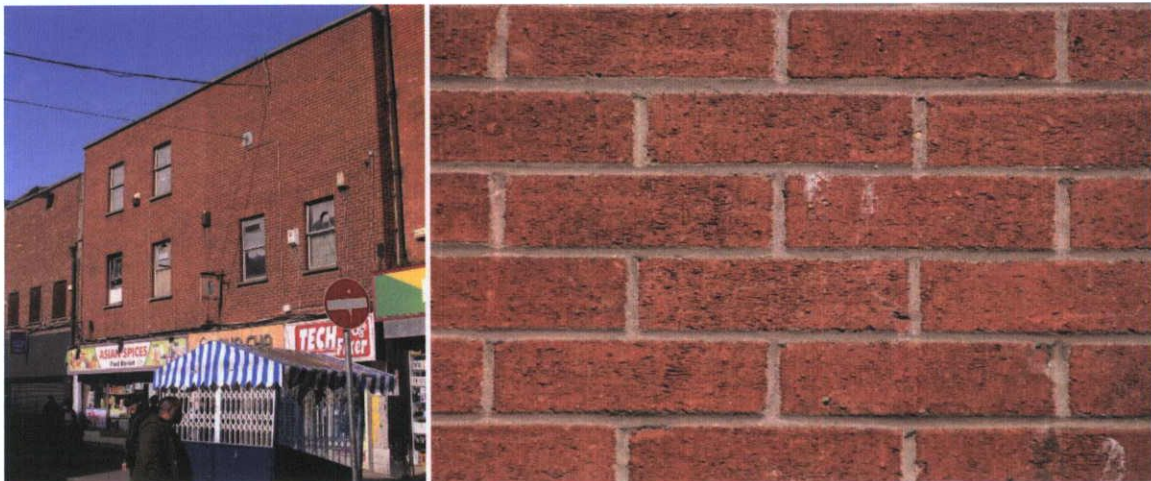
Fig.5.2.1: The façade of 11-12 Moore Street was built of machine-cut textured brick bedding in Portland Cement and finished with a 'bucket handle' joint, this finish is common from the late 1950s-1980s. The brick is widely used in the twentieth century, and this type of textured brick could date from anywhere from the 1930s to the 1990s.
