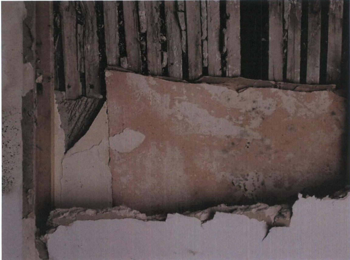
Fig.4.12.6: Lime lath-and-plaster ceiling surviving at the first floor of Nos.8-9 Moore Street (concealed behind poorly-applied later ceiling plaster layers).
