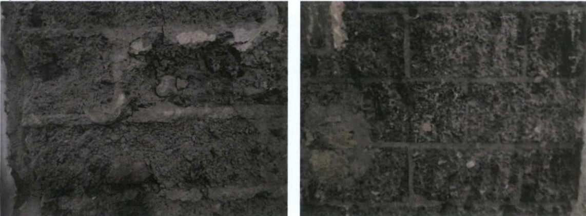
Fig.5.7.5: Concrete blockwork with natural stone, clinker and occasional iron fragments used to form the party wall with No.17 Moore Street, with a similar concrete block of smaller dimension used to form the rear wall of No.18 Moore Street.
