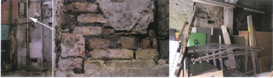
Fig.4.15.3: Exposed wall end at the junction of 5-8 and 9 Henry Place shows a mix of bricks in Portland Cement bedding mortars; internally, the limewash east wall at ground floor level is Calp limestone masonry, and consistent with 19 th century work.
