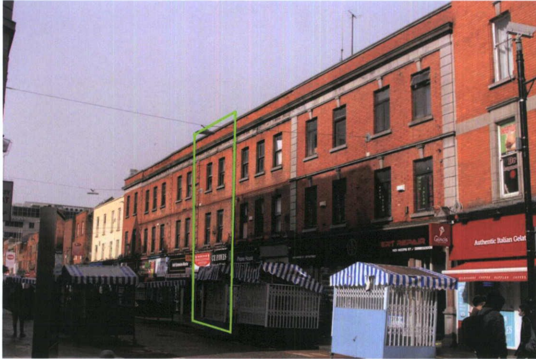
Fig.4.8.1: No.4 Moore Street, forming part of a terrace with Nos.3,5 and 6.
