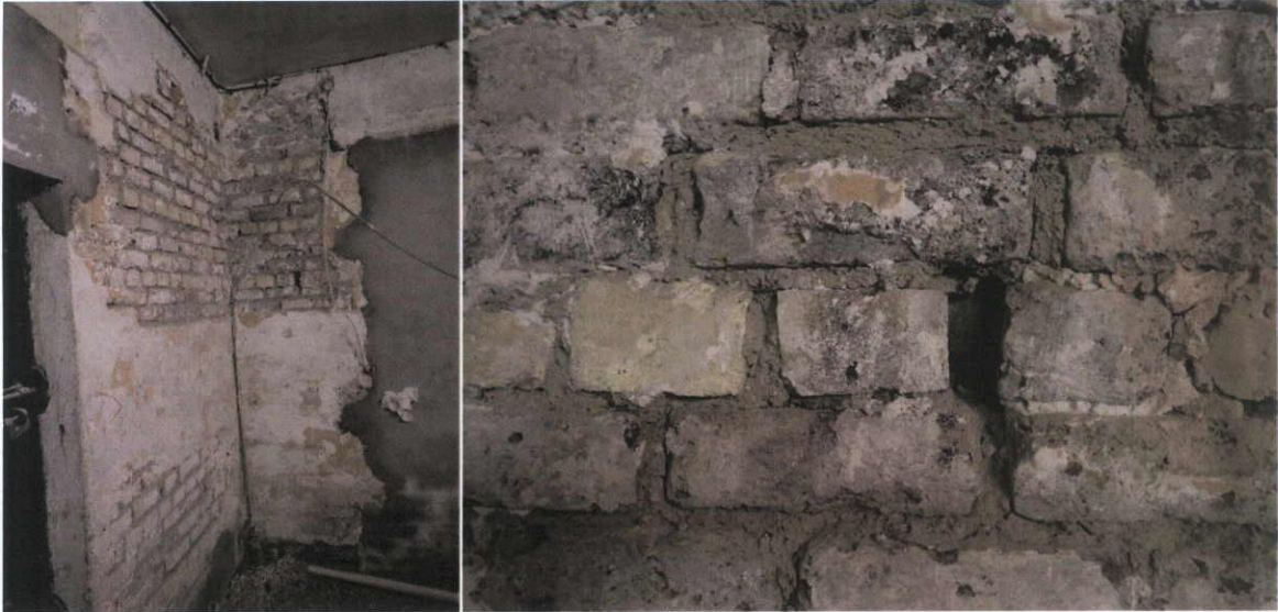
Fig.4.16.7: The north-east corner of the building formed of c.1920s yellow stock brick in a cementitious bedding mortar. There was no trace of any earlier brickwork in this part of the building.
