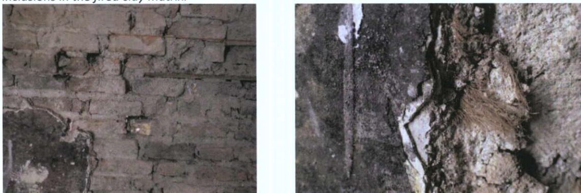
Fig.5.1.9: Internal face of the wall show in Fig.5.1.6 with a change in both brick and mortar at the 'creep hole' (left); while the surviving wall plaster has early haired lime plaster layers surviving beneath twentieth century surface finishes (right).
