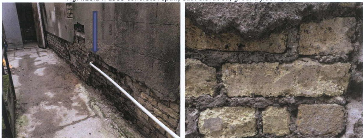
Fig.4.16.15: Junction (arrowed) between the c.1920 yellow stock brick in a cementitious bedding mortar and a section of probably nineteenth century stock brickwork in very poor condition.
