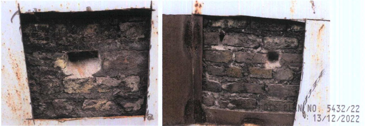
Fig.4.16.3: Nineteenth century yellow stock brick, first floor level, west elevation.
