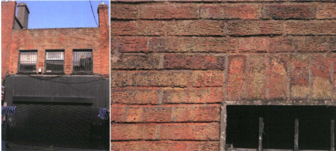
Fig.5.8.1: General view of 19 Moore Street with a detail of the painted brick at first floor level.
