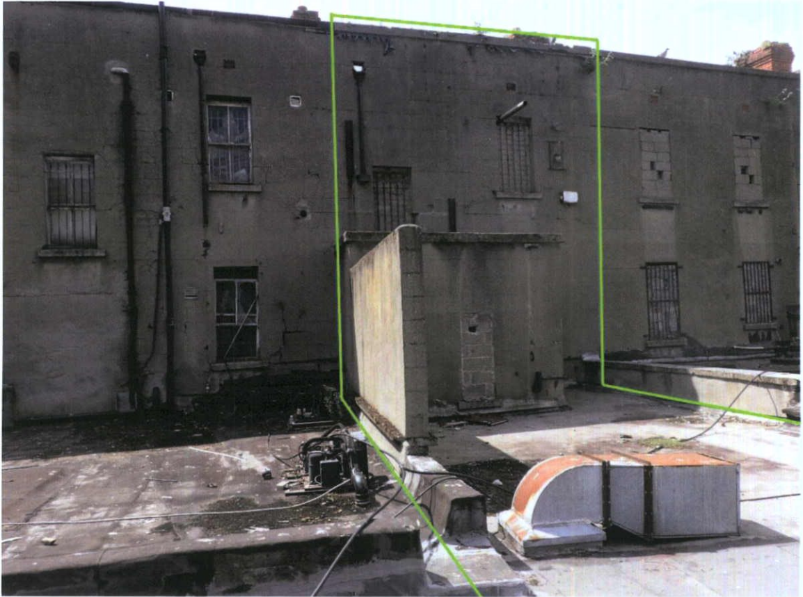
Fig.4.9.4: The rear elevation of No.5 Moore Street, built c.1917. Note that the colour and composition of the Portland Cement render and the configuration of the openings of Nos.5 and 4 matches; while the neighbouring No.6 Moore Street (right of image) was built using a slightly different Portland Cement render mix and with a different window arrangement.
