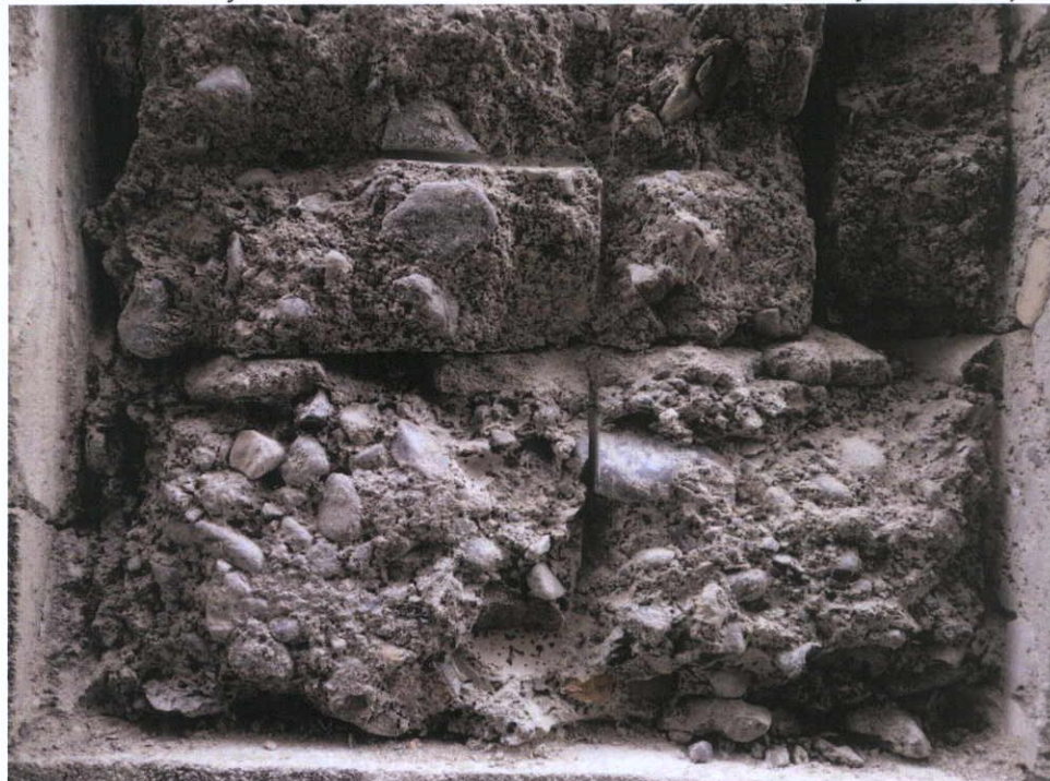
Fig.4.16.14: 1959 concrete repair, east elevation, ground floor level.
