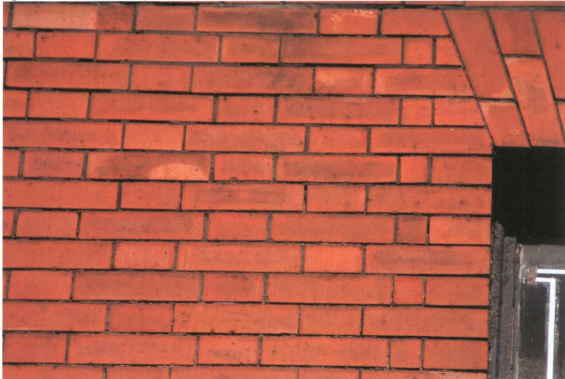
Fig.4.9.3: The surface of the brick shows subtle colour variations from the firing process.
