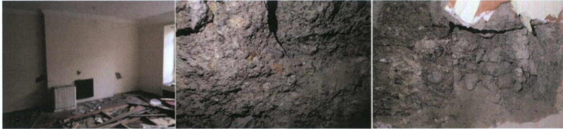
Fig.6.1.3: The south wall of the building (party wall with No.19 Moore Street) is of concrete construction.
