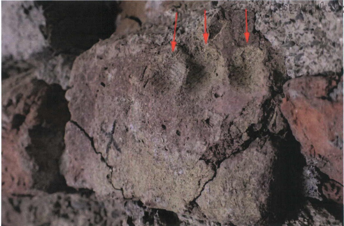
Fig.5.3.4: Fingerprint impression (probably from a child or young adolescent) formed in the brick. This occurs when the brick is 'green' and is turned prior to firing.
