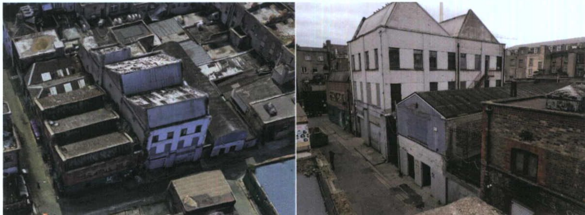
Fig.4.15.1: General view of No.9 Henry Place.
