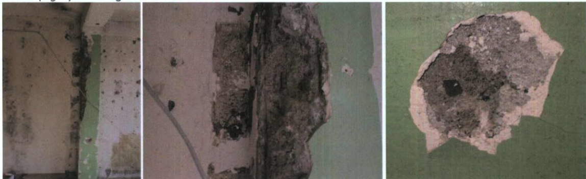
Fig.5.8.4: The party wall (left) and inner face of the west wall (right) are of concrete.
