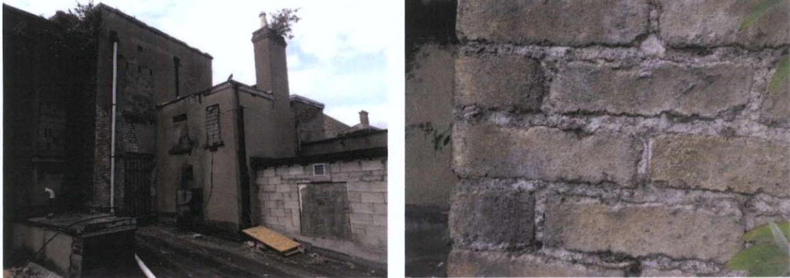
Fig.4.11.3: General view of the rear of No.7 Moore Street, which extends further than the terrace immediately to the south, and was constructed using a yellow stock brick (normally concealed beneath a Portland Cement render).
