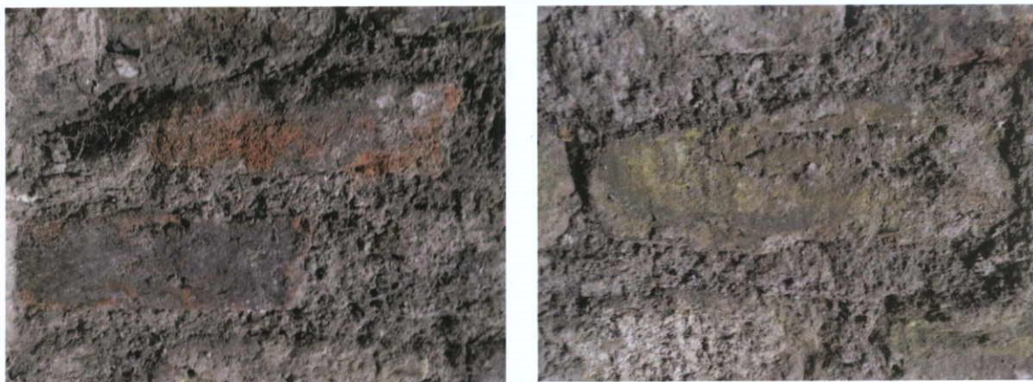
Fig.4.12.5: Red and yellow stock brick, internal wall lining, north wall, 9 Henry Place.
