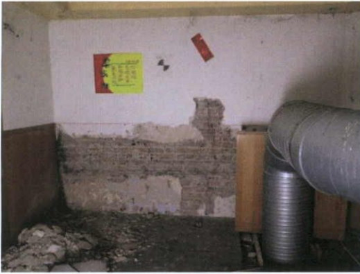
Fig.5.1.10: The party wall between Nos.10 and 11 Moore Street contains early brickwork with lime mortars struck in the same style as the internal walls of the mid-eighteenth century No.42 O'Connell Street.
