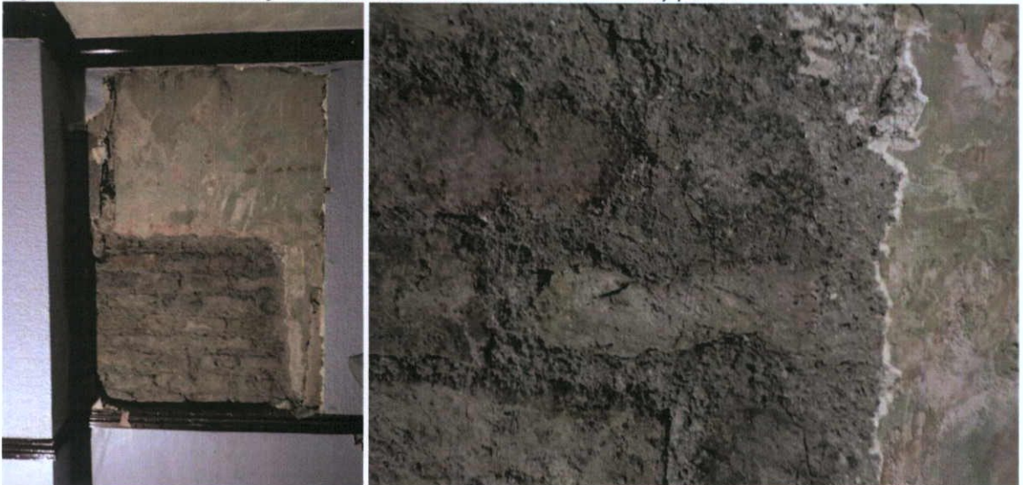
Fig.4.12.3: Yellow and red stock brick bedded in thick lime bedding mortars on the internal face of the north wall of No.9 Henry Street.
