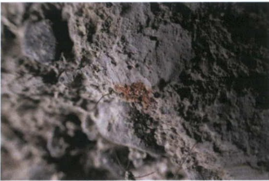
Fig.5.1.11: The bedding mortars of the party wall contains sub-rounded limestone aggregate and brick pozzolan (left); while the lime plasters on the wall have clumps of animal hair (right).
