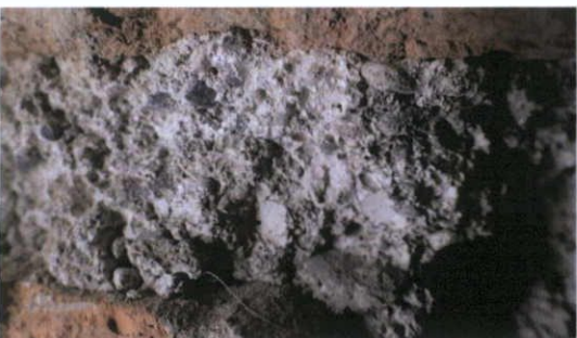
Fig.5.1.13: Poorly sorted bedding mortar containing limestone, chert and quartz aggregate.
