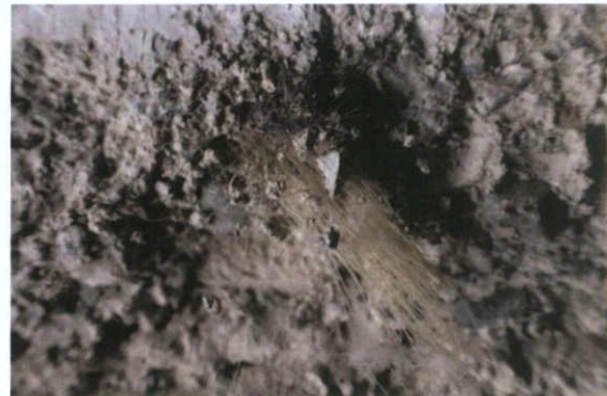
Fig.5.1.11: The bedding mortars of the party wall contains sub-rounded limestone aggregate and brick pozzolan (left); while the lime plasters on the wall have clumps of animal hair (right).
