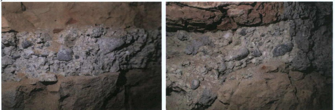
Fig.6.1.5: The lime mortar joints bedding the hand-made clamp-fired brick consist mainly of sub-rounded limestone aggregate with scarce angular lime lumps.
