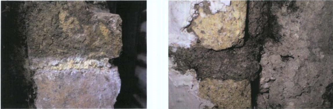
Fig.5.6.8: Detail of yellow stock brick from the inner face of the south wall bedded in a lime-rich mortar; and the inner face of the east wall showing coarse yellow brick bedded in a cement mortar (right).
