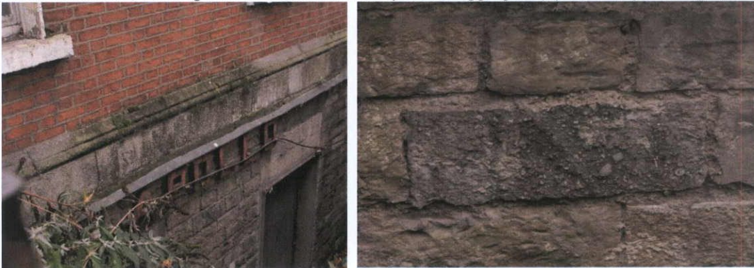
Fig.4.3.5: The basement level is separated from the brick superstructure by a moulded granite strong course, with the well-cut Calp limestone face of the basement wall laid in a coarse-grained lime mortar. One large limestone block is coarsely fossiliferous and may be Ardbraccan limestone.
