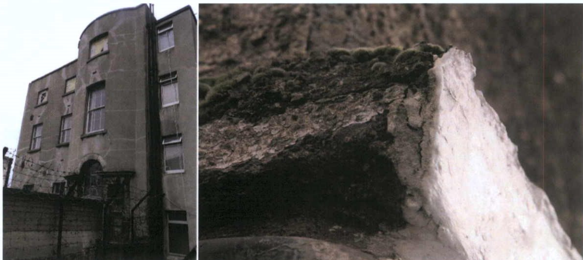
Fig.4.3.13: The rear retains a tripartite arched window in the curving bay, mirroring the treatment of the main door. The rear has been re-rendered throughout in a Portland Cement-based mortar.
