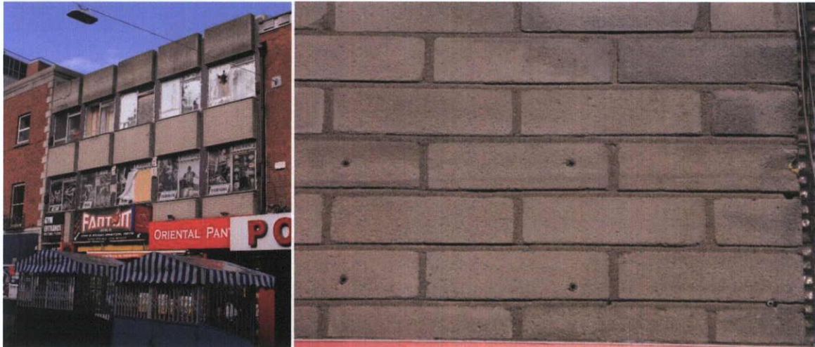
Fig.6.2.2: Detail of the concrete brick on the façade.
