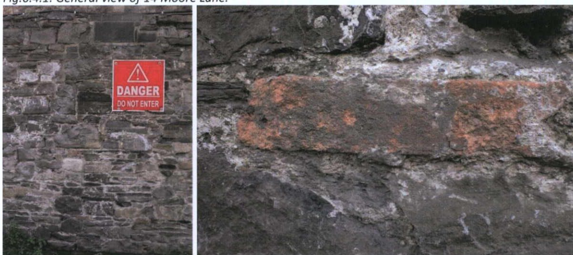
Fig.6.4.2: Calp limestone masonry section with thin brick forming part of the fabric. Note that the masonry contains flaggy and rounded stones. The masonry is similar to the Calp limestone masonry forming the internal east wall at 9 Henry Place (probably the remnants of a nineteenth century stable).
