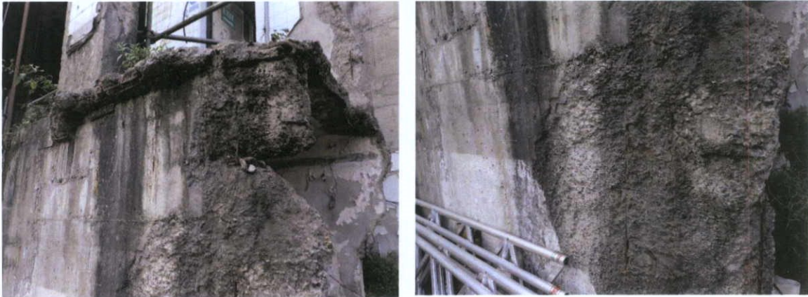
Fig.4.2.5: Detail of reinforced concrete structure on the north side of the site.
