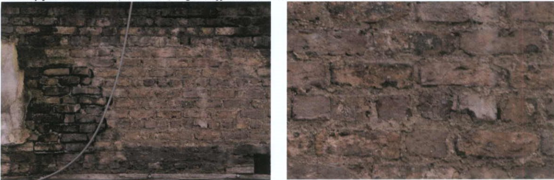
Fig.5.3.25: Yellow stock brick in lime bedding mortar.
