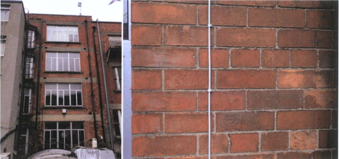
Fig.5.1.2: The rear is composed of machine-cut red brick laid in English garden bond with a lime-cement mortar and having concrete courses above the window openings.
