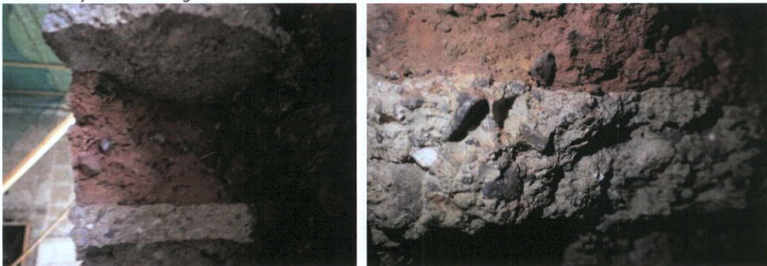
Fig.4.3.10: The large aggregate in the coarse-grained bedding mortars is similar in shape, dimension and mineralogical composition to the stone inclusions seen in the handmade bricks – suggesting a similar source. This is probably brick from the Moore Street brickfield.
