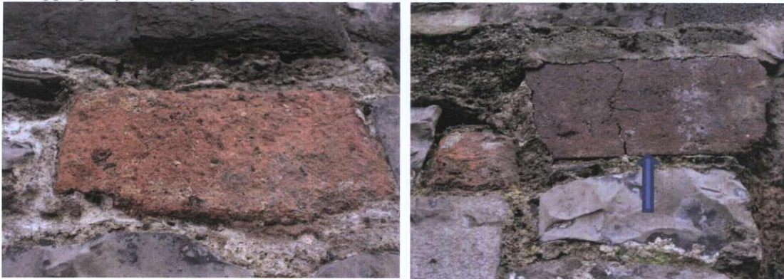
Fig.8.4.9: Warped hand-made clamp fired brick (left) while the upper course contain occasional imported brick (right, arrowed) presumably added as a levelling-up course before the concrete was poured).
