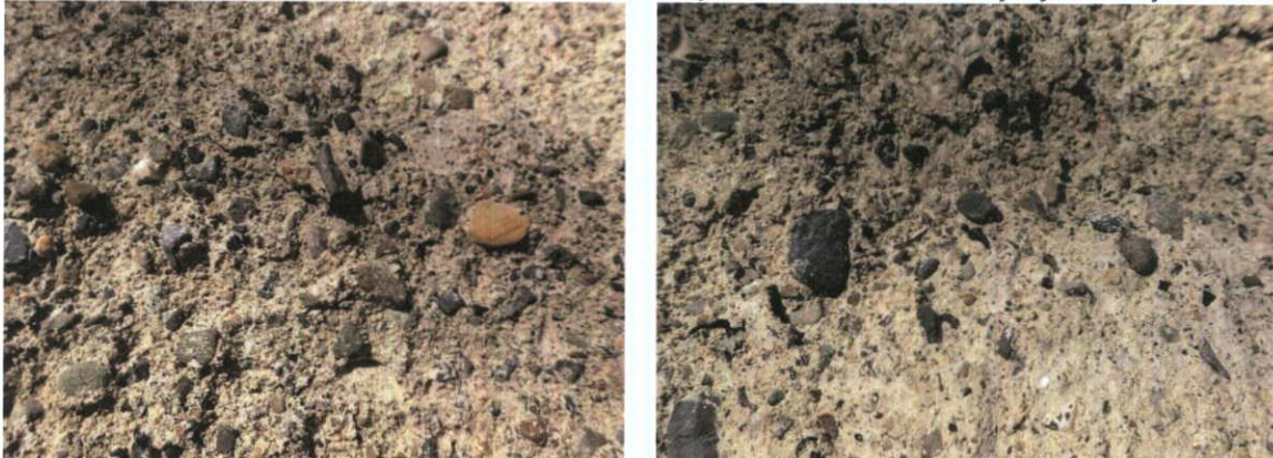
Fig.5.3.6: Detail of the mortar showing rounded limestone, quartz, greywacke and other lithic aggregate.
