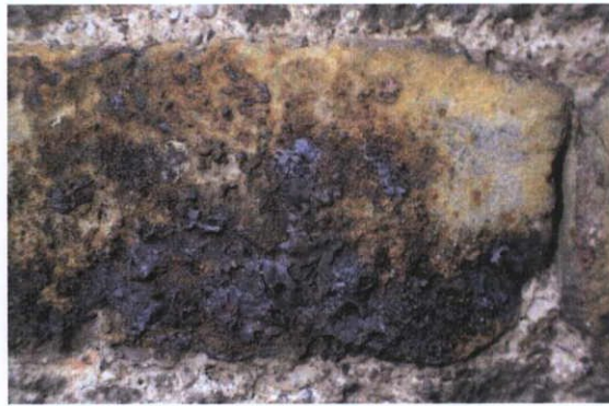
Fig.4.4.5: Overburnt clamp-fired yellow stock brick showing calcined stone and vitrified zones.
