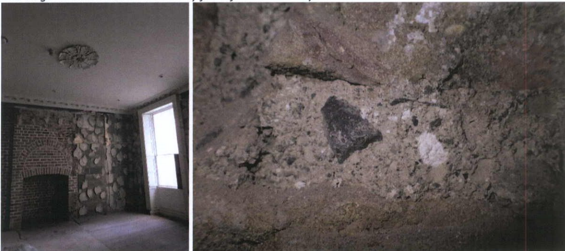
Fig.4.3.6: The ground floor shows later alterations, but the party wall shows place brick laid in a coarse-grained lime bedding mortar with poorly sorted limestone, quartz and chert aggregate and large lime lumps.
