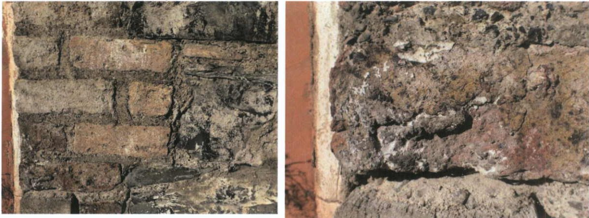
Fig.5.3.14: The chimney breast is edged by irregular clamp-fired brick.
