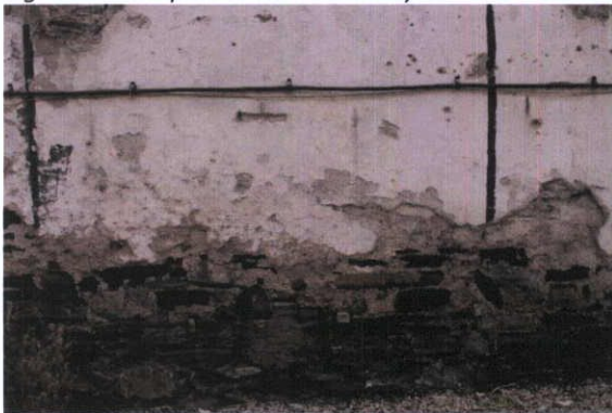
Fig.5.3.29: Detail of the plaster showing brick pozzolan and animal hair. The fine brick dust (& saturation) has contributed to the pinkish hue of this section of the mortar.
