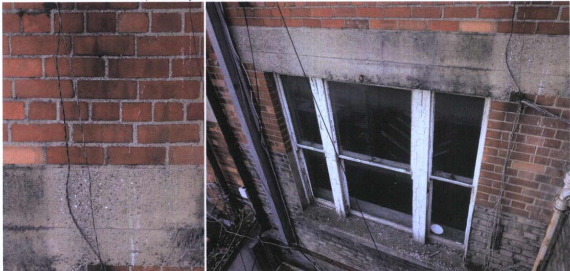
Fig.5.2.2: Detail of the 1920s machine-cut brick and concrete lintel of the superstructure, above yellow stock brick at the rear basement level.
