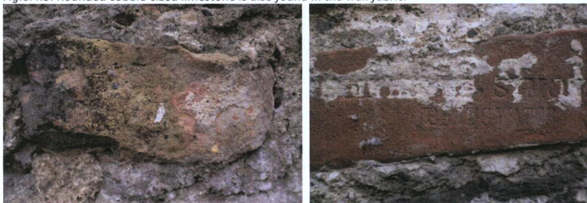
Fig.6.4.4: Irregular distorted clamp-fired vitrified yellow brick, possibly 18 th century (left) and imported stamped 'Colhurst Symon & Co. Ltd Bridgwater' from Somerset. This brickmaker was in operation from 1857 until the 1960s
