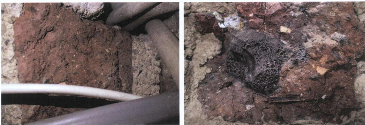
Fig.9.1.1: Brick with coarse angular limestone inclusions from the basement of No.43 O’Connell Street (left), and seen in the internal walls of No.71 Parnell Street (right).
