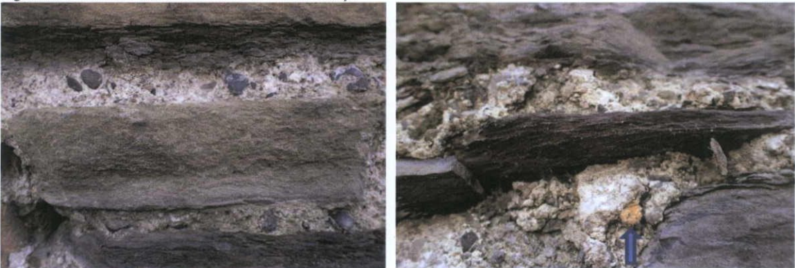
Fig.6.4.5: Deep lime mortar joints with poorly sorted predominantly coarse limestone aggregate, slate pinnings and scarce coarse brick aggregate (arrowed).
