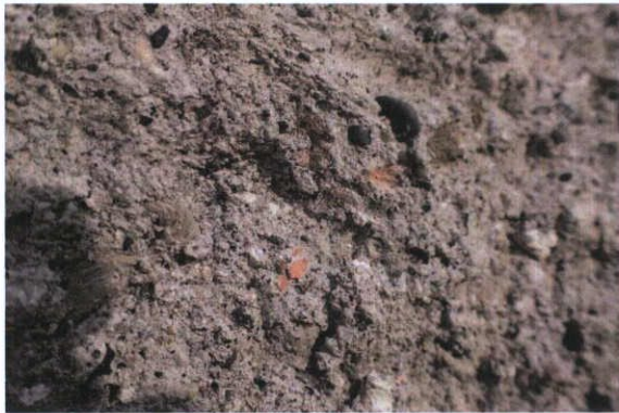
Fig.5.3.30: Detail of the surface of the exposed plaster showing limestone aggregate, occasional burnt fuel fragments, clumps of animal hair added to improve mechanical strength (but with poor craftsmanship as the hair is not teased through) and crushed brick (porous aggregate) and fine brick dust.
