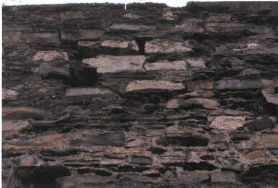
Fig.5.3.28: Calp limestone masonry.
