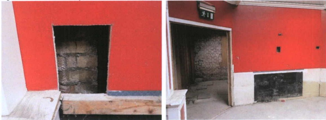
Fig.4.4.2: The brickwork is covered by modern plasterboard.
