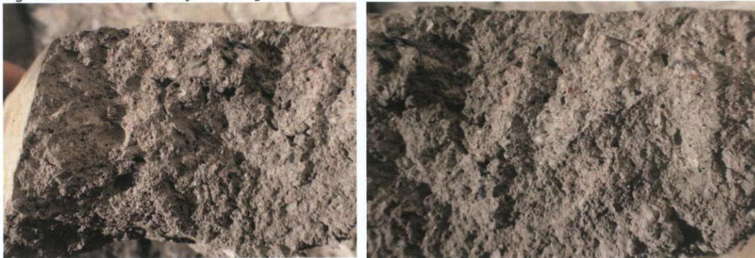
Fig.5.3.8: Cross-section of plaster from the niches.
