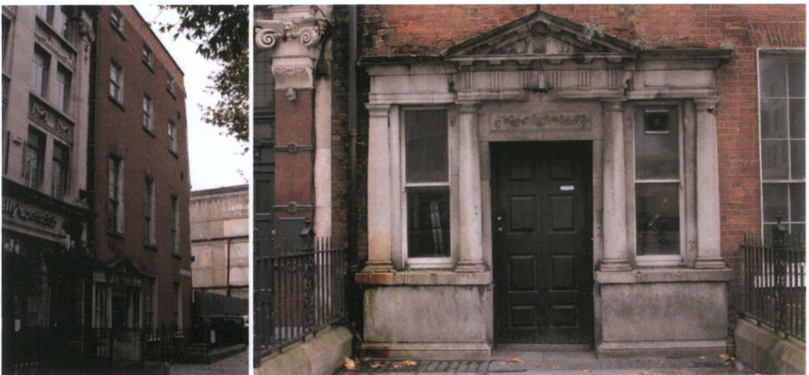
Fig.4.3.1: Four-storey-over-basement façade with parapet in later brick, with railings on a granite plinth enclosing the basement well; and a tripartite Neo-Classical doorway of imported English limestone.
