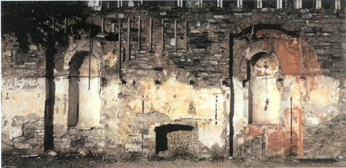
Fig.5.3.7: General view of 'Building B'.
