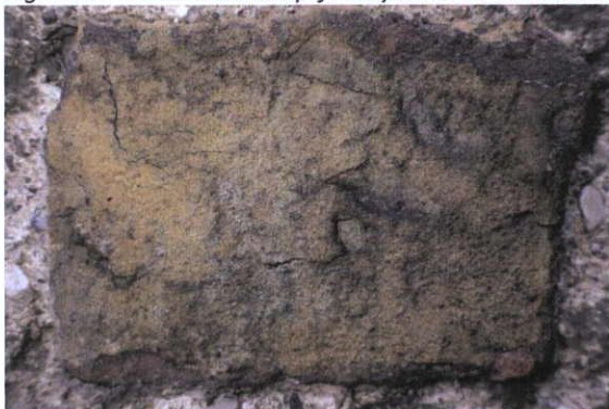
Fig.4.4.6: Clamp-fired yellow stock brick showing shrinkage cracks and over-burnt edges; laid in a coarse-grained lime mortar of rounded limestone pebbles with angular chert and quartzite and crushed brick pozzolan added.
