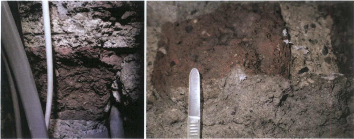
Fig.5.1.8: The coarse-grained lime bedding joints are horizontally struck joints. The lime mortar contains limestone, quartz, chert and lime limps. The clamp-fired brick is similar to that seen in No.42. The mortar and clamp-fired brick contain similar aggregate (morphology, size range and mineralogy) suggesting a similar source of raw materials. This is probably brick from the Moore Street brickfields.
