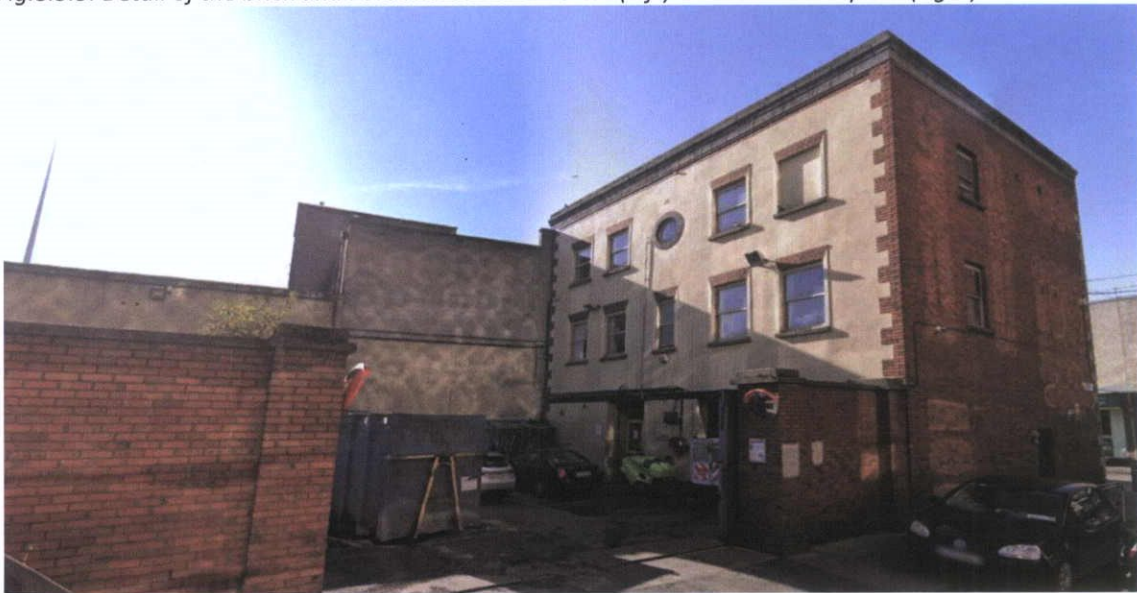
Fig.8.3.4: View of the north elevation and rear from Rahilly Parade.
