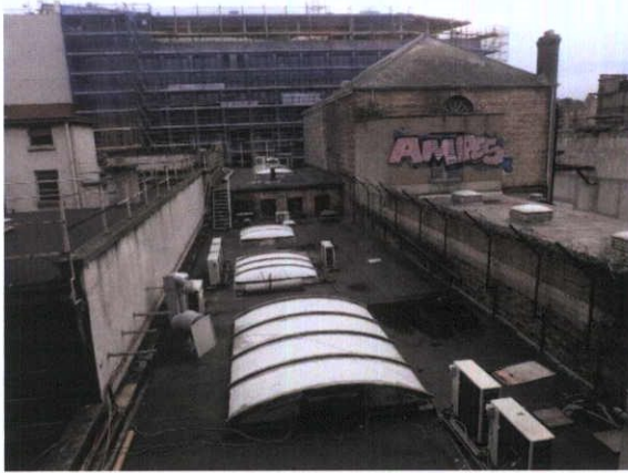
Fig.4.4.4: The boundary wall with No.43 O'Connell Street is formed of clamp-fired yellow stock brick and likely to be of nineteenth century date.
