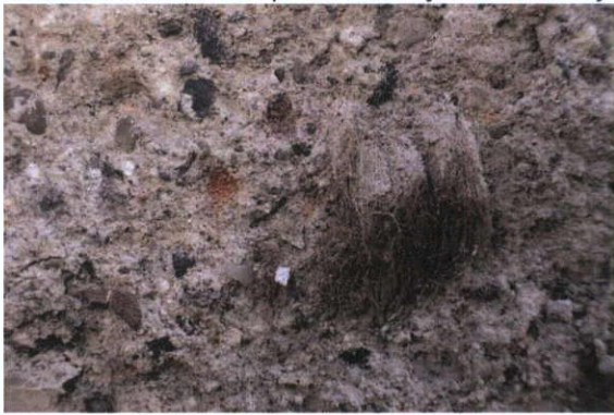
Fig.5.3.30: Detail of the surface of the exposed plaster showing limestone aggregate, occasional burnt fuel fragments, clumps of animal hair added to improve mechanical strength (but with poor craftsmanship as the hair is not teased through) and crushed brick (porous aggregate) and fine brick dust.
