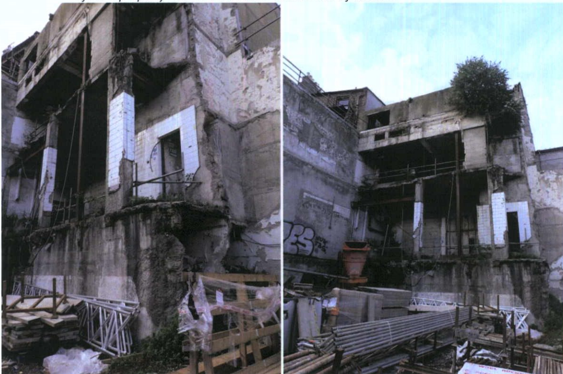
Fig.4.2.4: Reinforced concrete structures on the north side of the vacant lot.
