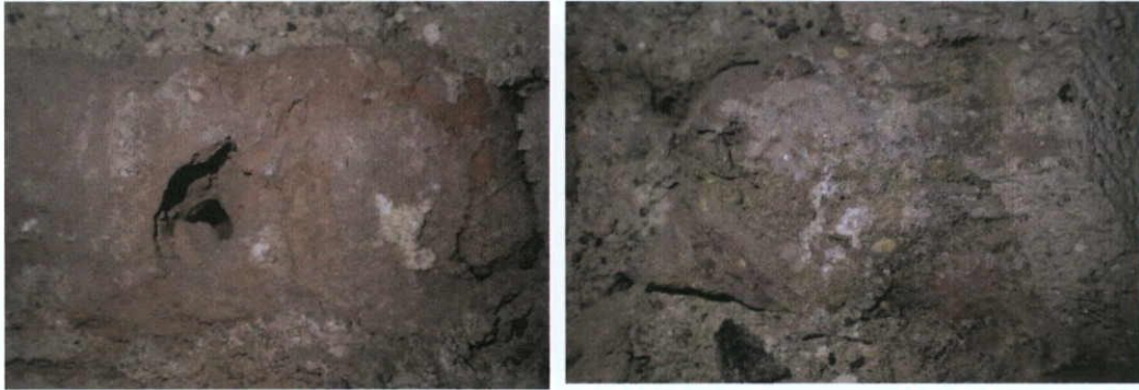
Fig.4.3.7: Place bricks in a coarse-grained lime bedding mortar. Internal walls at first floor level.
