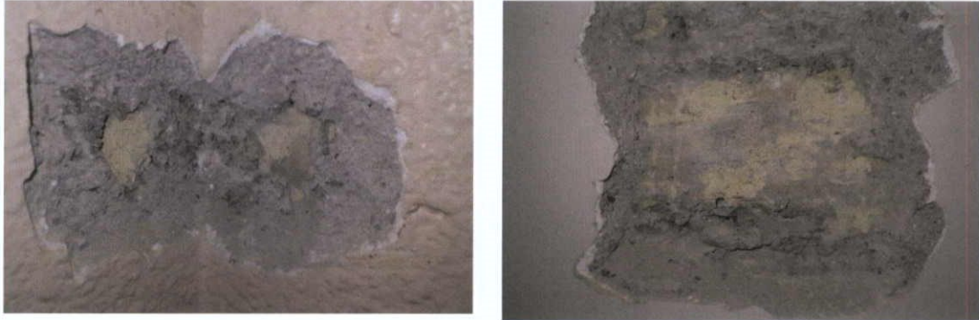
Fig.5.2.14: 1920s yellow stock brick in cementitious mortar exposed in the party walls of the south (left) and west (rear) walls of the first floor level.
