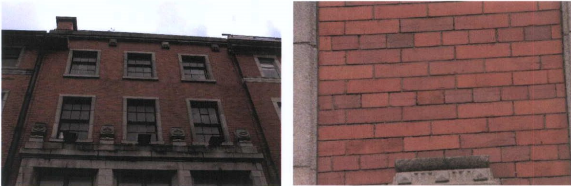
Fig.5.4.1: Brickwork at the façade of 57 O’Connell Street.
