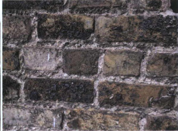
Fig.4.4.4: The boundary wall with No.43 O'Connell Street is formed of clamp-fired yellow stock brick and likely to be of nineteenth century date.
