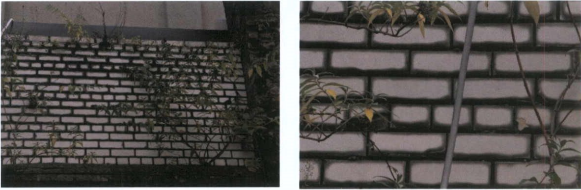
Fig.5.3.24: White glazed 'encaustic' brick which became popular towards the end of the 19 th and early 20 th century for bathrooms, kitchens, high traffic areas and some rear elevations.
