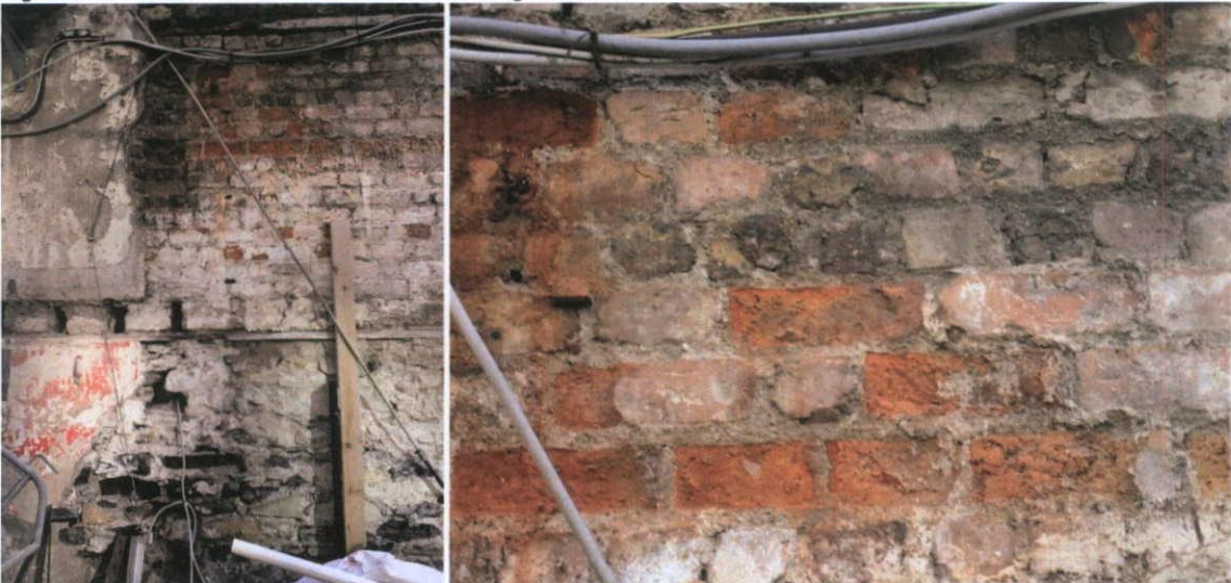
Fig.5.3.26: The red stock brick, in poor condition with the fireskin lost in many places, and the lower section of Calp limestone masonry also visible (left, bottom).
