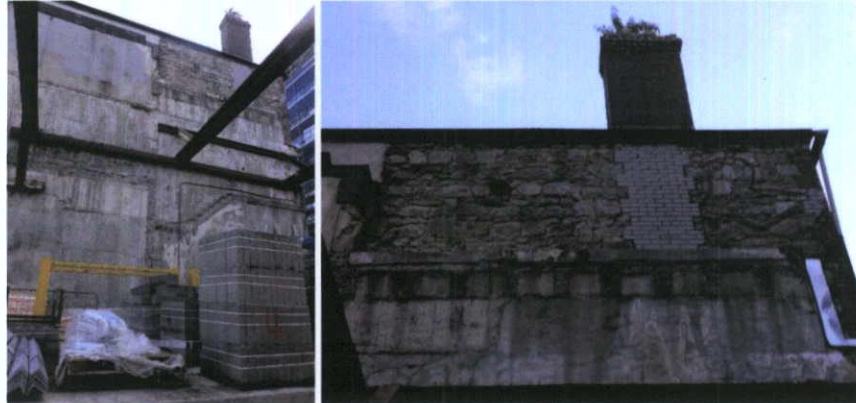
Fig.4.2.3: Reinforced concrete on the south side, with historic masonry of the adjacent property visible at the south-west corner of the site.
