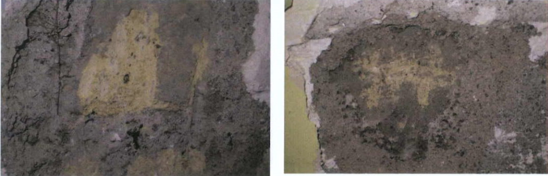
Fig.5.2.13: 1920s yellow stock brick in cementitious mortar exposed in the party walls of the north (left) and east (façade) walls of the first floor level.
