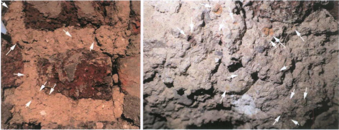
Fig.4.1.4: Brick pozzolan (arrowed) was added to the mortar. This imparts hydraulic qualities to the mortar, while the larger brick fragments also function as porous aggregate. The mortars commonly show relatively coarse 'lime lumps'.
