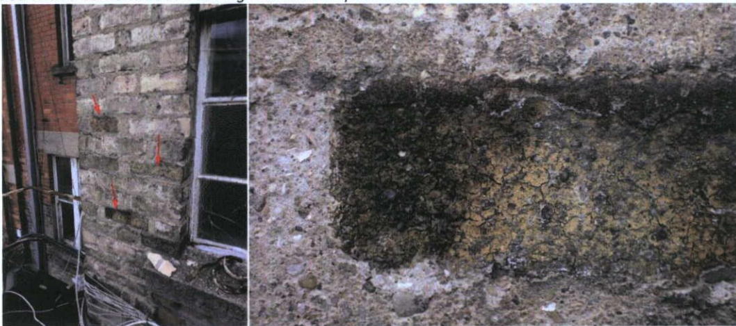
Fig.5.2.10: Salvaged earlier clamp-fired yellow stock brick in the return.
