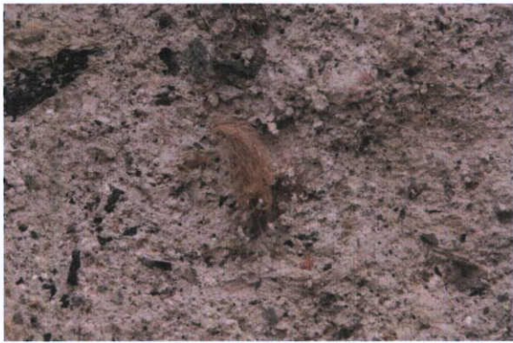
Fig.5.3.29: Detail of the plaster showing brick pozzolan and animal hair. The fine brick dust (& saturation) has contributed to the pinkish hue of this section of the mortar.
