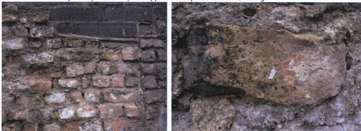
Fig.8.4.11: Poorly formed hand-made place brick, with modern concrete construction adjacent.
