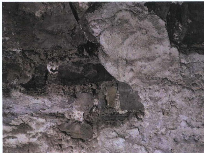
Fig.5.2.3: Dublin Calp limestone at basement level with single-coat lime plaster and multiple coats of limewash.
