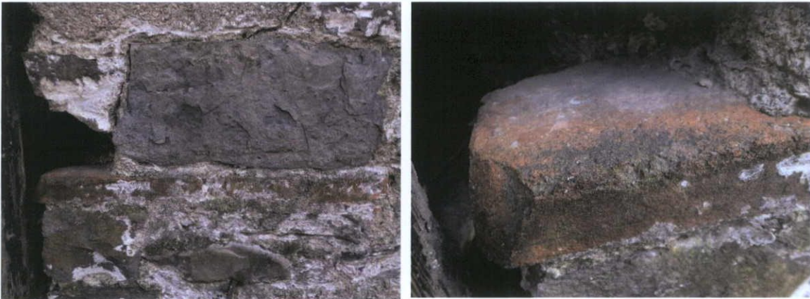
Fig.6.4.6: Ceramic tile used within the masonry.
