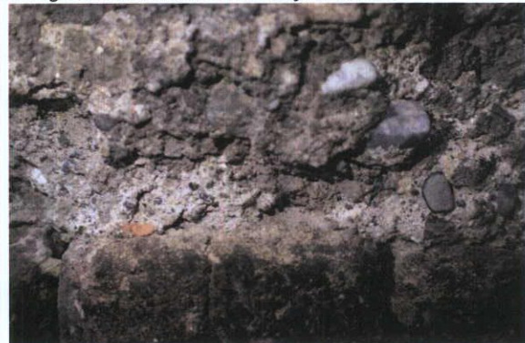
Fig.4.4.6: Clamp-fired yellow stock brick showing shrinkage cracks and over-burnt edges; laid in a coarse-grained lime mortar of rounded limestone pebbles with angular chert and quartzite and crushed brick pozzolan added.
