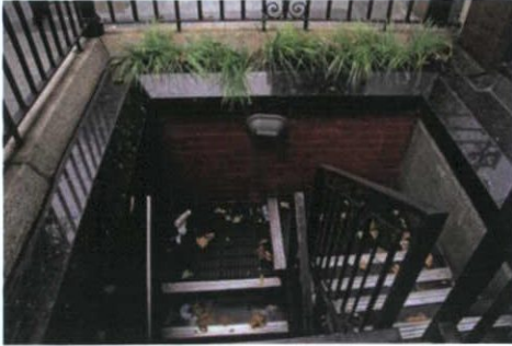
Plate 10: B-1 – View south into basement well
