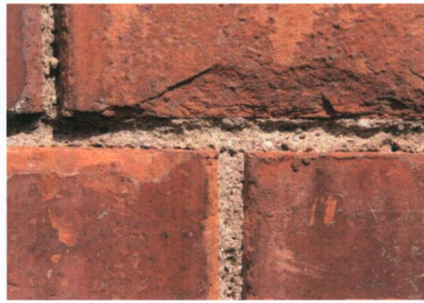
Fig.5.5.6: Perforated red brick used for flatwork and rounded corners.
