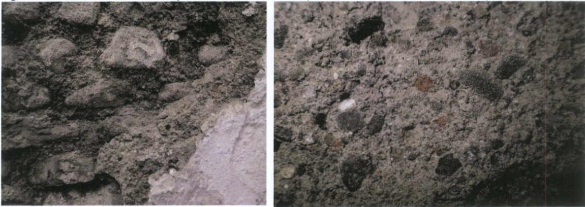
Fig.5.7.6: The south wall of the basement well is formed from Calp limestone masonry, many of which consist of rounded and sub-rounded cobbles which are indicative of Georgian building. The lime render laid on top of the wall is in poor condition; but contains poorly-sorted predominantly limestone aggregate with large coarse lime lumps and crushed brick and brick dust pozzolan.
