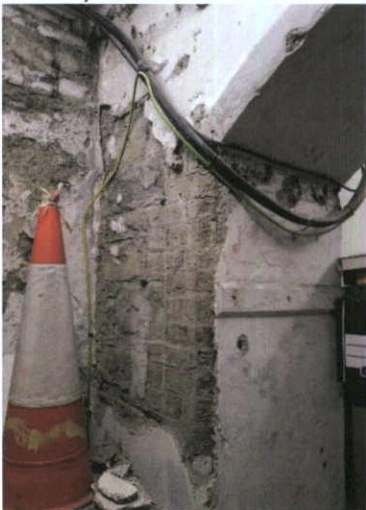
Fig.5.7.4: Detail of a mid-nineteenth century brick arch at basement level of No.60, with sharp limestone sand and coarse lime lumps in the bedding mortar (beneath the Portland Cement pointing).
