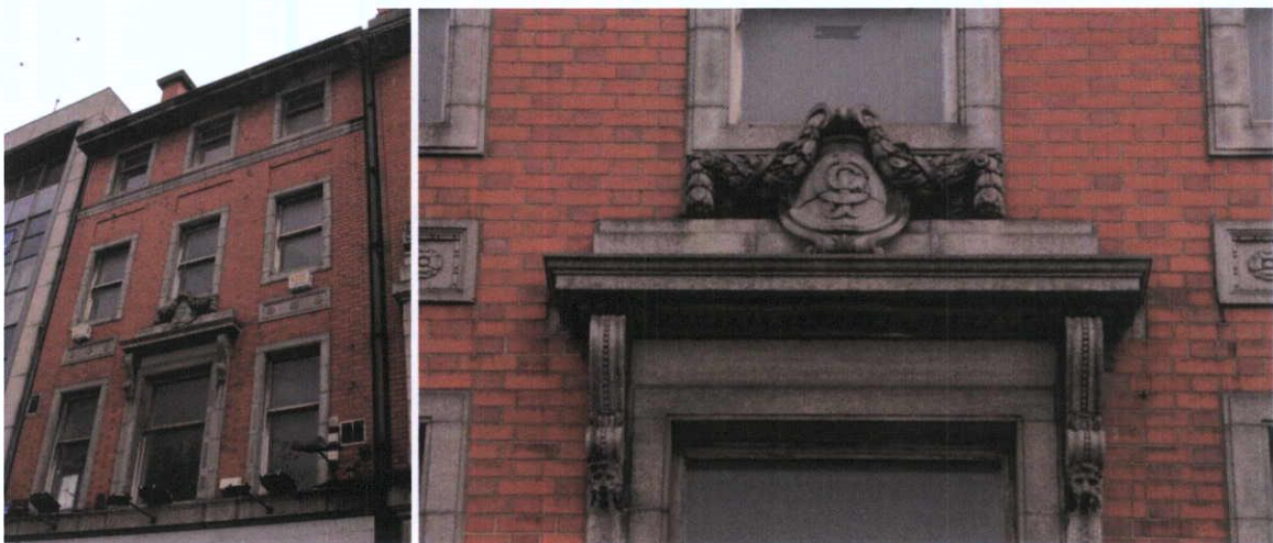
Fig.5.5.1: Granite and brick at the façade.
