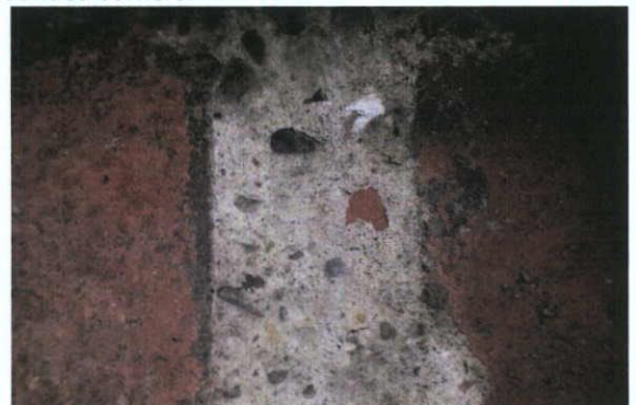
Fig.5.5.7: Brick stamped 'Davison' (left) and detail of the mortar mix containing poorly sorted sub-angular limestone as well as crushed red and yellow brick pozzolan. Charles Davison's Ewloe Barn Brick and Tile Works were active from 1933 to 1951 at Buckley in Flintshire, Wales 2 .
