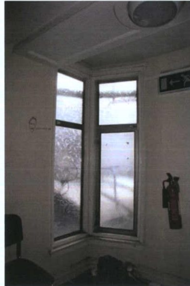
Plate 71: F-5 – View to south-west
