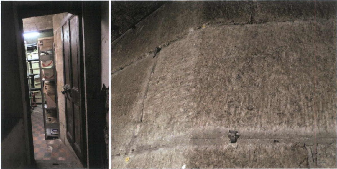
Fig.5.7.10: The strong room is lined with granite laid in a lime putty mortar, and pointed with a Portland Cement-based mortar with an incised line.
