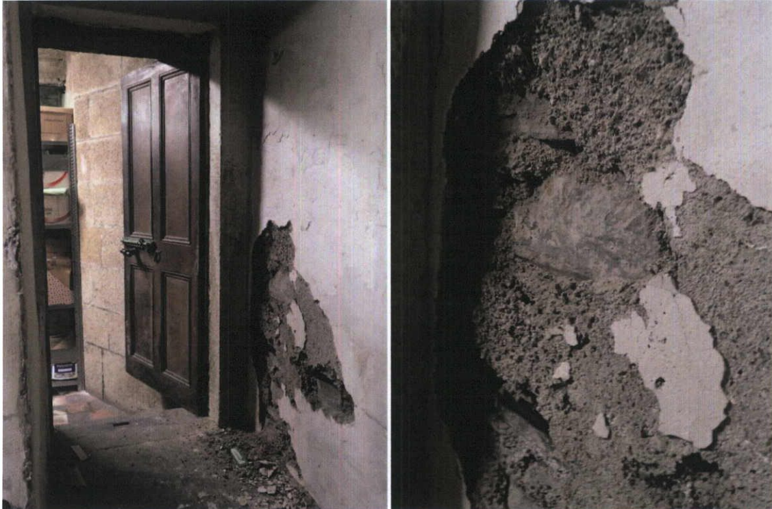
Fig.5.7.8: Detail of the entrance to the granite-lined strongroom at the rear of the building, and the Calp limestone masonry forming the north wall at basement level (right).
