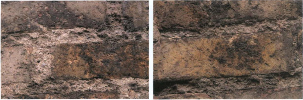
Fig.5.4.5: Clamp-fired yellow stock brick from the north window.
