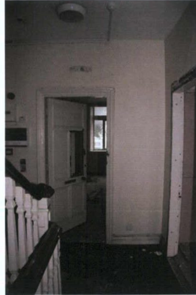
Plate 75: F-5 – View to east
