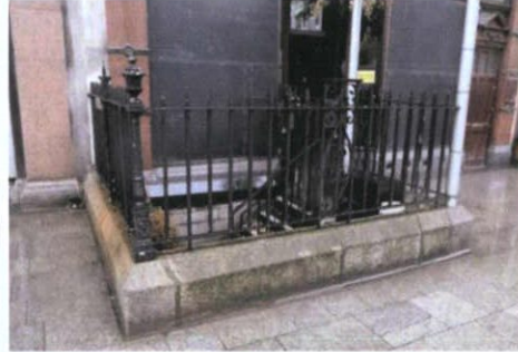
Plate 11: Railings to basement well
