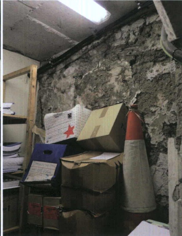
Fig.5.7.3: View of a brick pier at the front of the property at basement level, with a rendered Calp limestone masonry wall.
