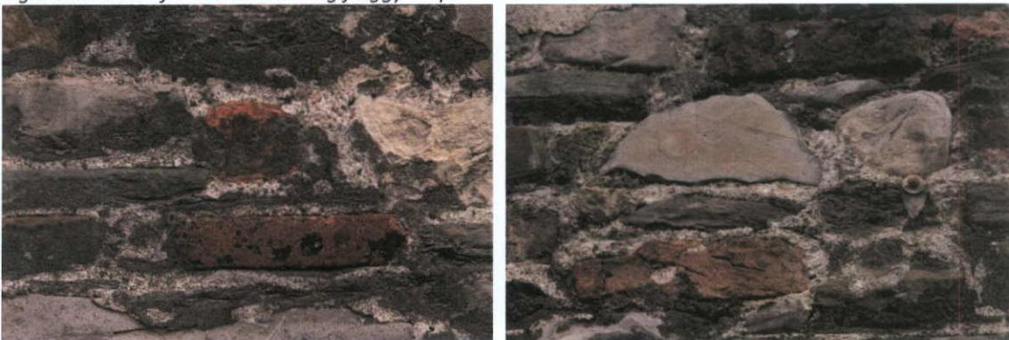
Fig.5.6.3: Thin irregular probably Georgian brick.
