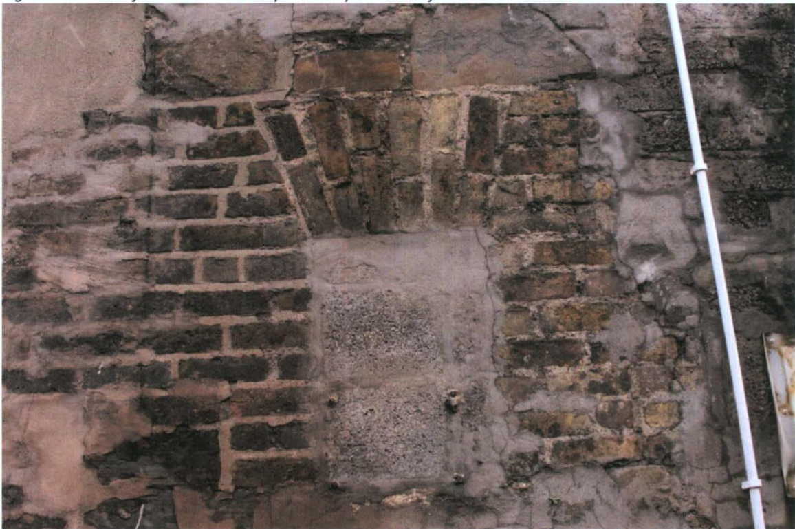
Fig.5.4.4: Detail of the yellow stock brick window.
