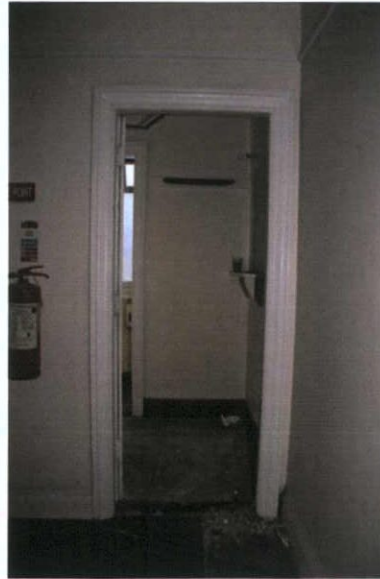
Plate 91: S-1 – View to west towards Room S-2
