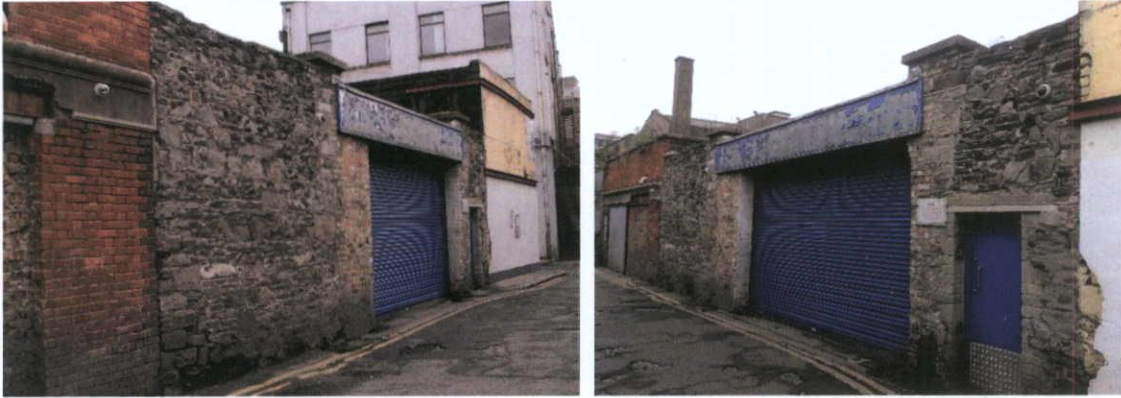
Fig.5.6.1: General view of the Calp limestone masonry wall at the rear of No.59 O'Connell St.
