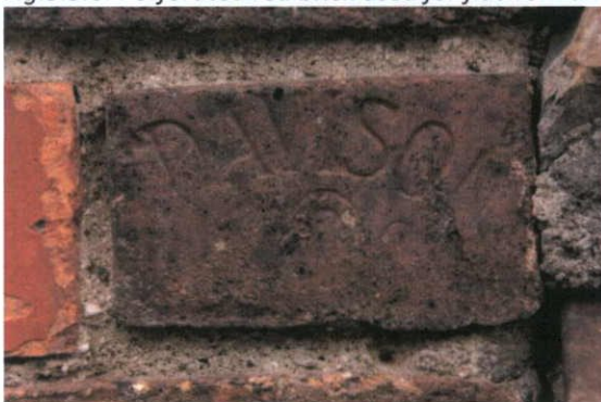
Fig.5.5.7: Brick stamped 'Davison' (left) and detail of the mortar mix containing poorly sorted sub-angular limestone as well as crushed red and yellow brick pozzolan. Charles Davison's Ewloe Barn Brick and Tile Works were active from 1933 to 1951 at Buckley in Flintshire, Wales 2 .
