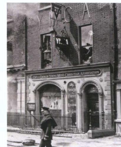
Figure 3: Damage to 43 Sackville Street Upper from fighting in July 1922 (National Library of Ireland)
