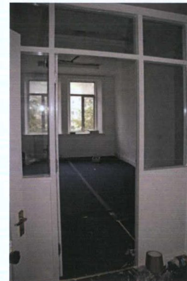
Plate 96: S-3 – View into Room S-4
