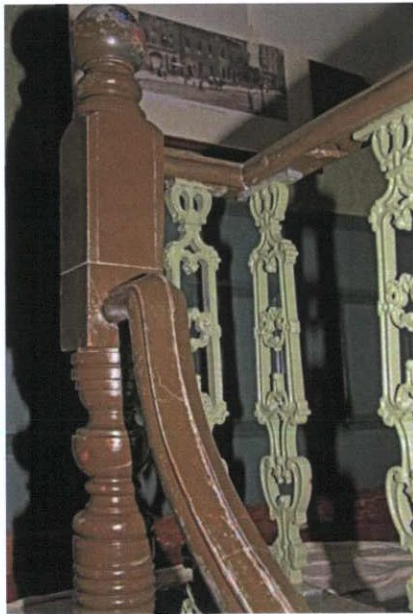
Plate 58: F-1 – Newel post and cast-iron balusters
