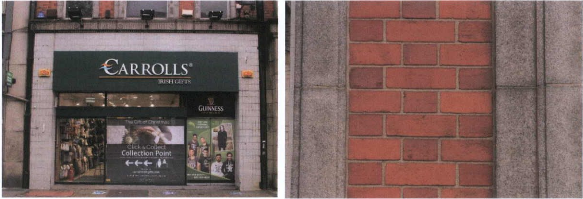
Fig.5.5.2: Modern shopfront with earlier granite course above (left); and a detail showing kiln-fired c.1920s brick in flush mortar joints (right).
