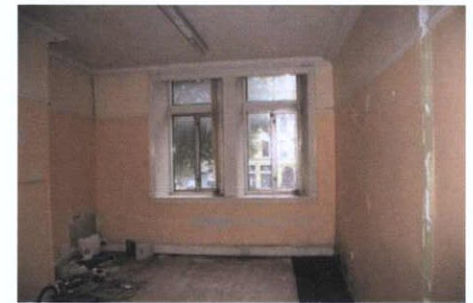
Plate 85: F-9 – View to east
