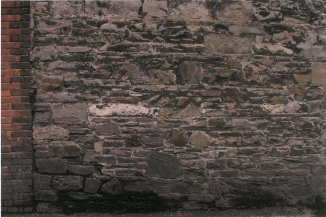
Fig.5.6.2: View of the wall showing flaggy Calp.
