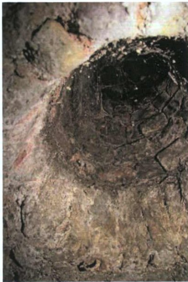
Plate 37: B-9 – Coal hole access to ceiling
