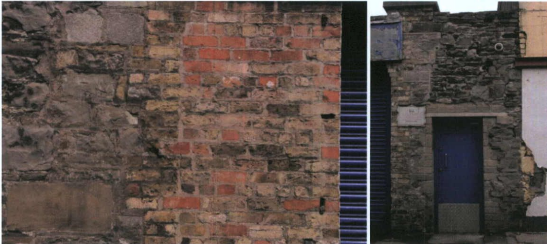
Fig.5.6.4: Later brick gate pier toothed-in to the Calp limestone masonry.
