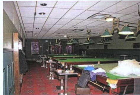
Plate 63: F-3 – View to north-west
