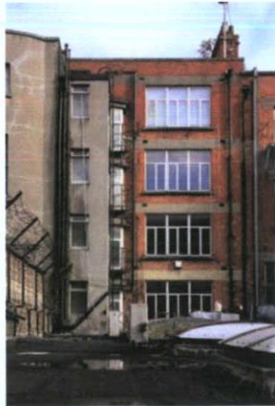
Plate 14: Rear (west) elevation
