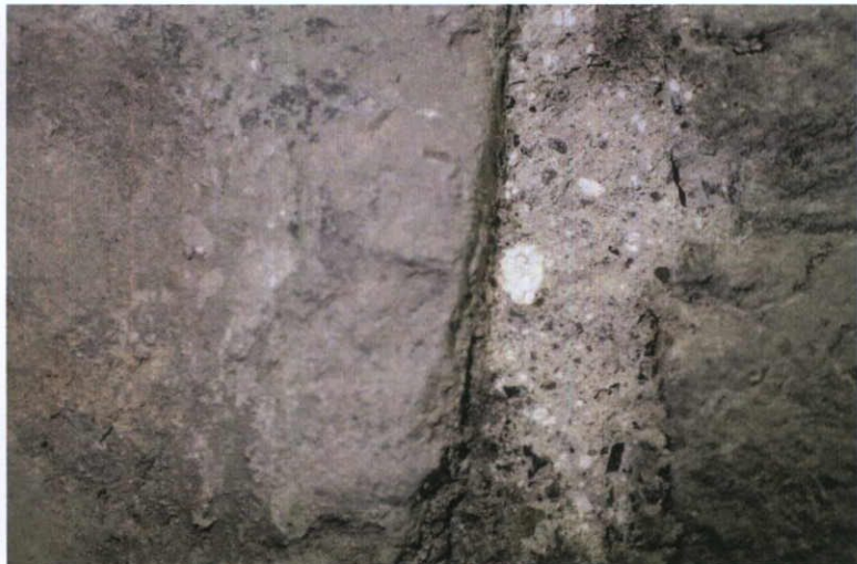
Fig.5.7.4: Detail of a mid-nineteenth century brick arch at basement level of No.60, with sharp limestone sand and coarse lime lumps in the bedding mortar (beneath the Portland Cement pointing).
