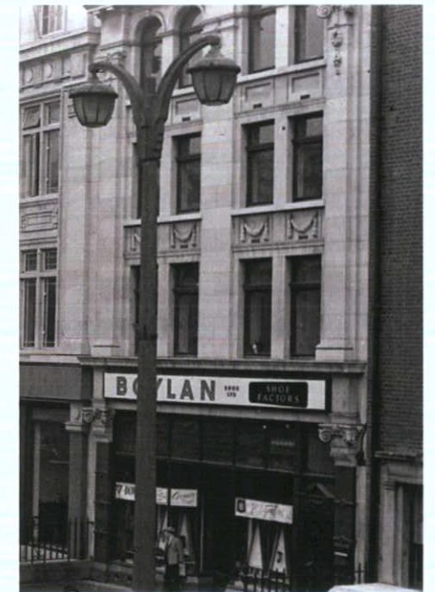
Figure 1: Façade c1960s showing original windows
